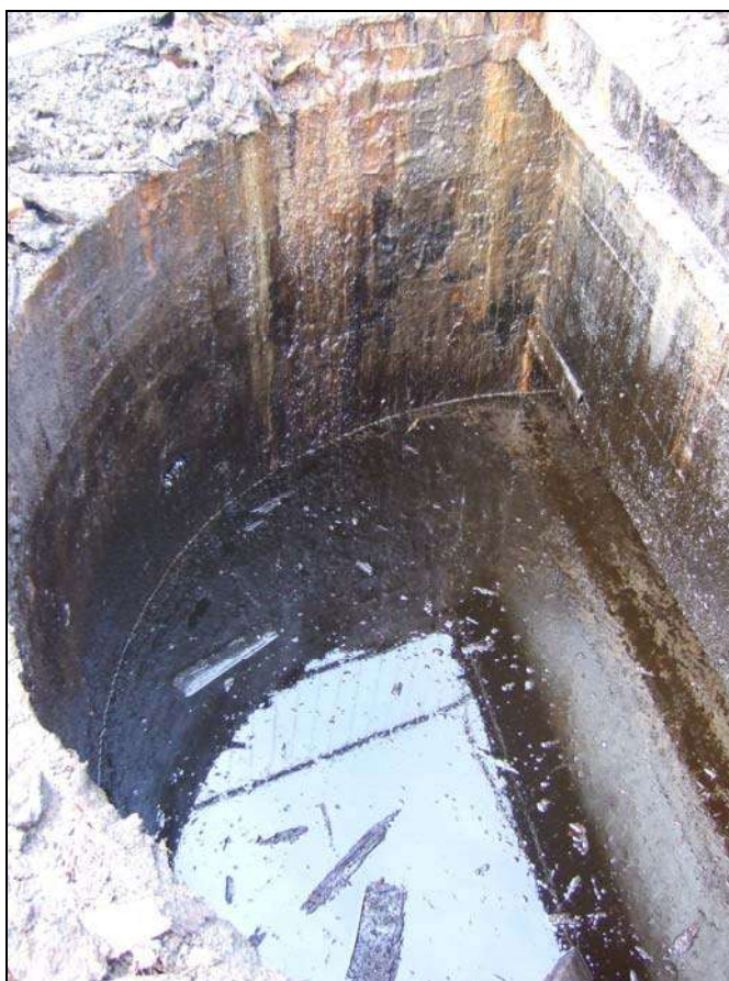
Plate 2 – Interior of Tar Tank
