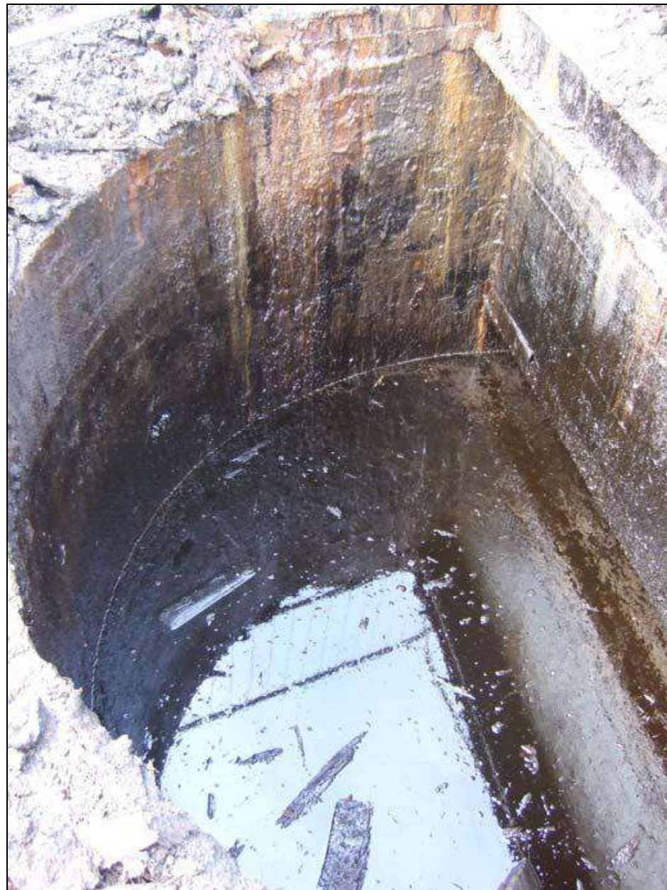
Plate 2 – Interior of Tar Tank
