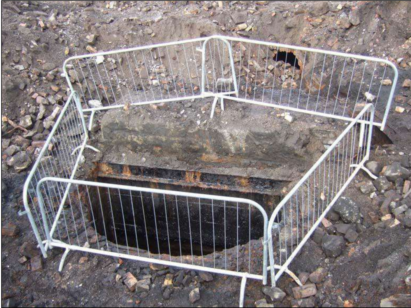
Plate 1 – Tar Tank beneath Unit D.
