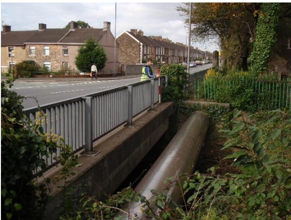
Figure 2-5 Upstream face of A48 bridge
