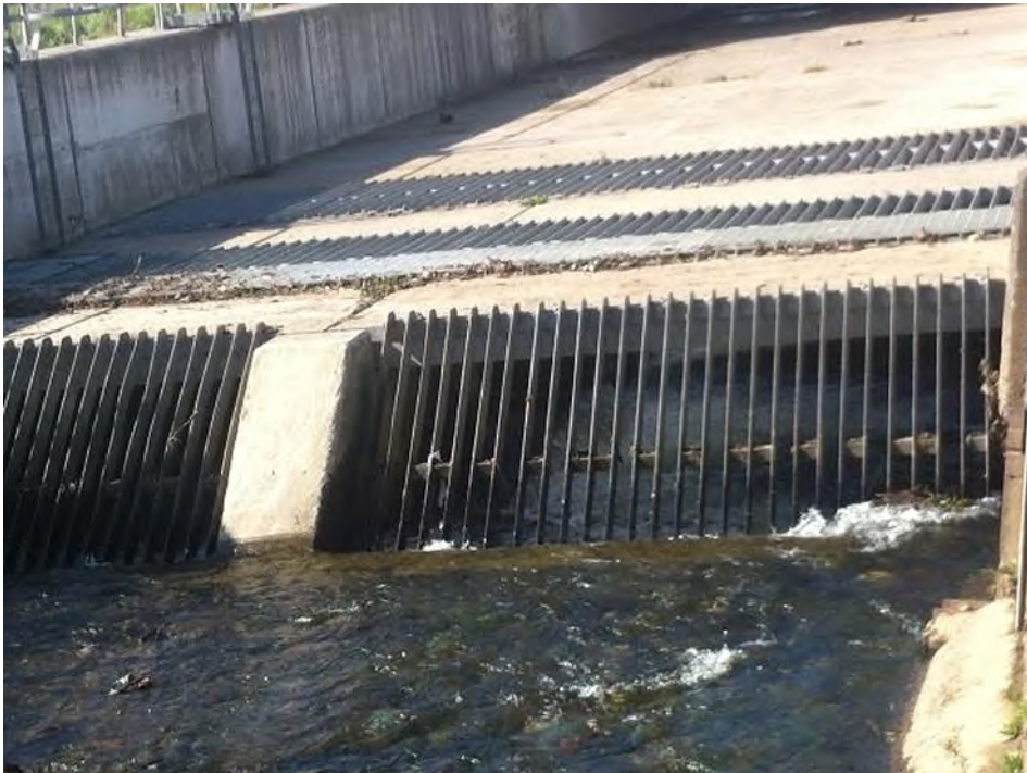
Figure 2-4: Culvert inlet and overflow upstream of PDR
