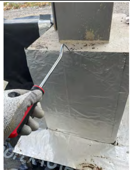
Pick and probe test to the Fosroc Proofex 3000MR.
