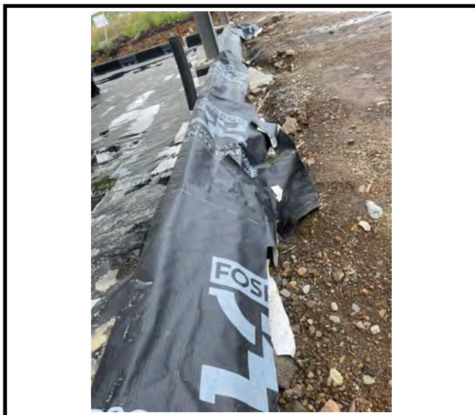
Installers have installed the Fosroc Proofex Total Gas Membrane tight to the perimeter walls.
