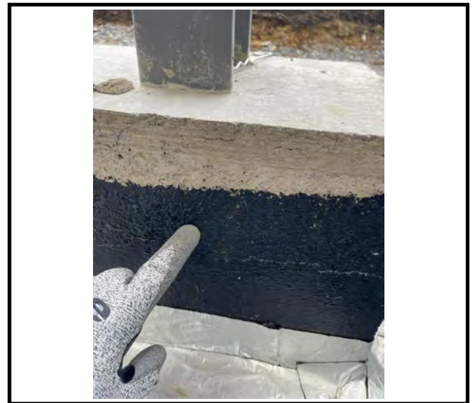
A photograph showing a primed column.
