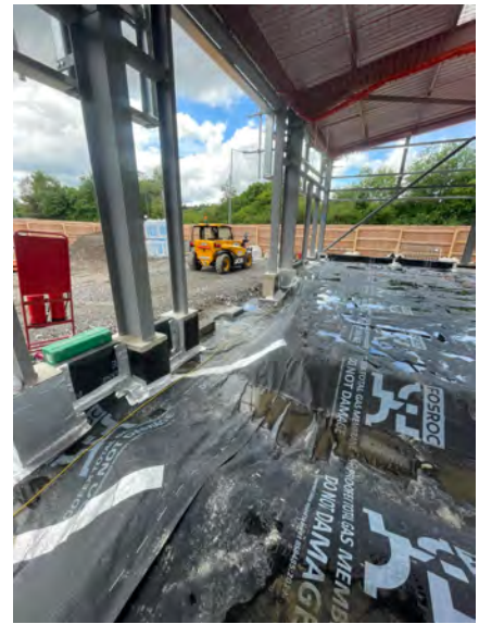
Overview of the area where the Fosroc Proofex Total Gas Membrane has been installed.
