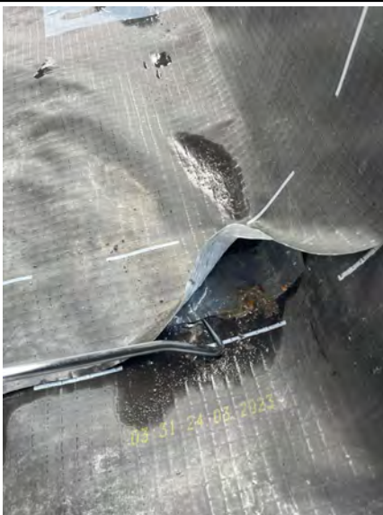
Pick and probe test on a taped lap joint.
