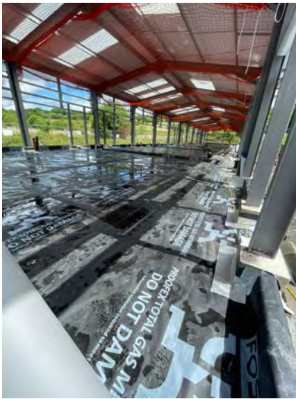
Overview of the area where the Fosroc Proofex Total Gas Membrane has been installed.
