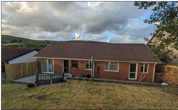
PHOTO REF A - REAR OF PROPERTY
