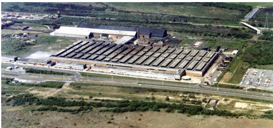
Figure 3: Photograph of the plant estimated from 1968.
