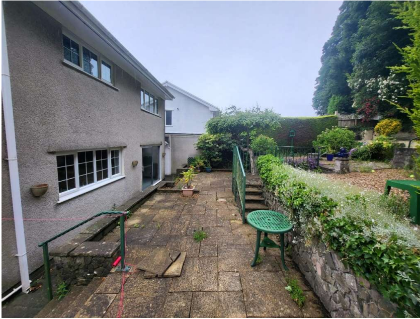
View of rear elevation and raised patio area. The new extension will be sited onto the existing hard surfaced areas
