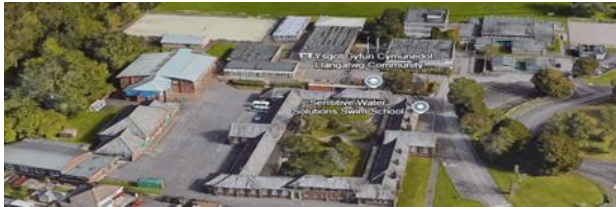
Fig.5.1 – Existing school demolished in Phase 2
