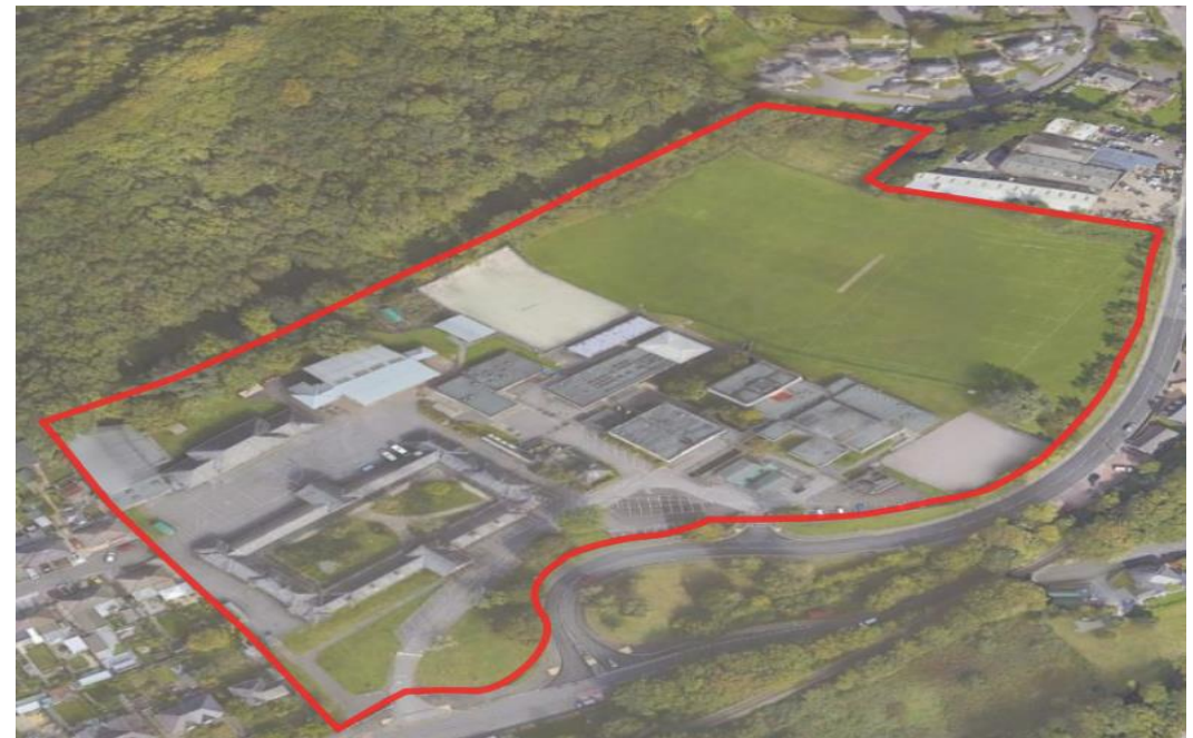
Fig.1.11 – Aerial View of Site
