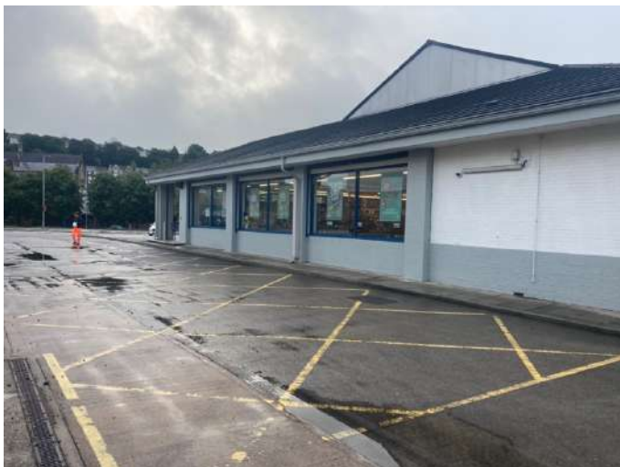
Photo 6: View eastwards along service road giving access to rear of both store buildings.
