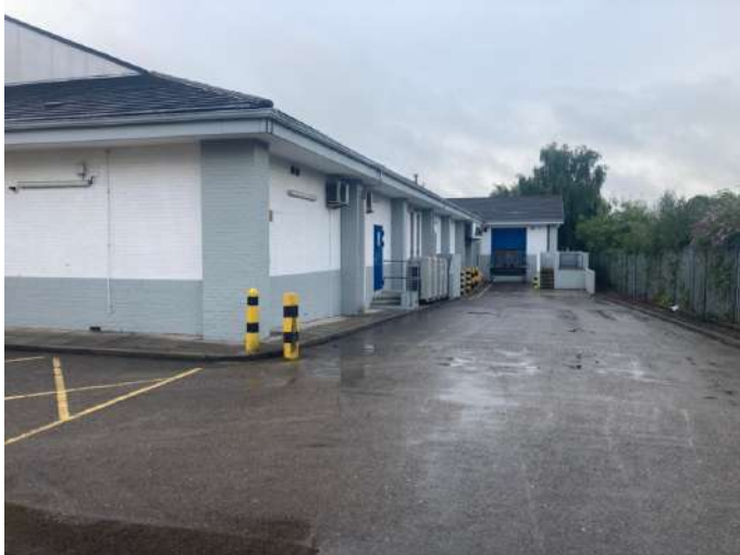
Photo 7: Lidl delivery area at rear of store.
