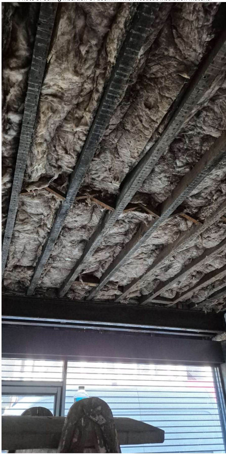
Photo 5: Ceiling Insertion Of 100mm Thick Acoustic Insulation Material
