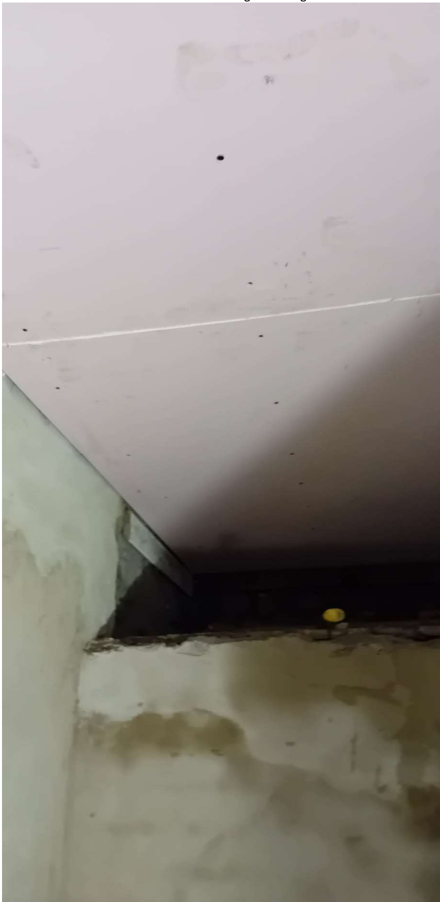
Photo 10: Plastering Of Ceiling
