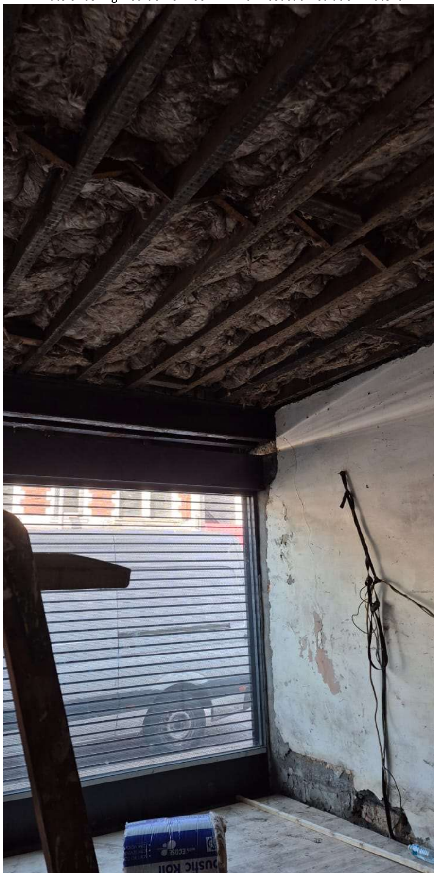
Photo 6: Ceiling Insertion Of 100mm Thick Acoustic Insulation Material
