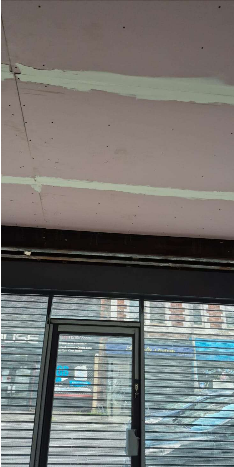
Photo 9: Plaster-Boarding Of Ceiling
