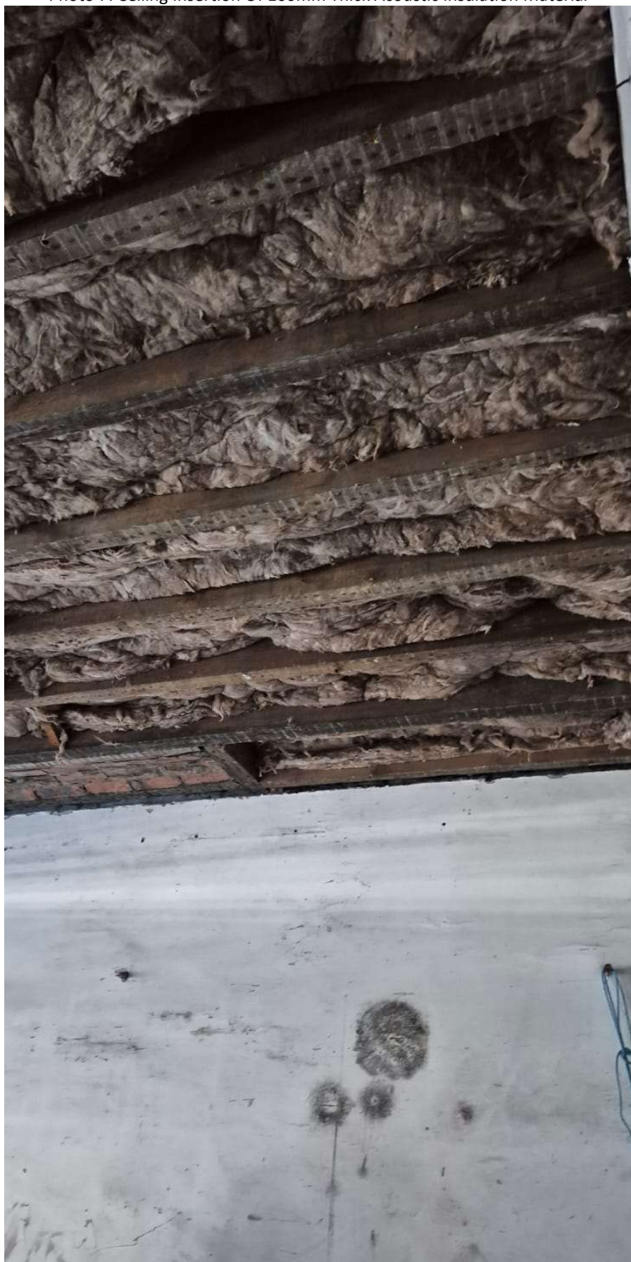
Photo 7: Ceiling Insertion Of 100mm Thick Acoustic Insulation Material
