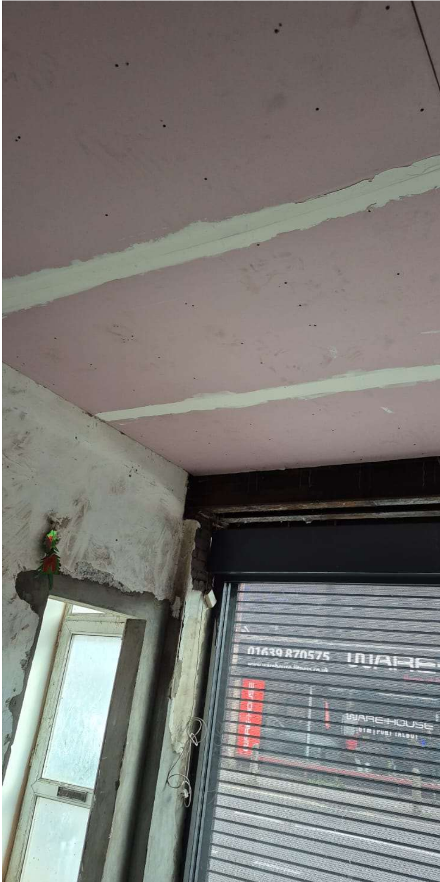
Photo 8: Plaster-Boarding Of Ceiling
