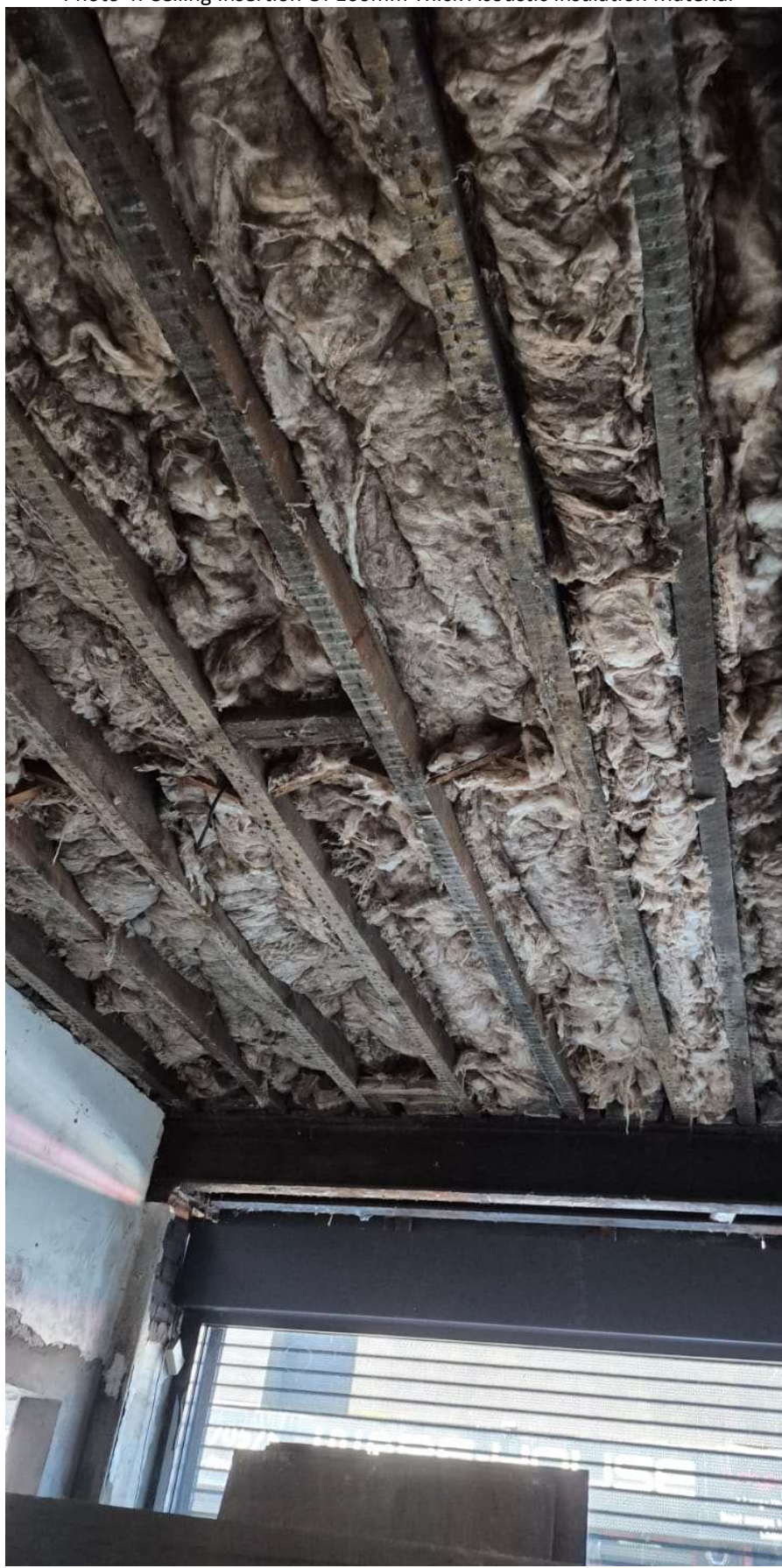
Photo 4: Ceiling Insertion Of 100mm Thick Acoustic Insulation Material
