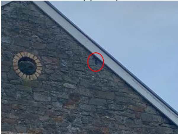
Photo 26: Permanently Open Window and Further Cracks in Stone Masonry (Circled) – B1
