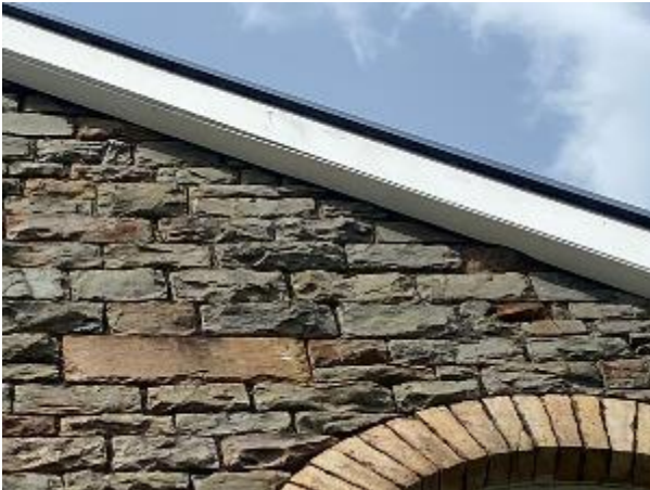
Photo 22: Gaps under Barge Board on Southern Front – B1
