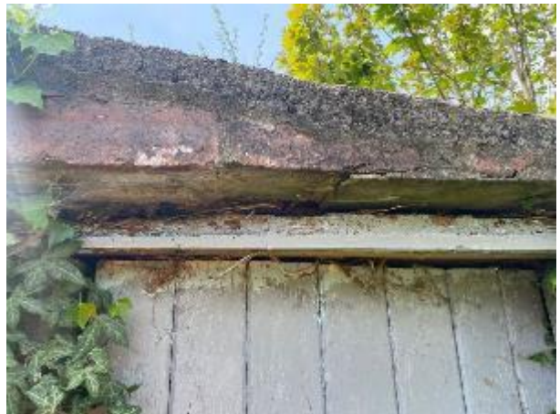
Photo 34: Gap in Wooden Frame – B3
