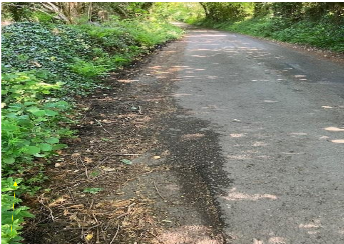
Repairs carried out on top of existing tarmac
