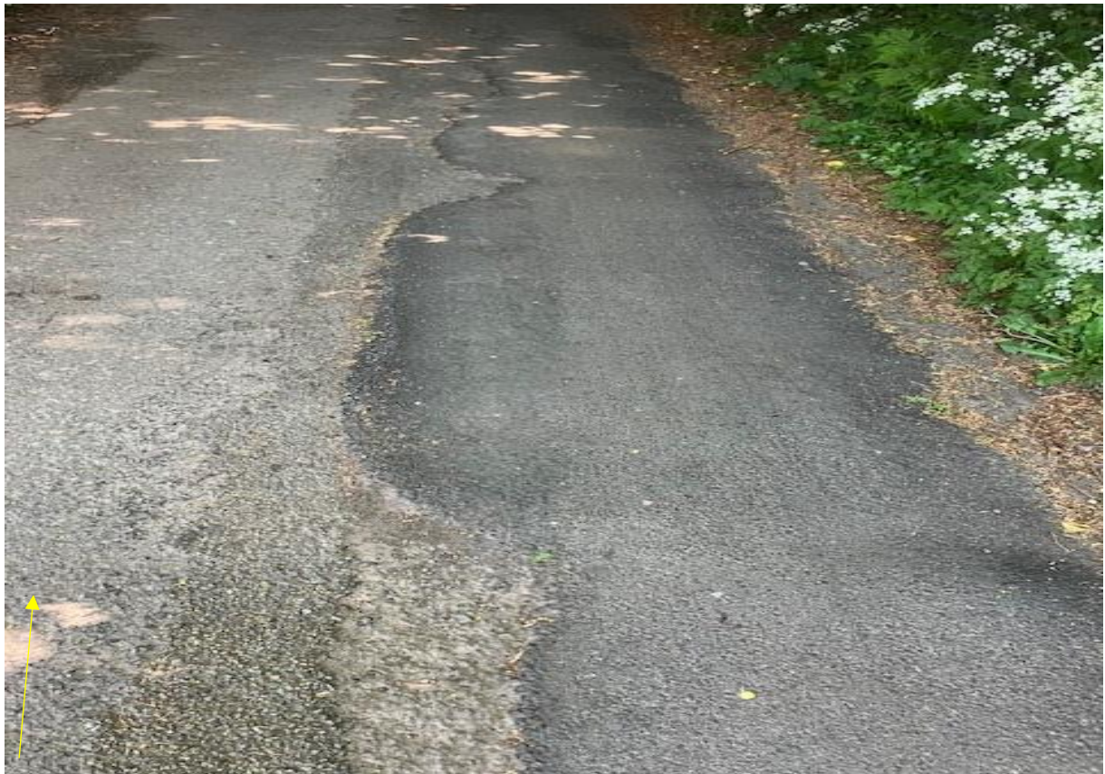
Repairs carried out on top of existing tarmac
