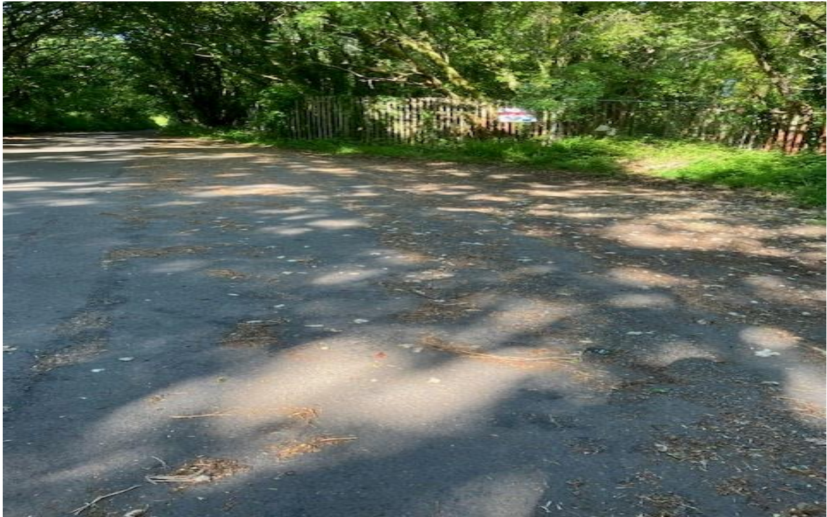
Secondary Entrance to Gelli Bwch Farm on the unclassified highway on the western side near to Llandarcy village dropping down to Prettyman Drive Junction Llandarcy
