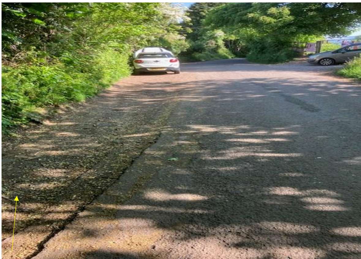
Rutts where vehicles have been parking minimum Rd width 4.6
