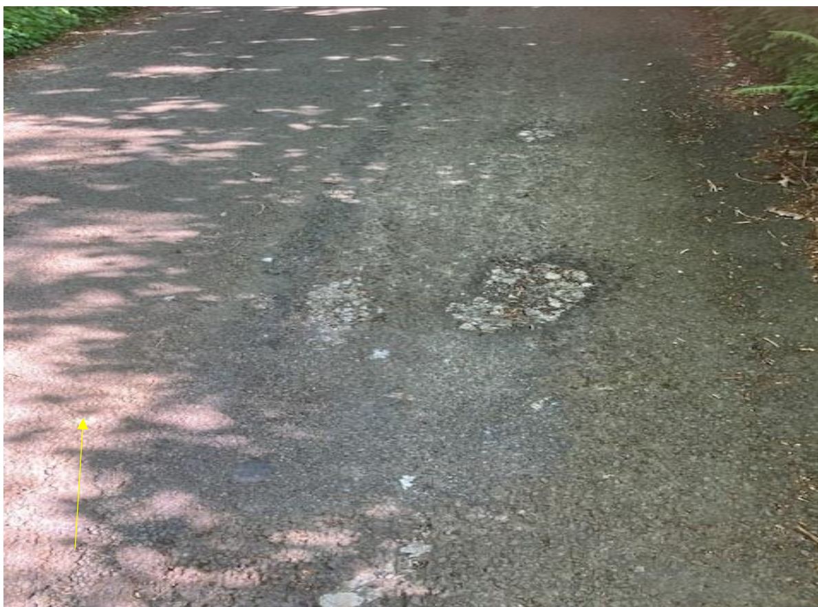
Various repairs have been carried out on top of existing tarmac
