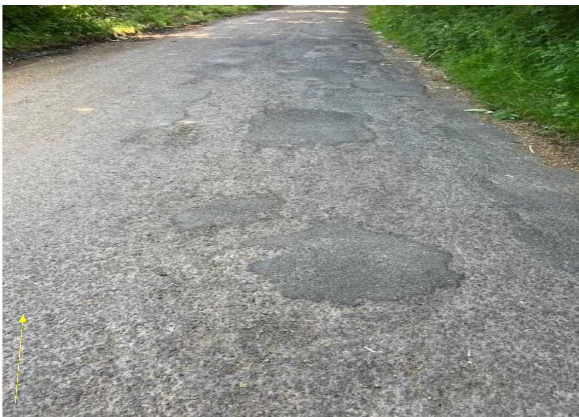
Rutts where vehicles have been parking minimum Rd width 4.6
