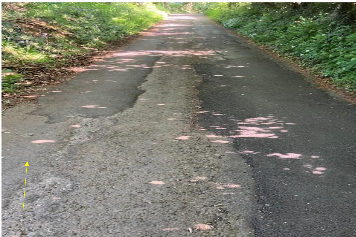
Various repairs have been carried out on top of existing tarmac
