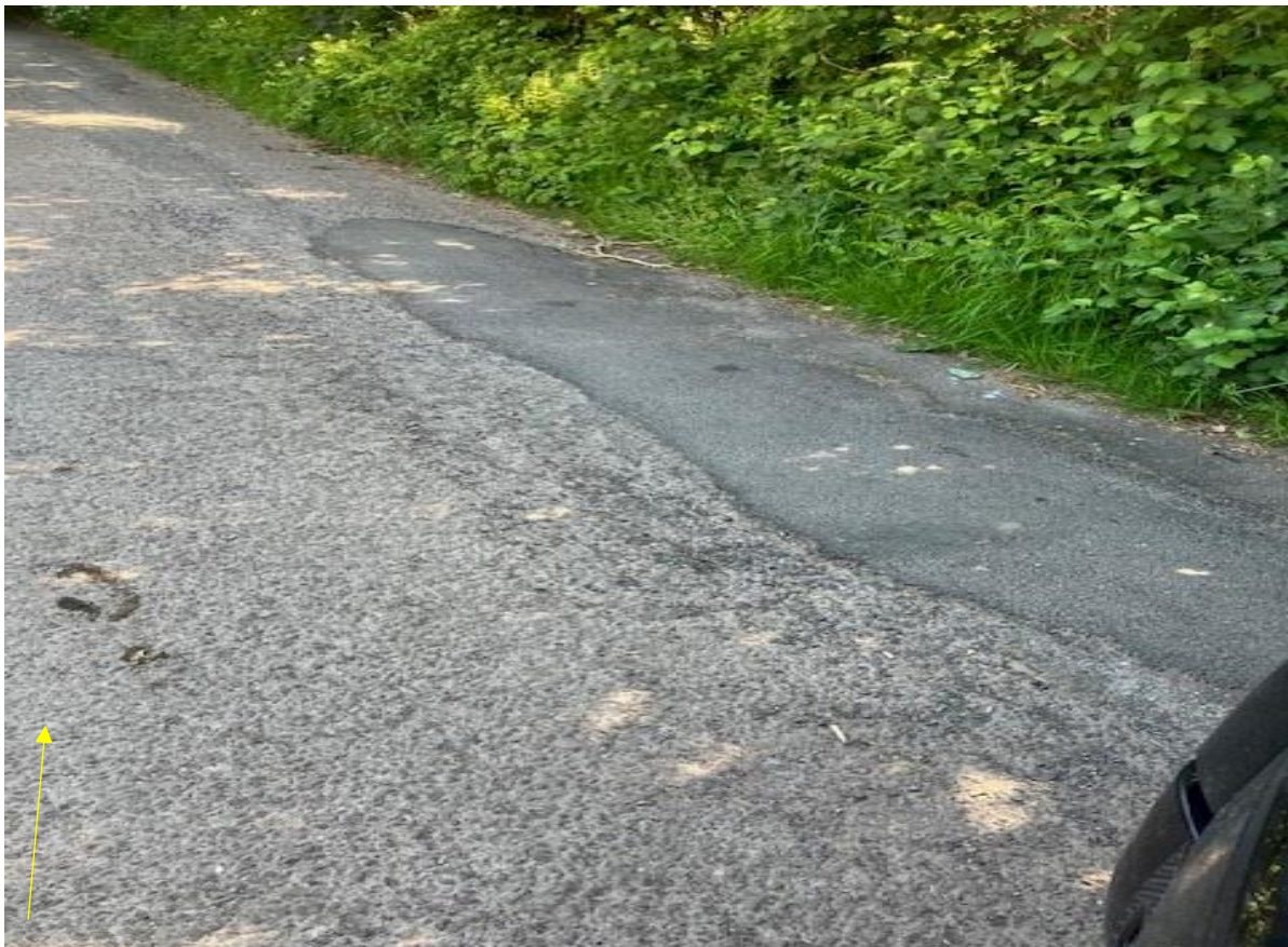
Repairs carried out on top of existing tarmac
