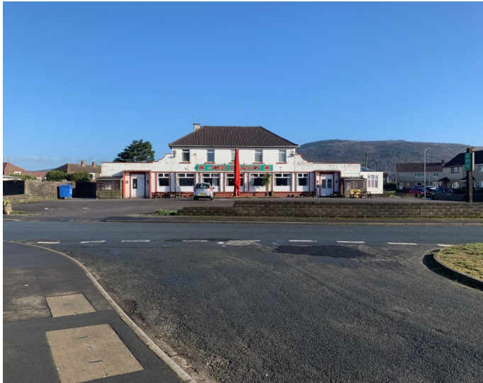
View of Red Dragon from Moorland Road.
