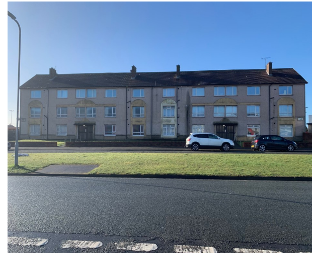
Dilapidated properties along Moorland Road.
