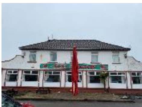
Photo 3. Southern elevation of main building section.
