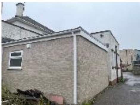
Photo 1. View from northwest corner of site of western elevation of building.
