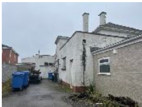
Photo 2. Northern elevation of building with series of flat roofed extensions off main building.
