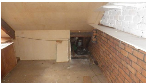
Access into eaves from Loft room A
