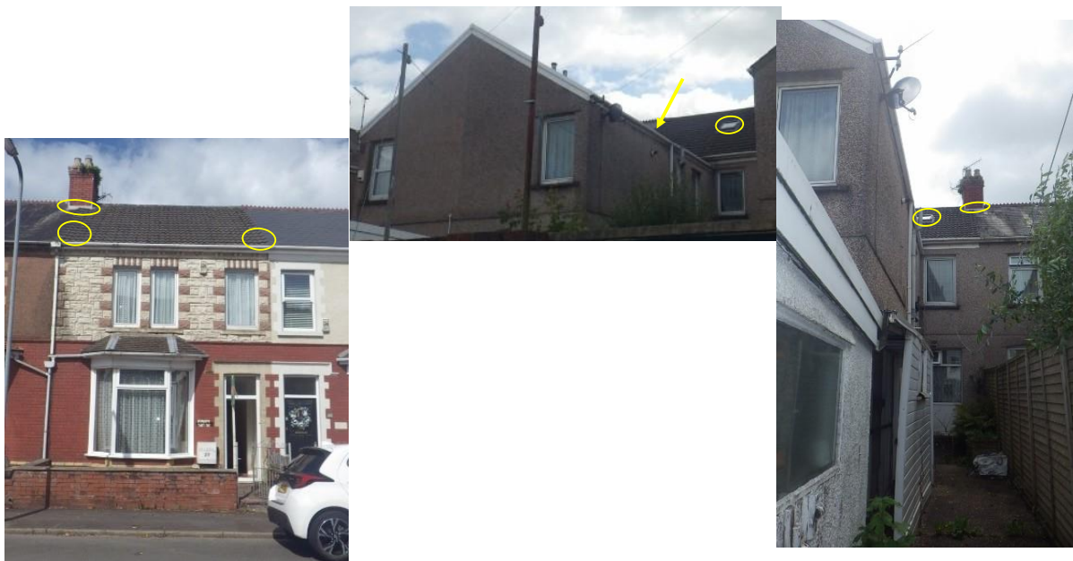
Potential crevice roost points via gaps under roof tiles, under chimney lead, and at the top and bottom of the rear roof valley
