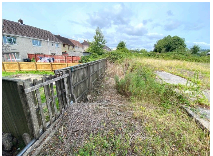
Eastern rear garden boundary fence of Heol Y Glo, viewing north
