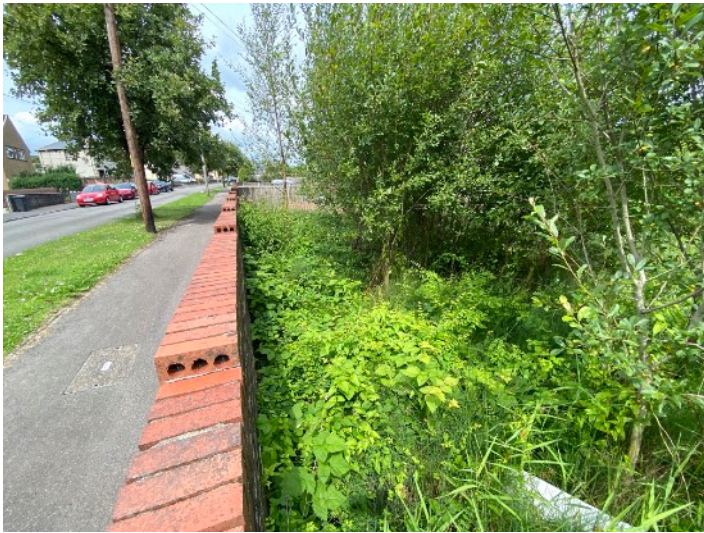
Low growing Bramble and Snowberry scrub to the east of the western boundary wall, viewing north
