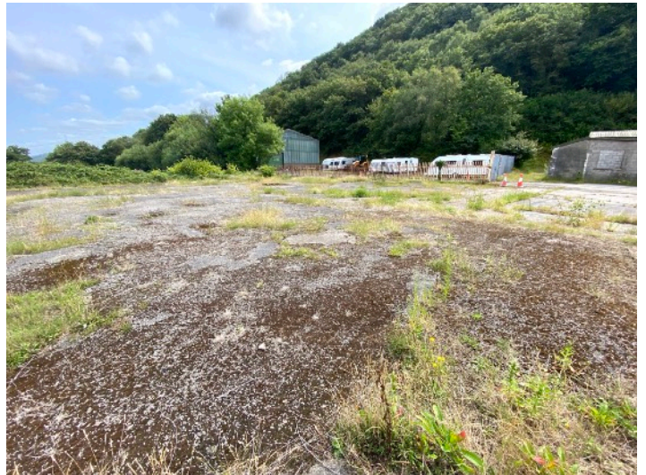
View south east with colonising vegetation growing over concrete hardstanding
