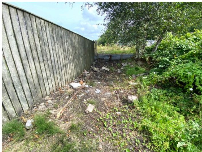
Bare earth area at south east corner of garden fence of 24 Heol Y Glo, viewing east
