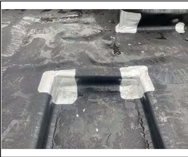
Additional sealed corners using gas resistant self adhesive membrane.
