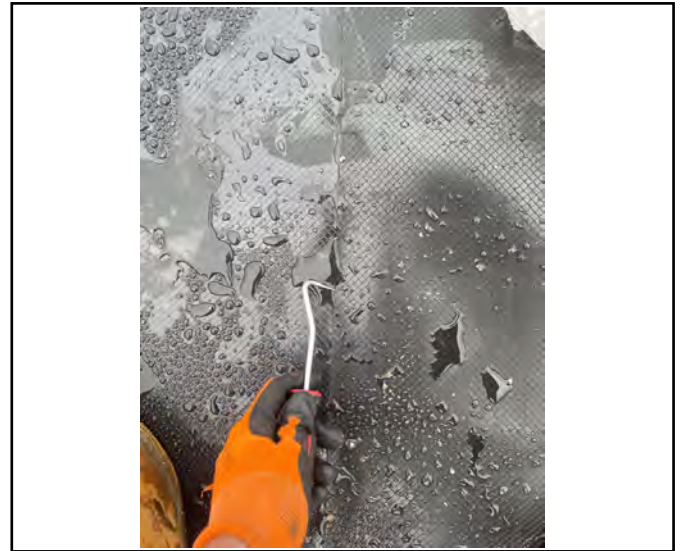
Additional pick and probe test carried out to welded lap.
