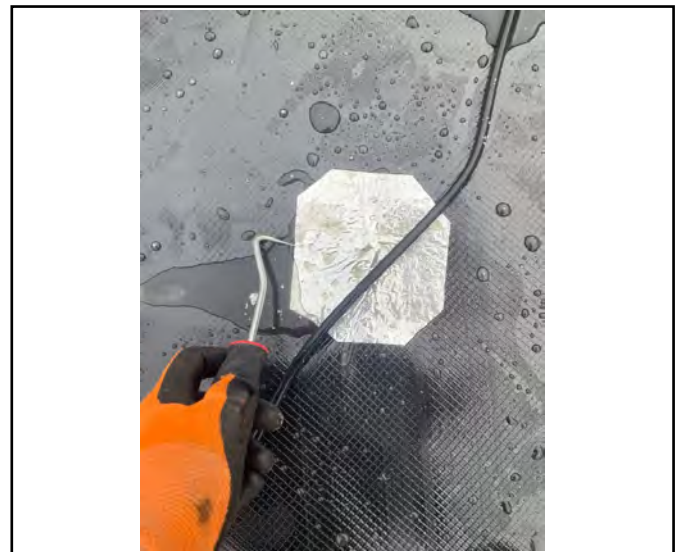
Pick and probe test carried out to patch repair.
