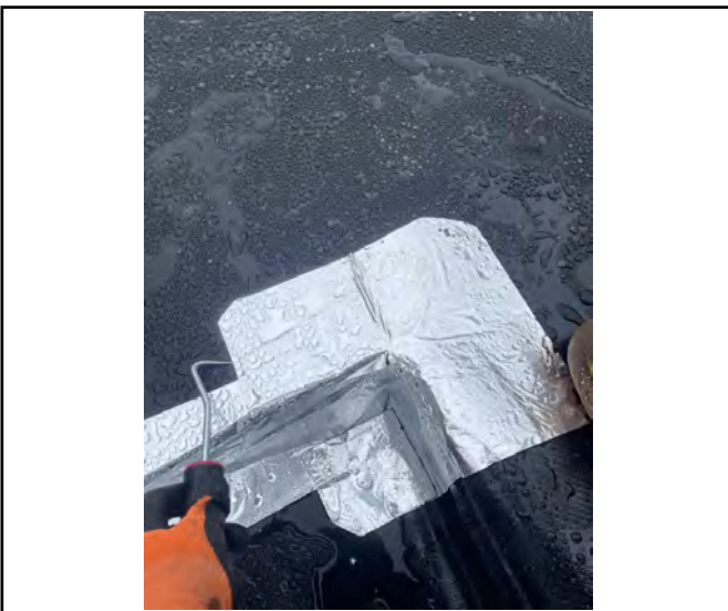
Pick and probe test carried out to sealed corner detail.
