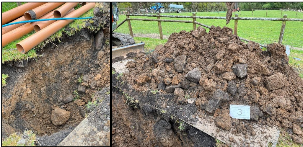
Insert 2 - View of ground conditions and arisings from TP203. Note Made Ground in upper portion.
