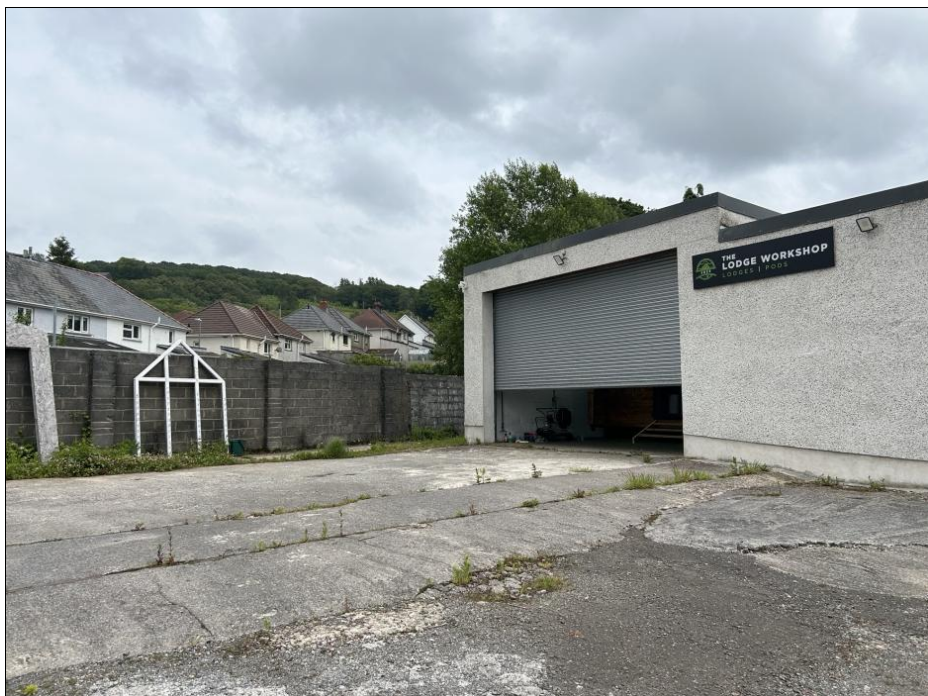
Photograph 3 – View of Side Elevation of Existing Building
