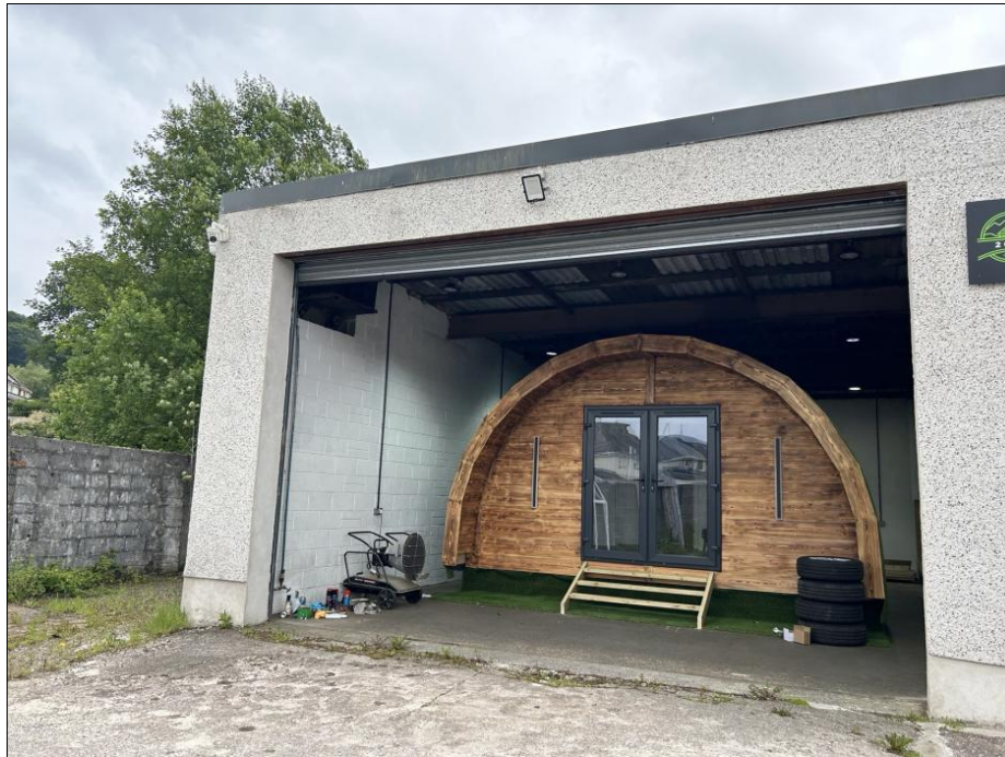
Photograph 4 – View of the Interior of the Western Portion of Building
