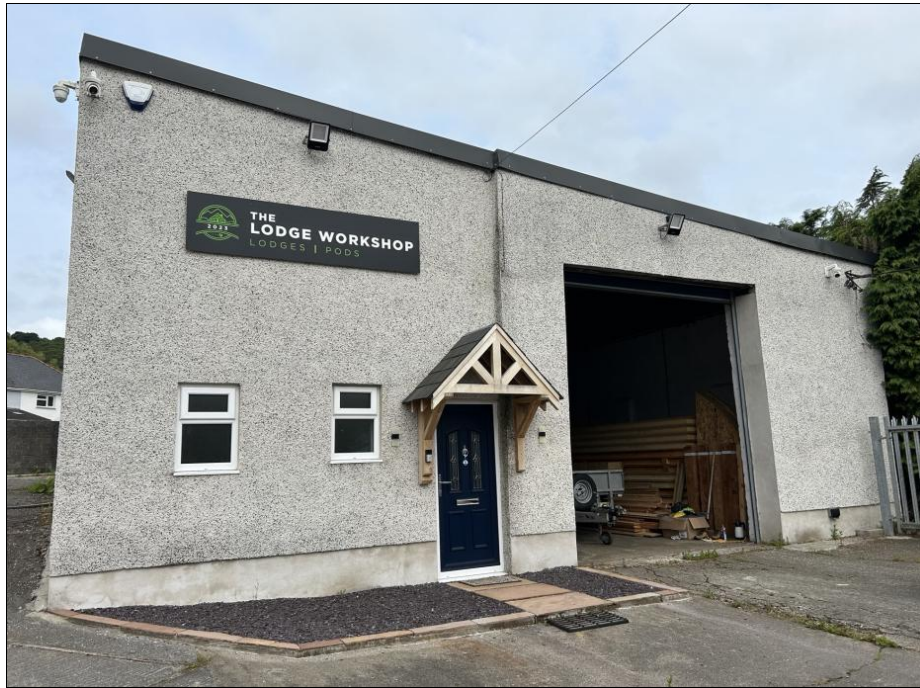
Photograph 1 – View of Front Elevation of Existing Building
