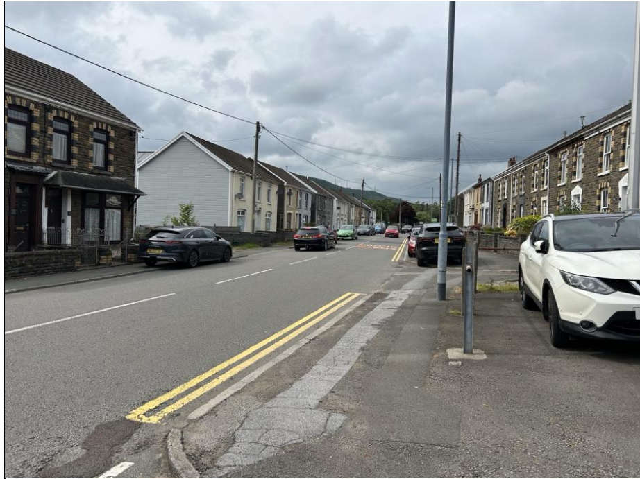
Photograph 13– Visibility Splay from the Site Looking North
