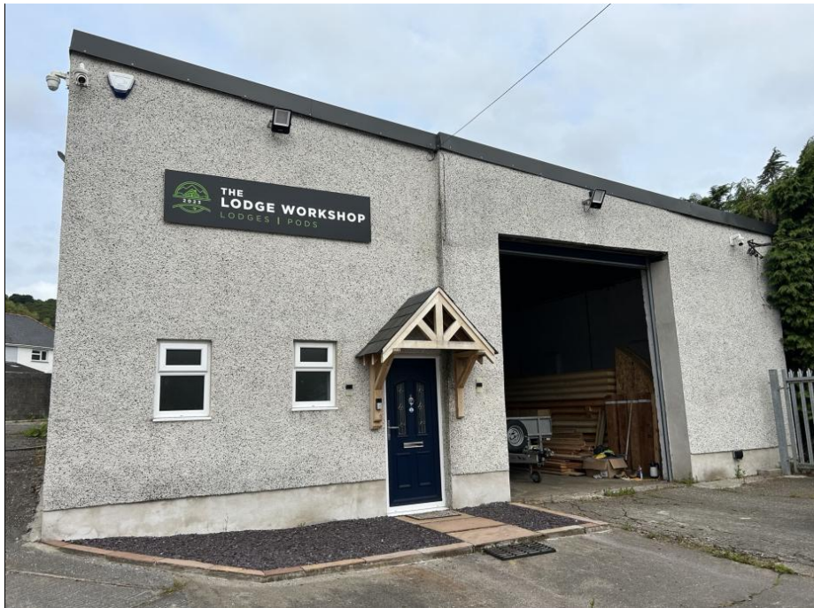
Photograph 1 – View of Front Elevation of Existing Building
