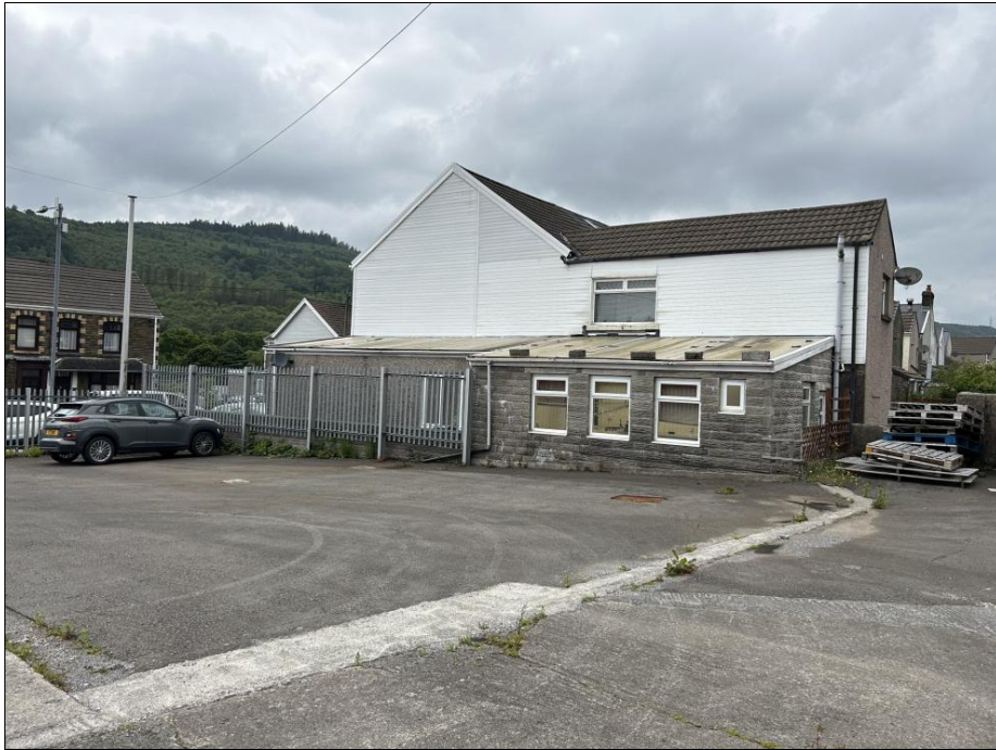
Photograph 9 – View of Northern Boundary with No. 43 Main Road
