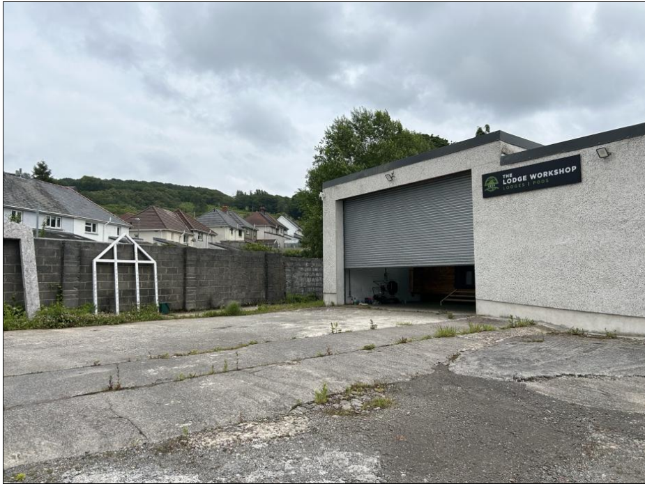
Photograph 3 – View of Side Elevation of Existing Building
