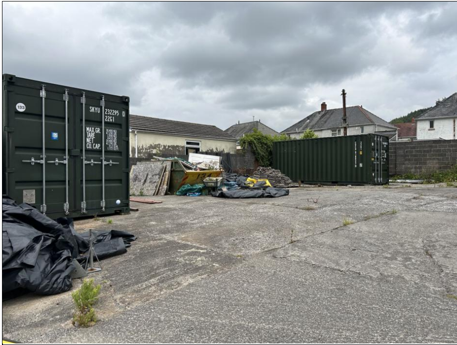
Photograph 7 – View of Northern Portion of the Yard
