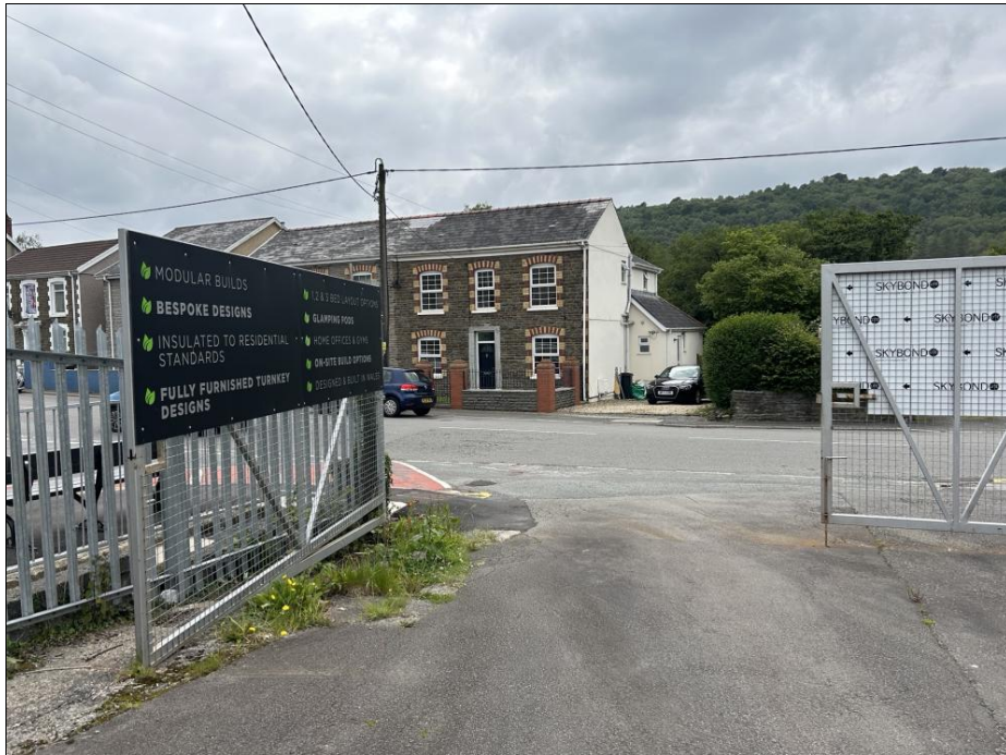
Photograph 11 – Existing Access to the Site
