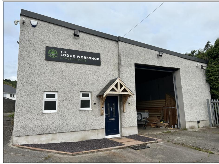
Photograph 1 – View of Front Elevation of Existing Building
