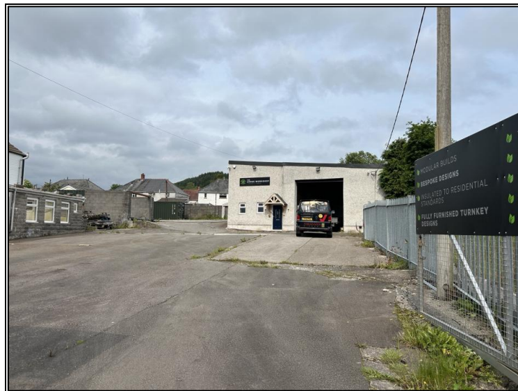
Photograph 2 – View of Front Elevation of Existing Building and Yard
