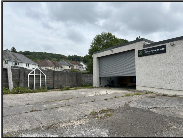
Photograph 3 – View of Side Elevation of Existing Building
