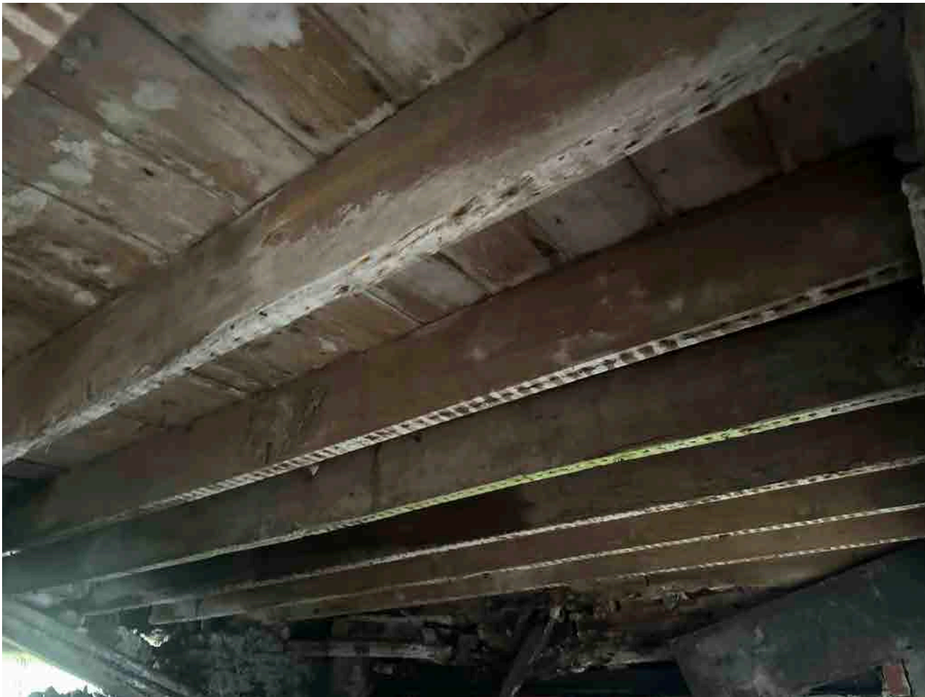
Underside of first floor joists.
