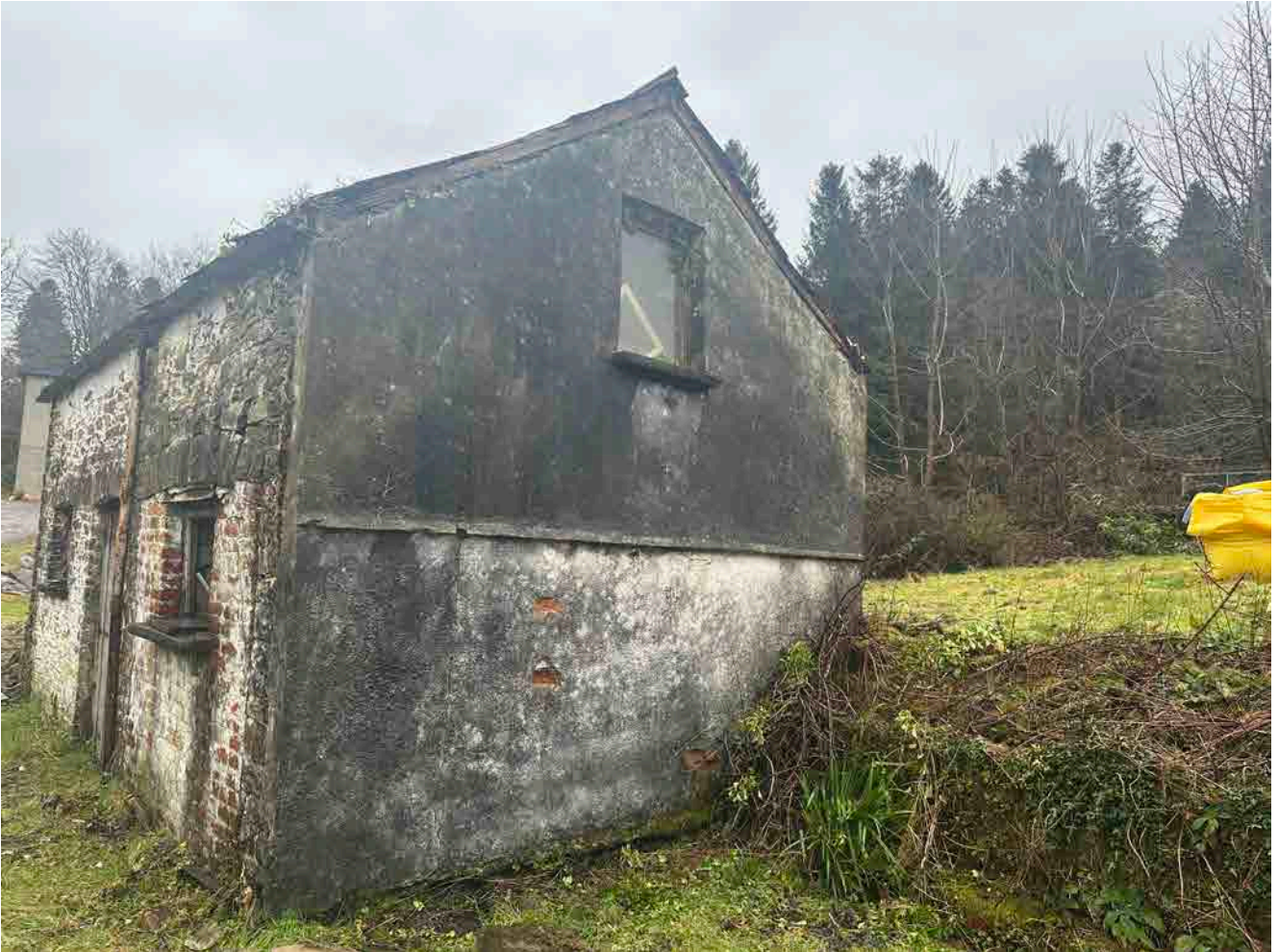
South West Gable Wall.
