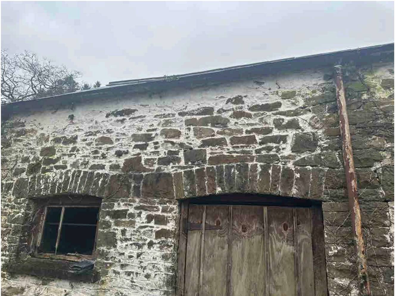
Stone masonry above opeinings in the northwestern face of the building.
