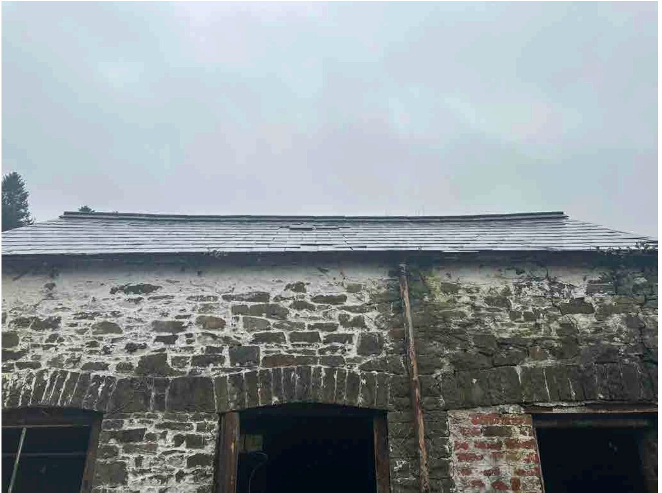
The roof appears to be mainly level with no sagging. Some tiles need to be replaced.
