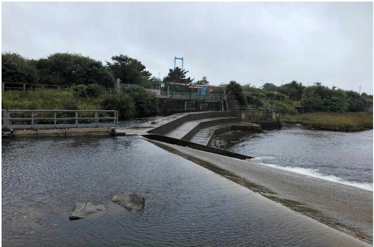
Photograph 5 – Weir to east of site.
