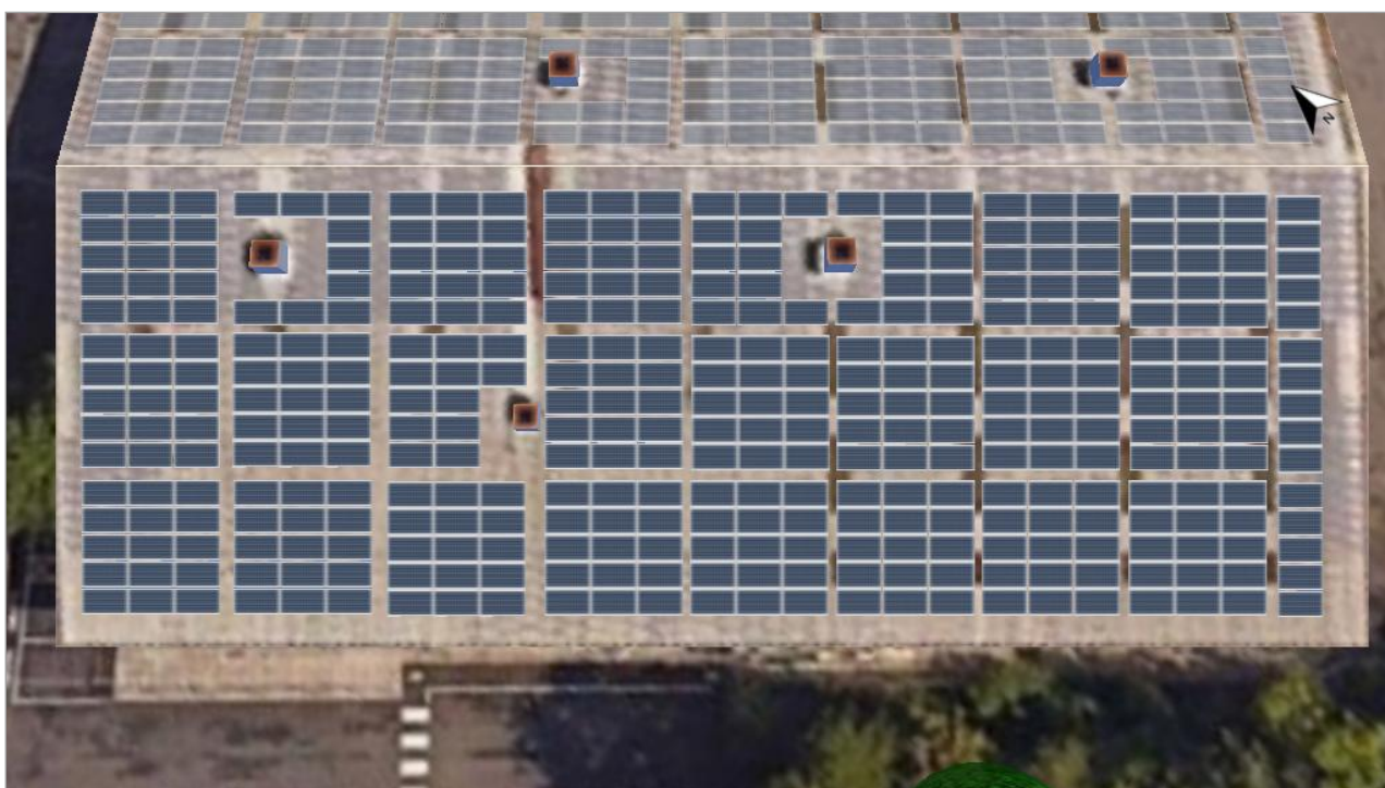
Figure: 2. Module Area - Building 01-Roof Area Southwest
