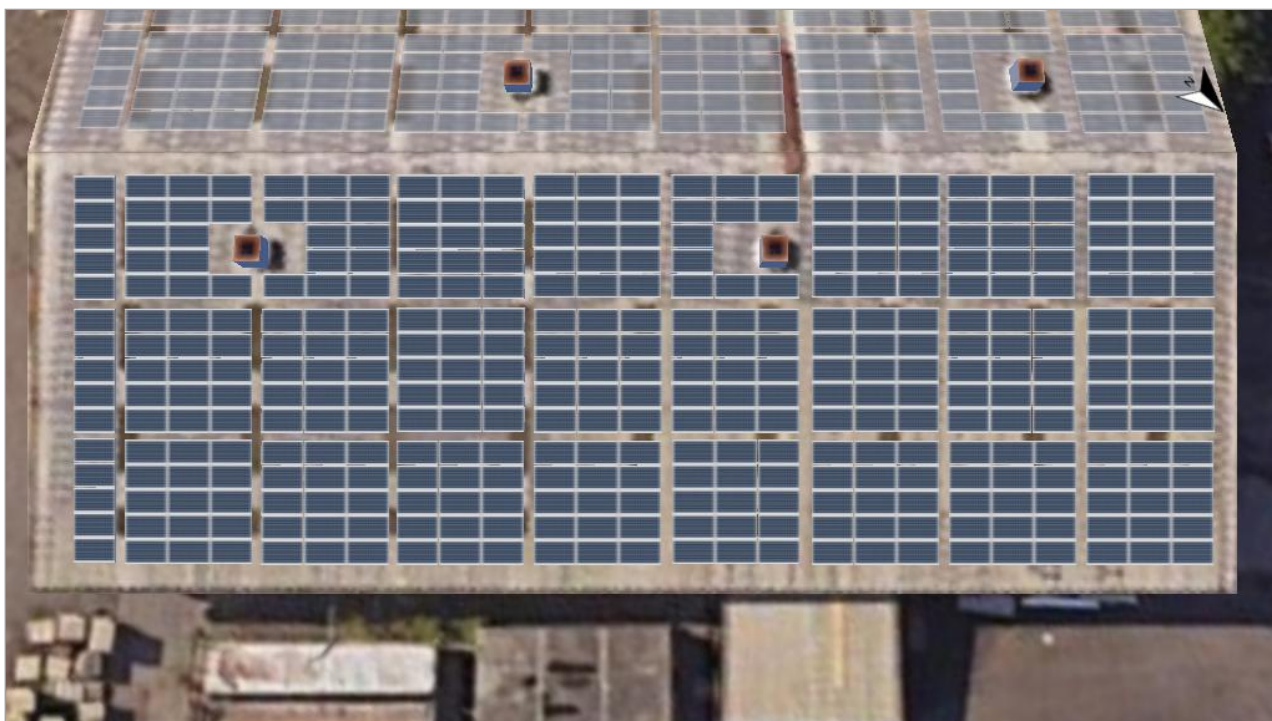
Figure: 1. Module Area - Building 01-Roof Area Northeast
