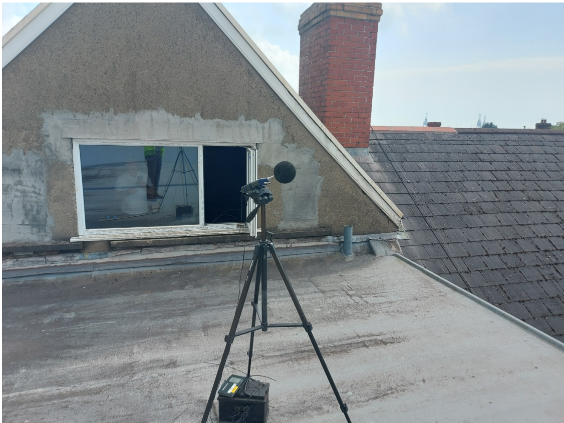
Picture 2: The ducting will terminate on the roof.
