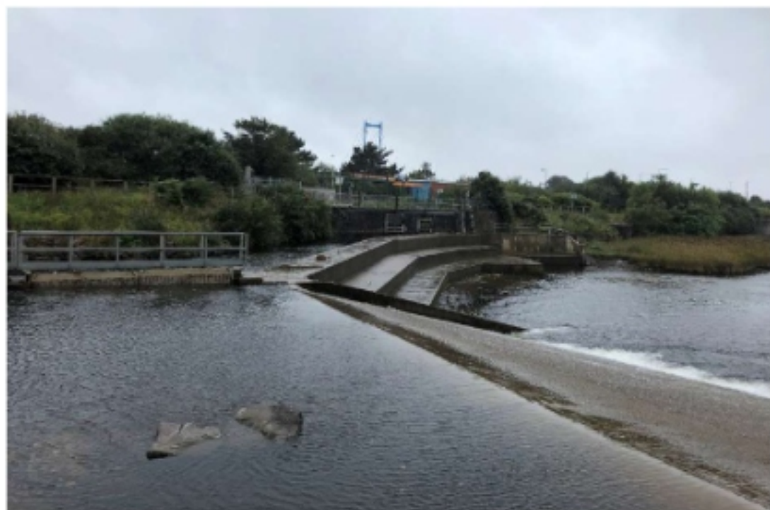
Photograph 5 – Weir to east of site.
