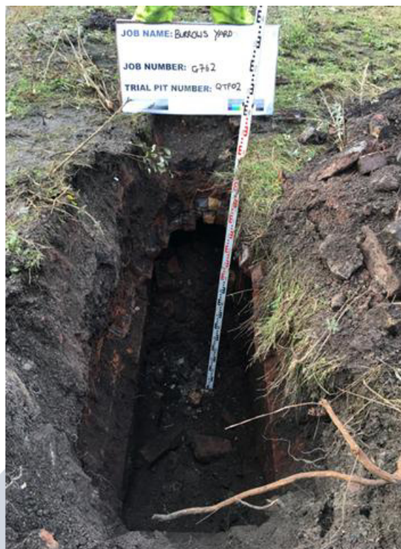
Possible Culvert identified in TP02 during the Quantum Investigation
