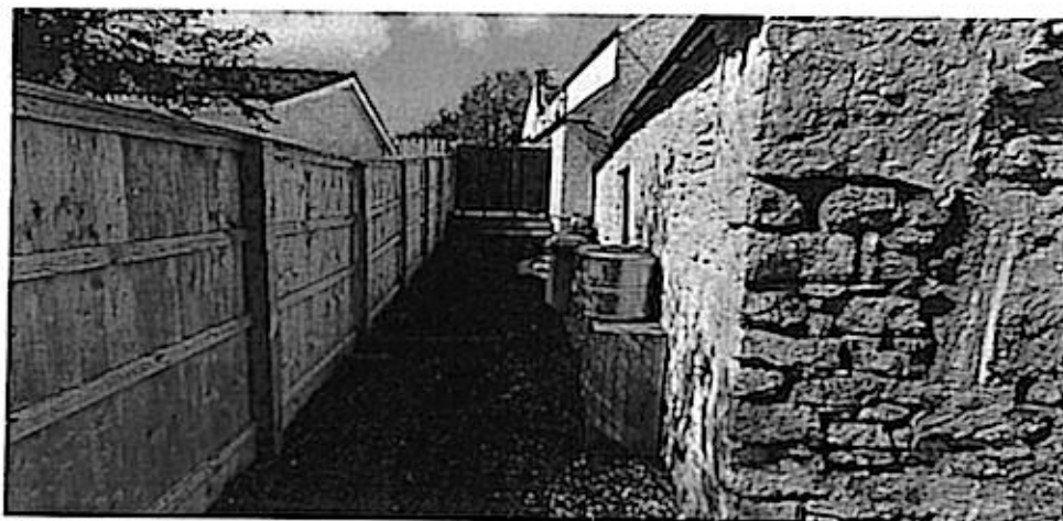
Photo from the northern corner of the site looking southwards.
