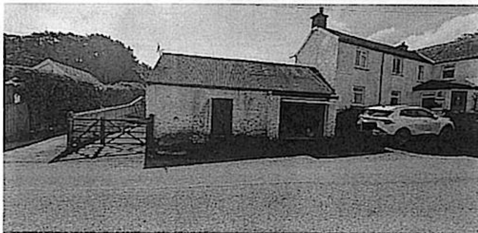
Site frontage from the west.
