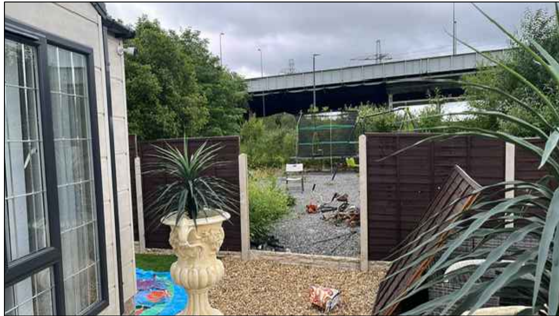
Access already in place for escape route
