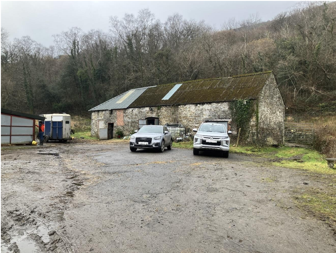
Figure 5, Photo showing stone building
