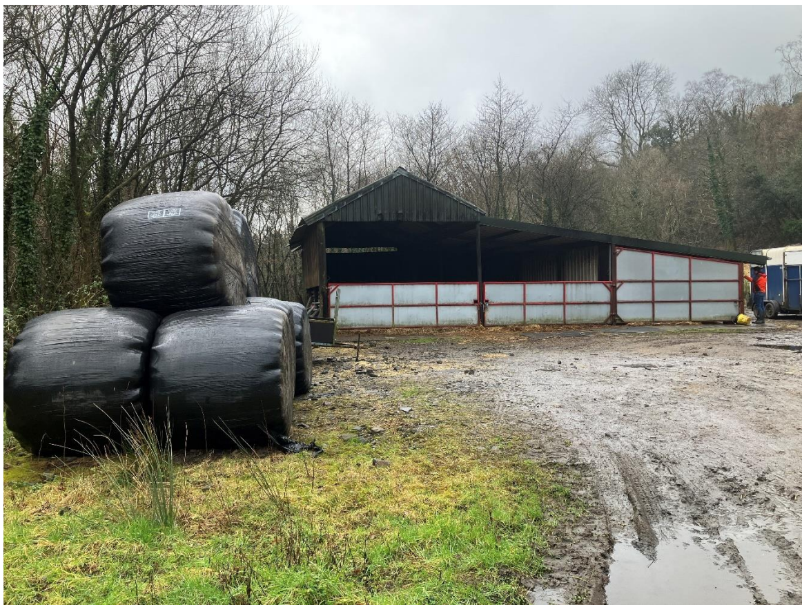
Figure 4, Photo showing metal stables facing north across yard
