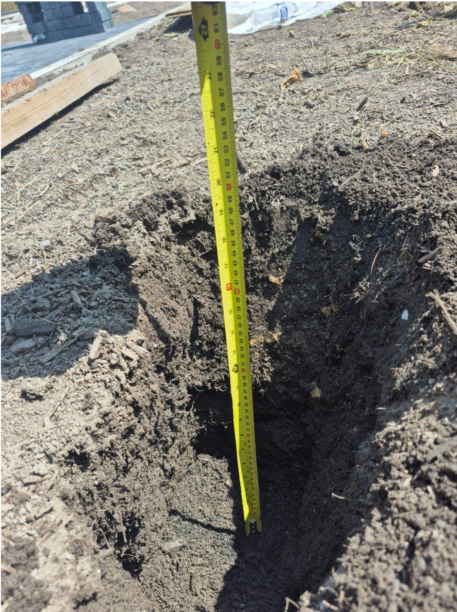
Plate 3: 450mm Thickness of Topsoil (Pit 2)
