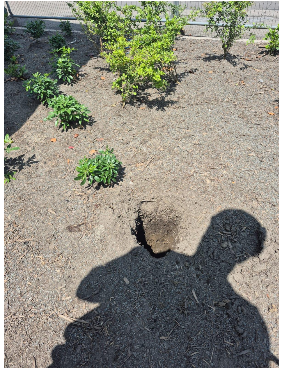
Plate 2: Inspection Hole Position (Pit 1)
