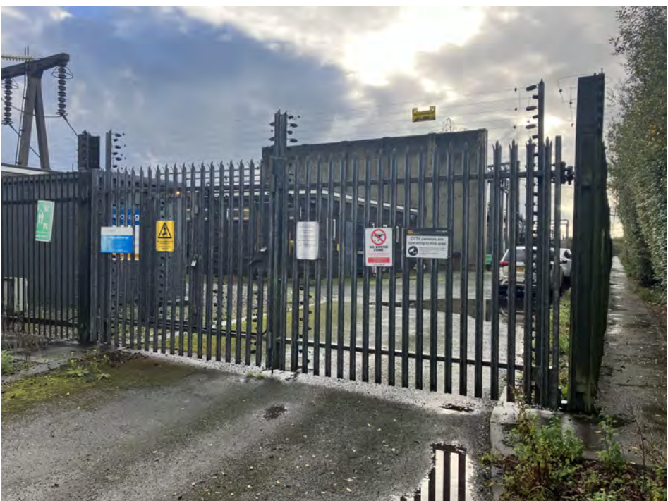
EXAMPLE IMAGE SHOWING STEEL ACCESS GATE WITH ELECTRIFIED WIRE OVERHEAD
