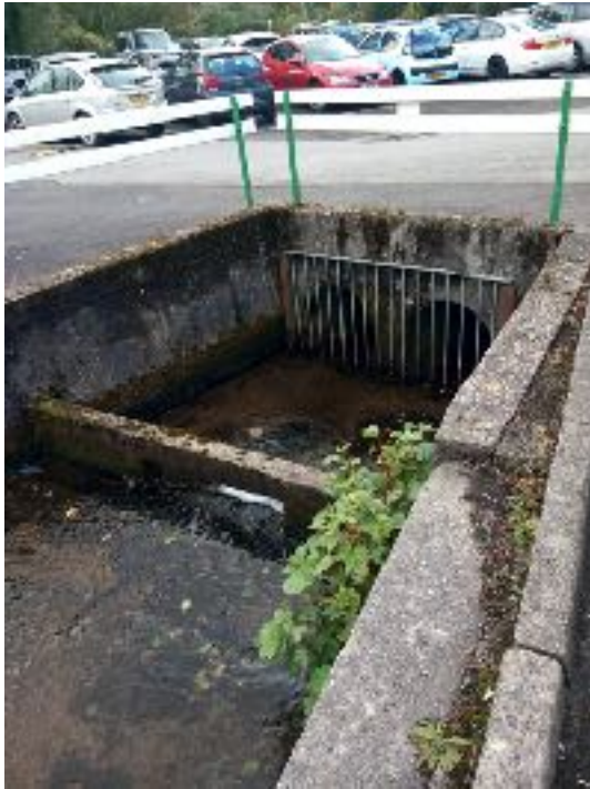
Photo 6 Grilled entrance to the culvert beneath the car park (Looking south west)
