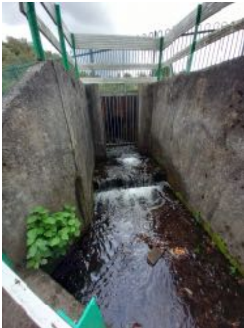
Photo 2 Grilled end of the culvert south of sports field (Looking east)
