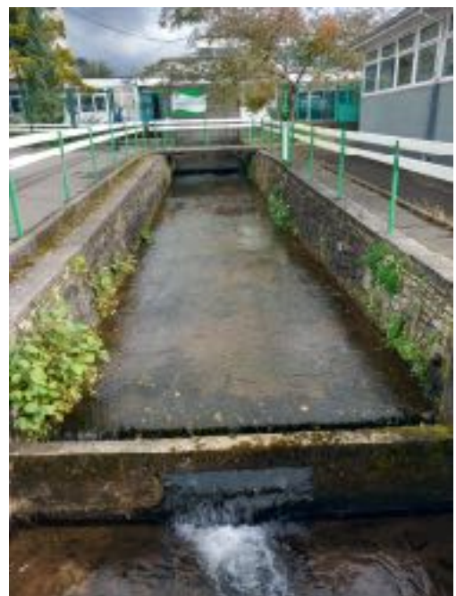
Photo 5 Channel flowing to the south in between Buildings 3 and 4 (Looking east)
