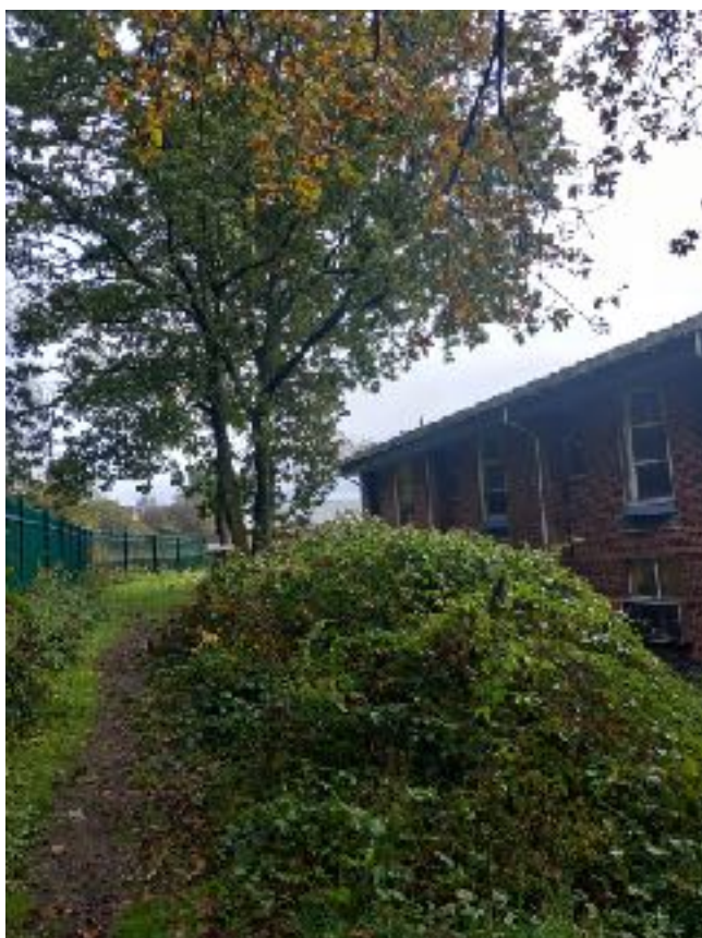
Photo 16 vegetation to the rear of Building 7 (Looking north)
