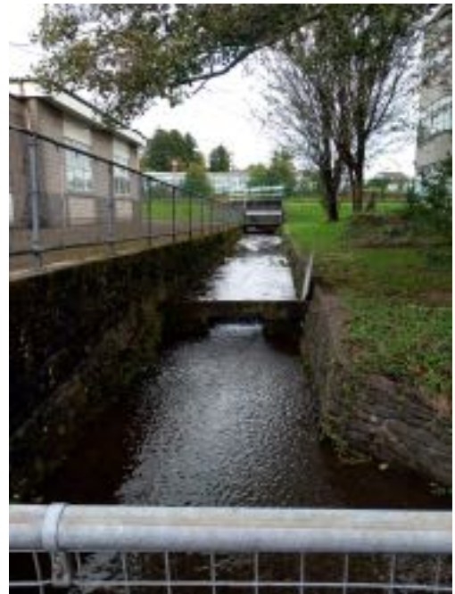
Photo 3 Canalised channel flowing south (Looking east)
