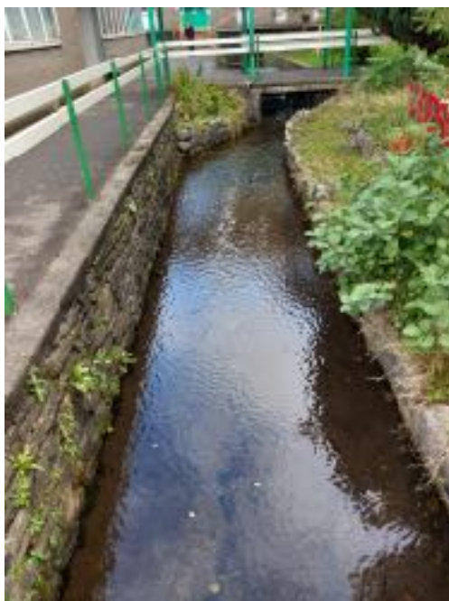
Photo 4 Channel flowing west (Looking north)
