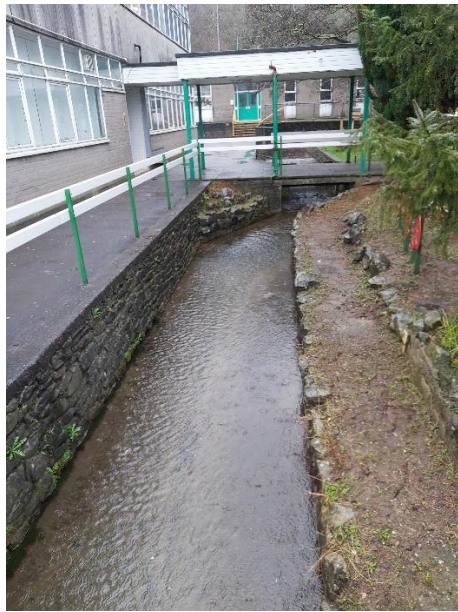
Fig. Appendix A1 Photo of culverted stream running through the existing school site
