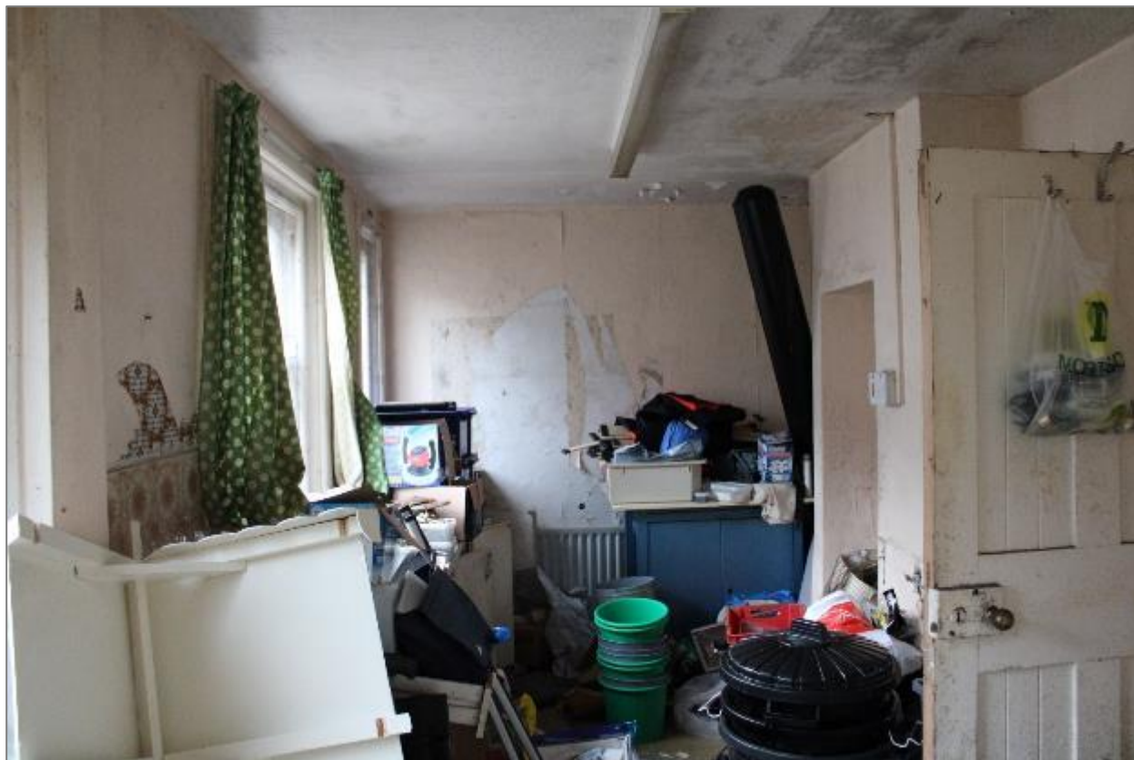
Photo 77: Kitchen, with former fireplace to the right. Facing southeast.
