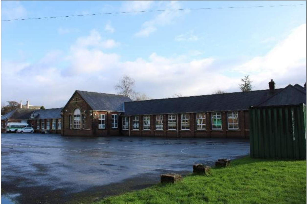
Photo 9: Northwest facing façade. Facing east.
