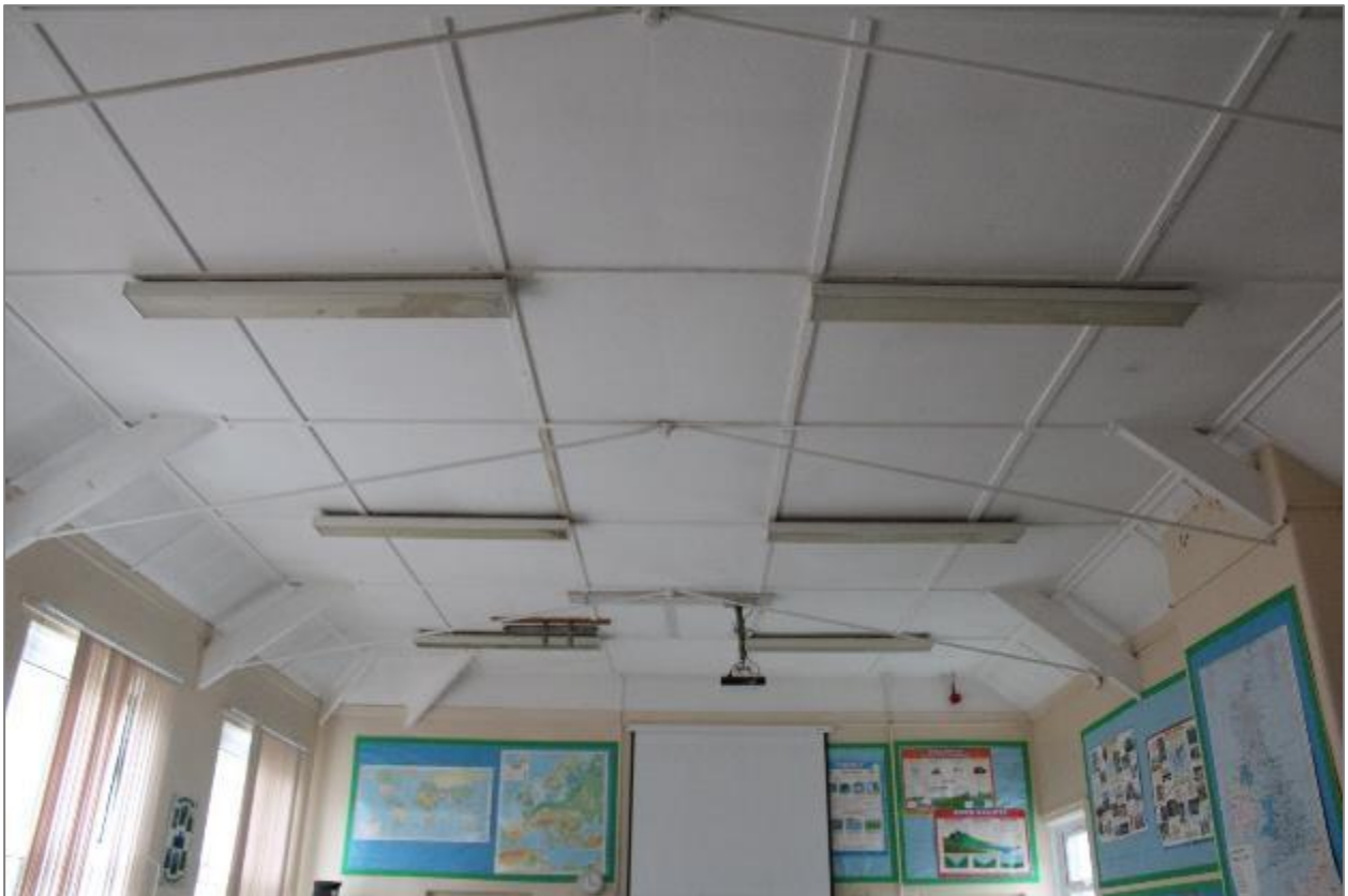
Photo 47: Ceiling with visible joists and bracing in corner classroom.
