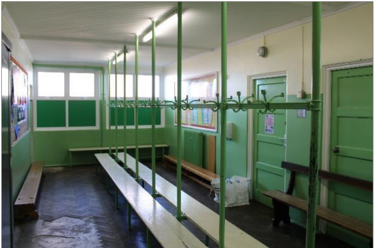
Photo 94: Interior of the gymnasium changing room, facing east.
