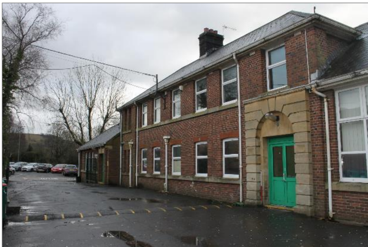
Photo 5: Northeast facing façade. Facing southeast. 1 x 1m scale.
