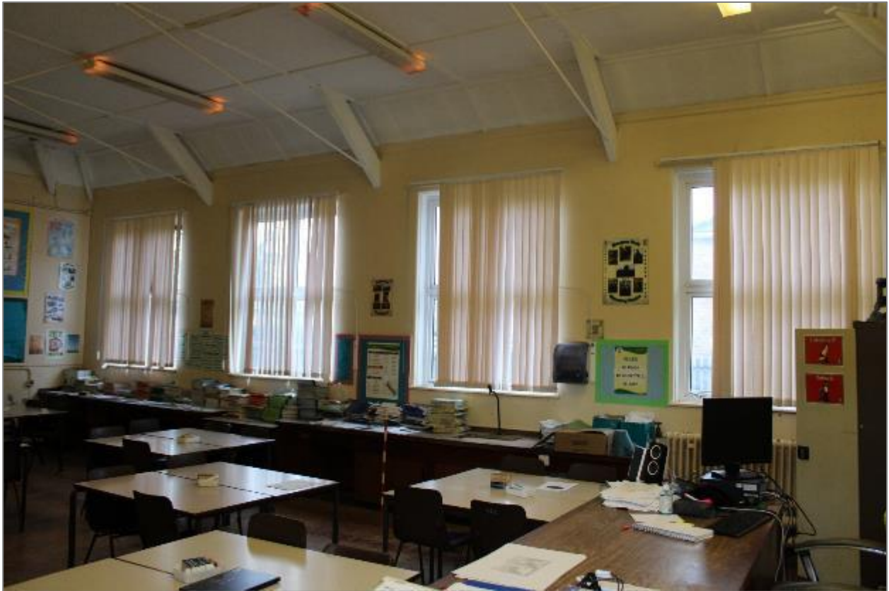
Photo 48: External wall of corner classroom.
