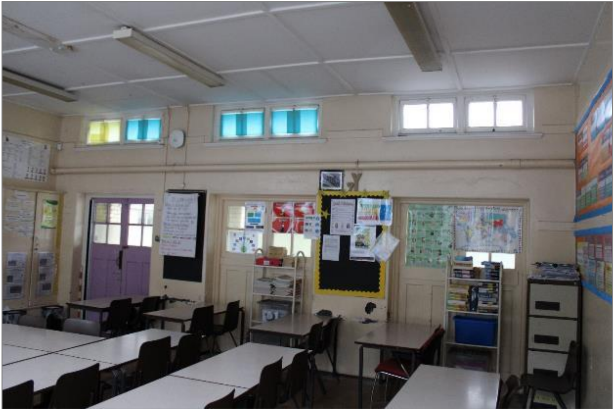
Photo 30: Internal wall in a standard classroom adjacent to covered walkway.
