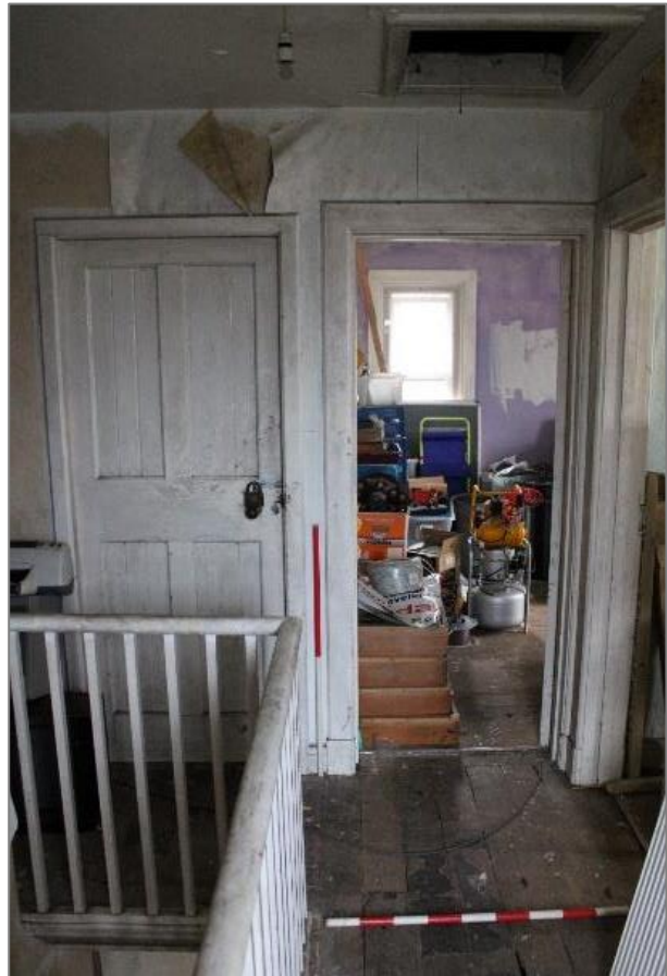
Photo 79: First floor landing. Facing southeast. 1 x 1m scale.
