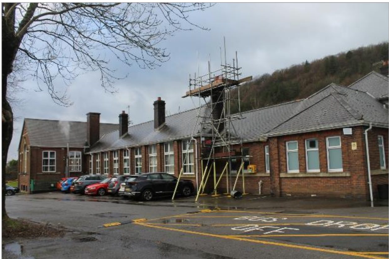
Photo 4: Southeast facing façade. Facing west.
