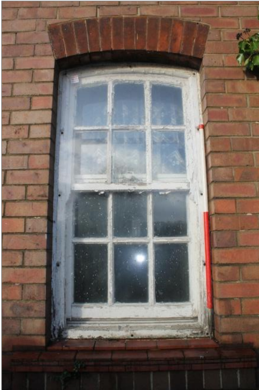
Photo 68: Southeast facing façade – ground floor window.
