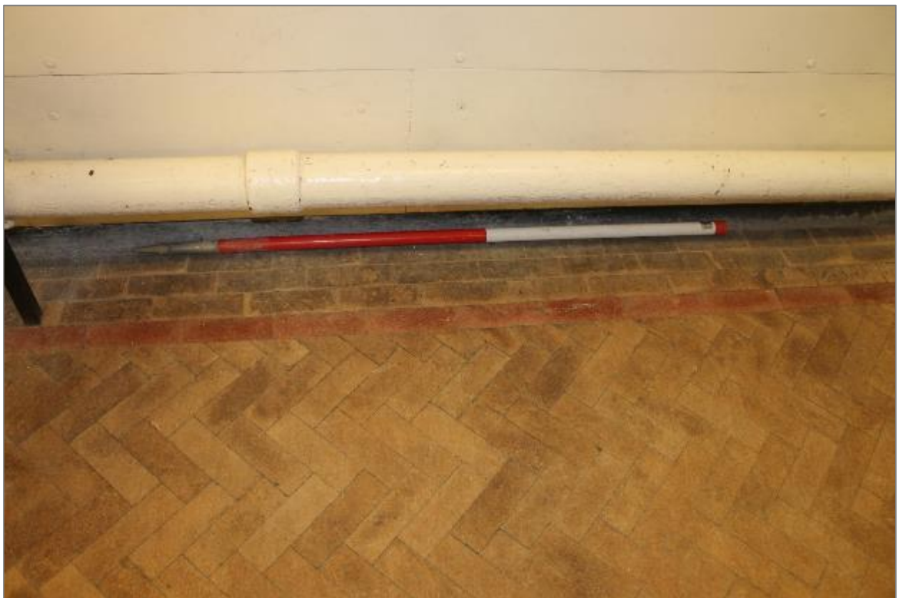
Photo 27: Floor in standard classroom. 1 x 1m scale.
