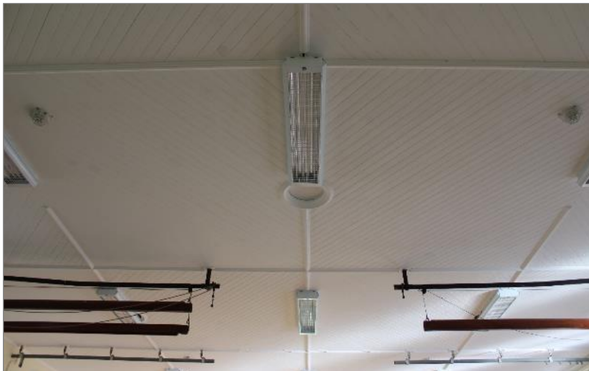
Photo 93: Interior of the gymnasium, ceiling detail.
