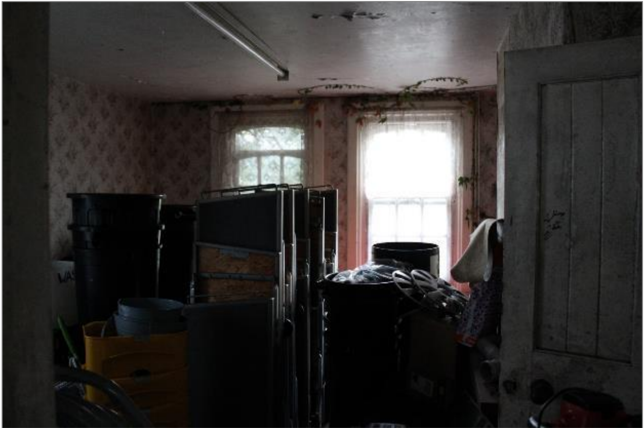
Photo 76: Front room 2. Facing southwest.
