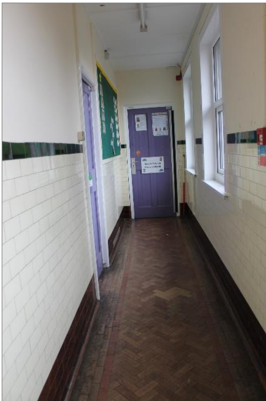
Photo 39: Corridor leading to first floor classroom. 1 x 1m scale.
