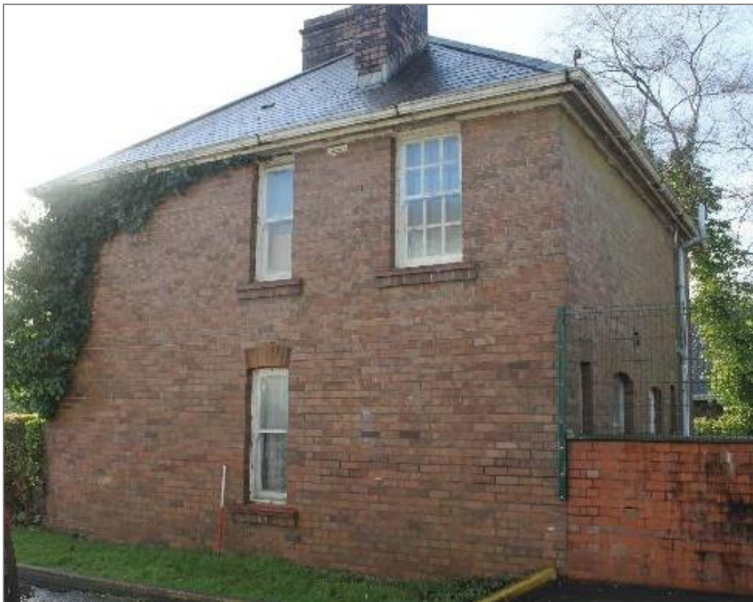
Photo 73: Northeast facing façade. 1 x 1m scale.
