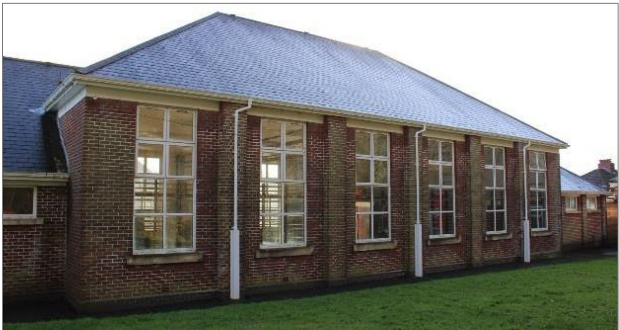
Photo 88: Gymnasium, northwest façade.
