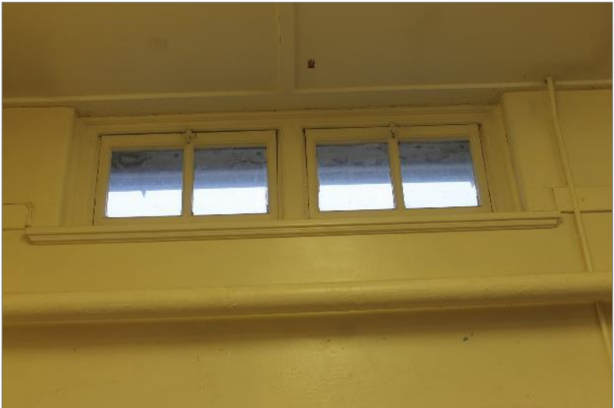
Photo 31: Windows and exposed pipework above double doors in a standard classroom.
