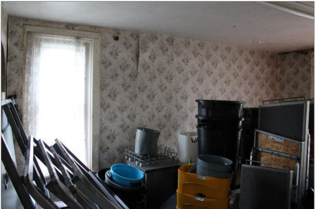
Photo 77: Front room 2. Facing southeast.
