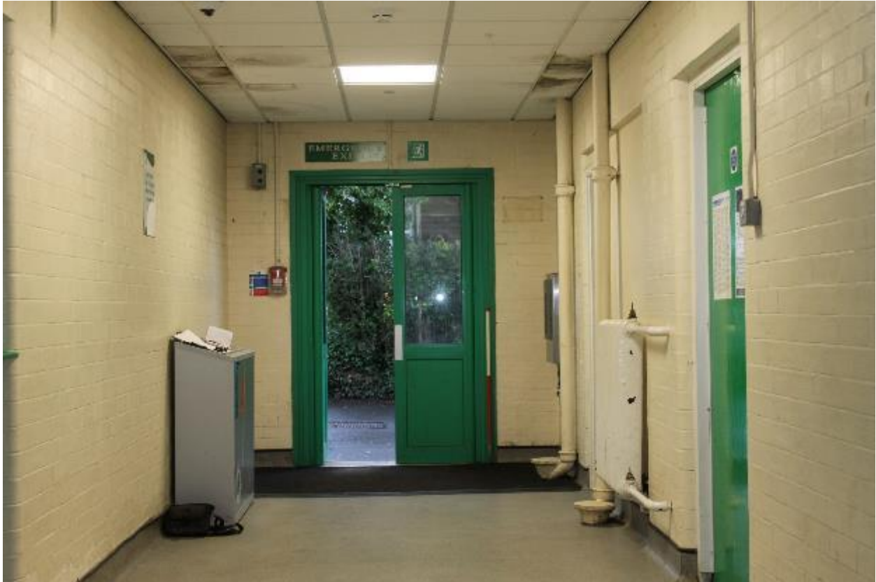
Photo 53: Entrance corridor. Facing northeast. 1 x 1m scale.
