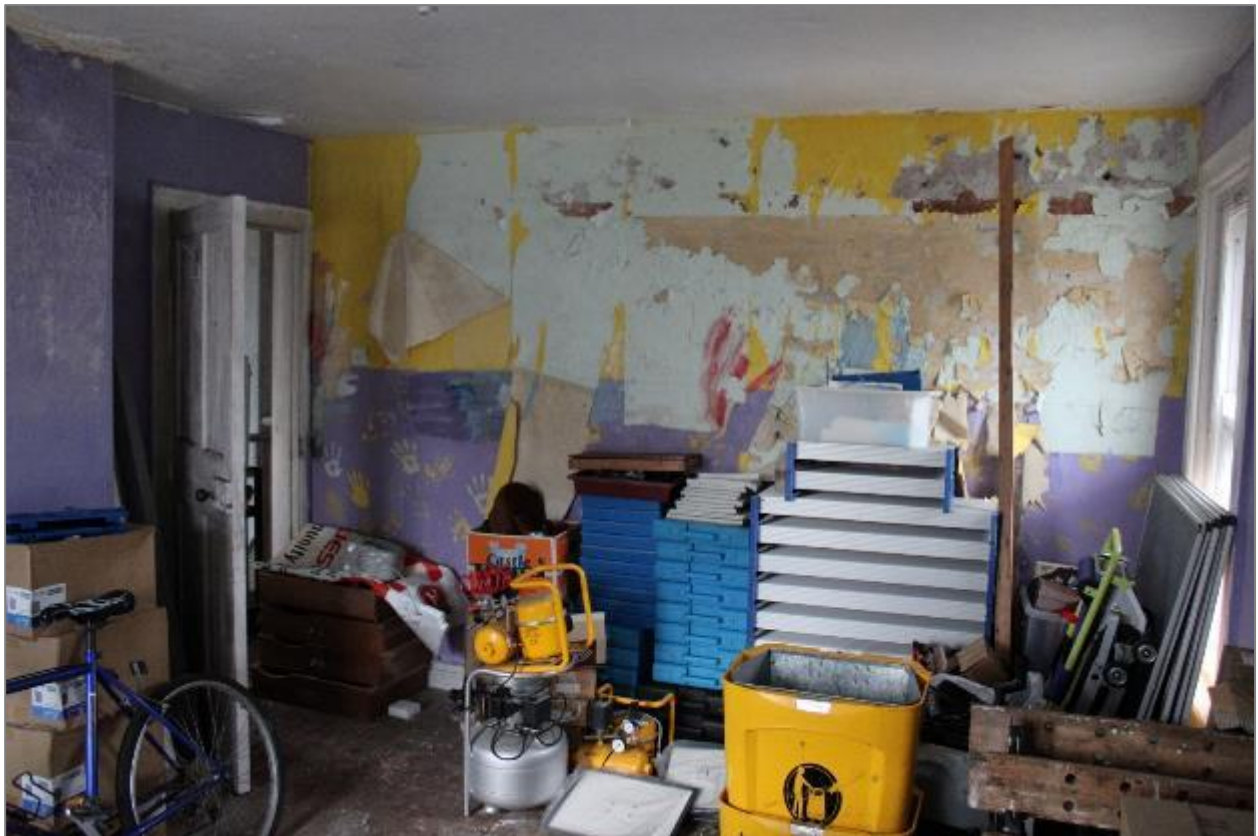
Photo 83: Bedroom 2. Facing northeast.
