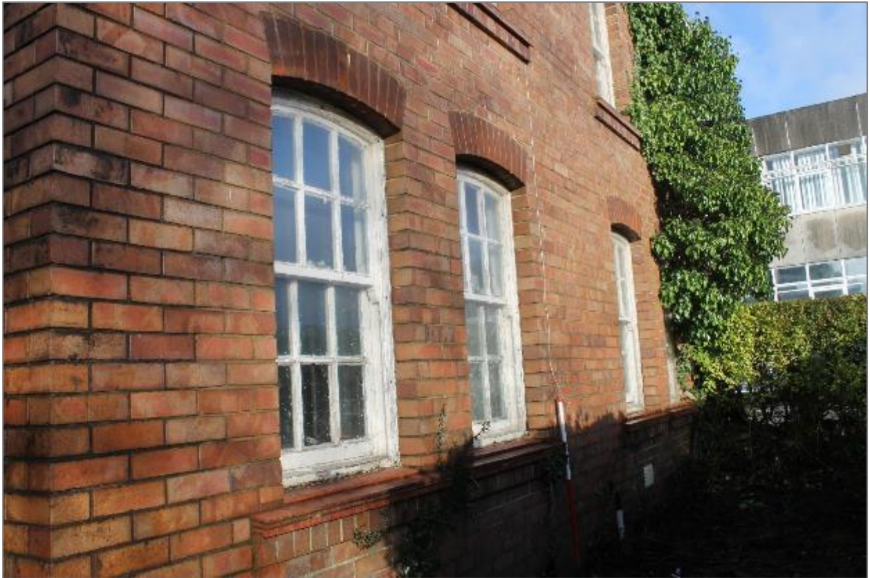
Photo 66: Southeast facing façade of former caretaker's house – ground floor. 1 x 1m scale.
