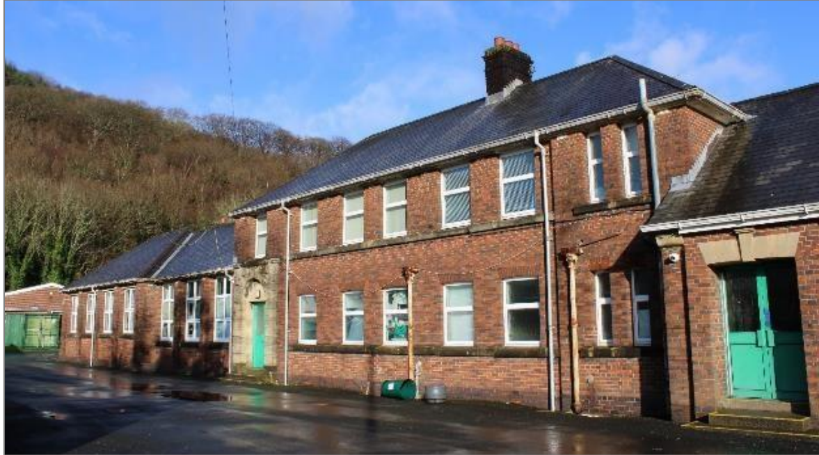
Photo 13: Southwest facing façade. Facing north.
