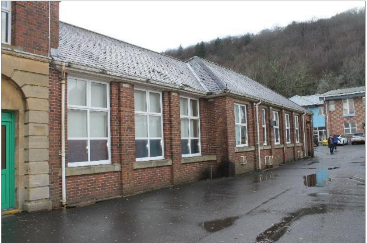
Photo 6: Northeast facing façade – north end. Facing northwest.
