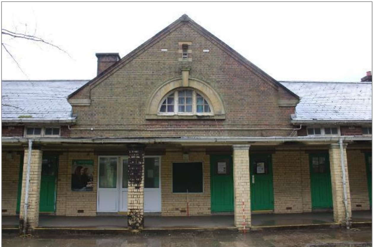
Photo 20: The central classroom on the southeast range of the quadrangle. 1 x 1m scale.
