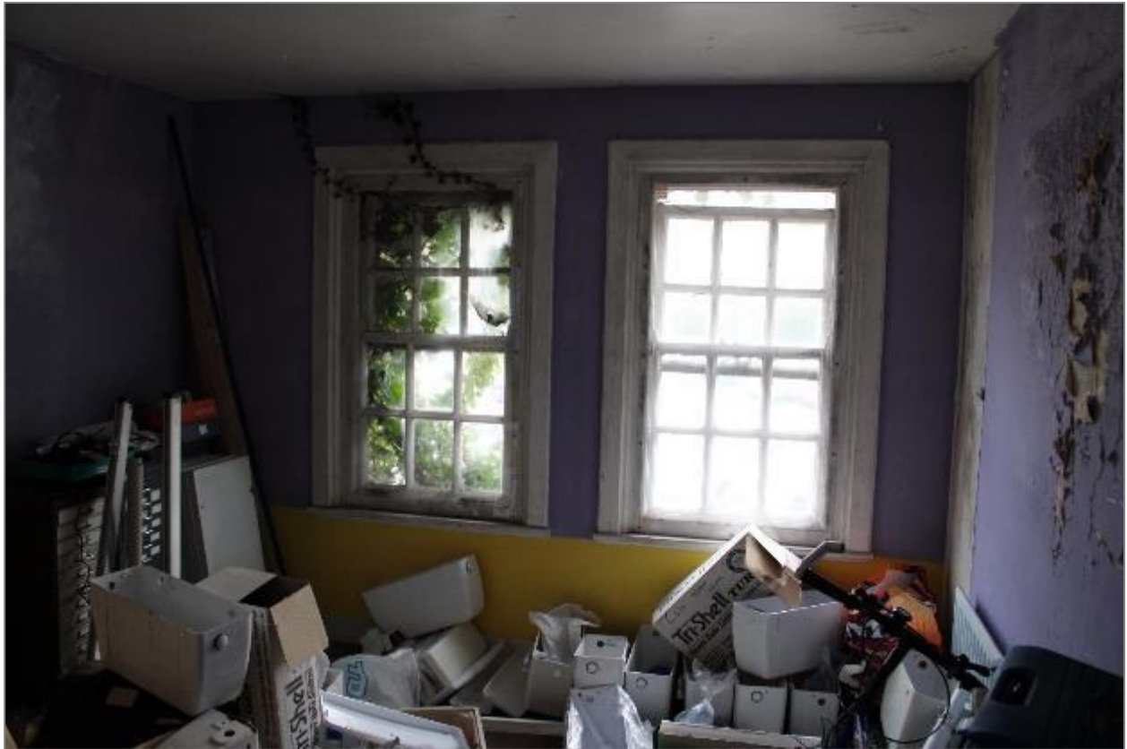
Photo 82: Bedroom 2. Facing southwest.
