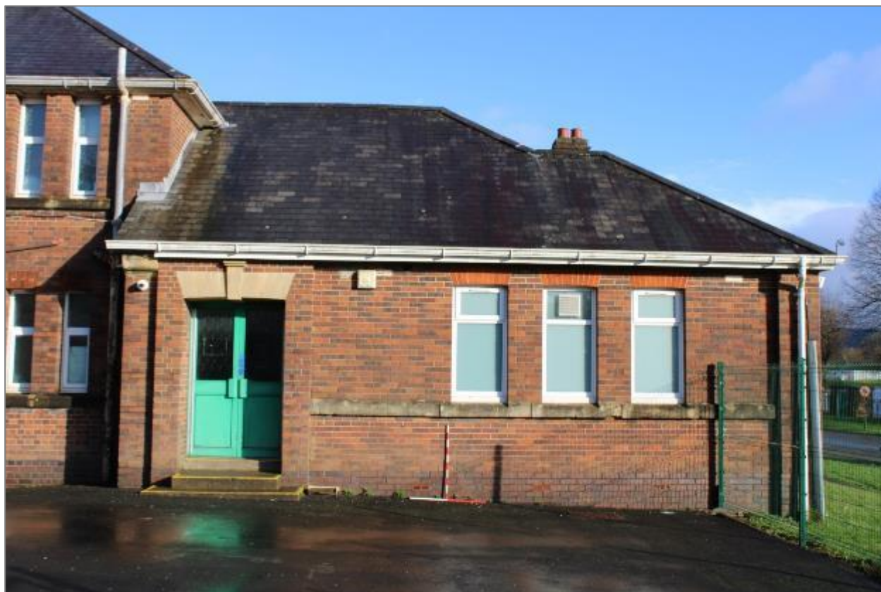
Photo 16: Southwest facing façade – southern end. Facing northeast. 2 x 1m scale.
