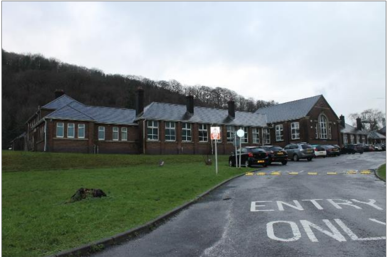
Photo 1: Southeast facing façade. Facing north.
