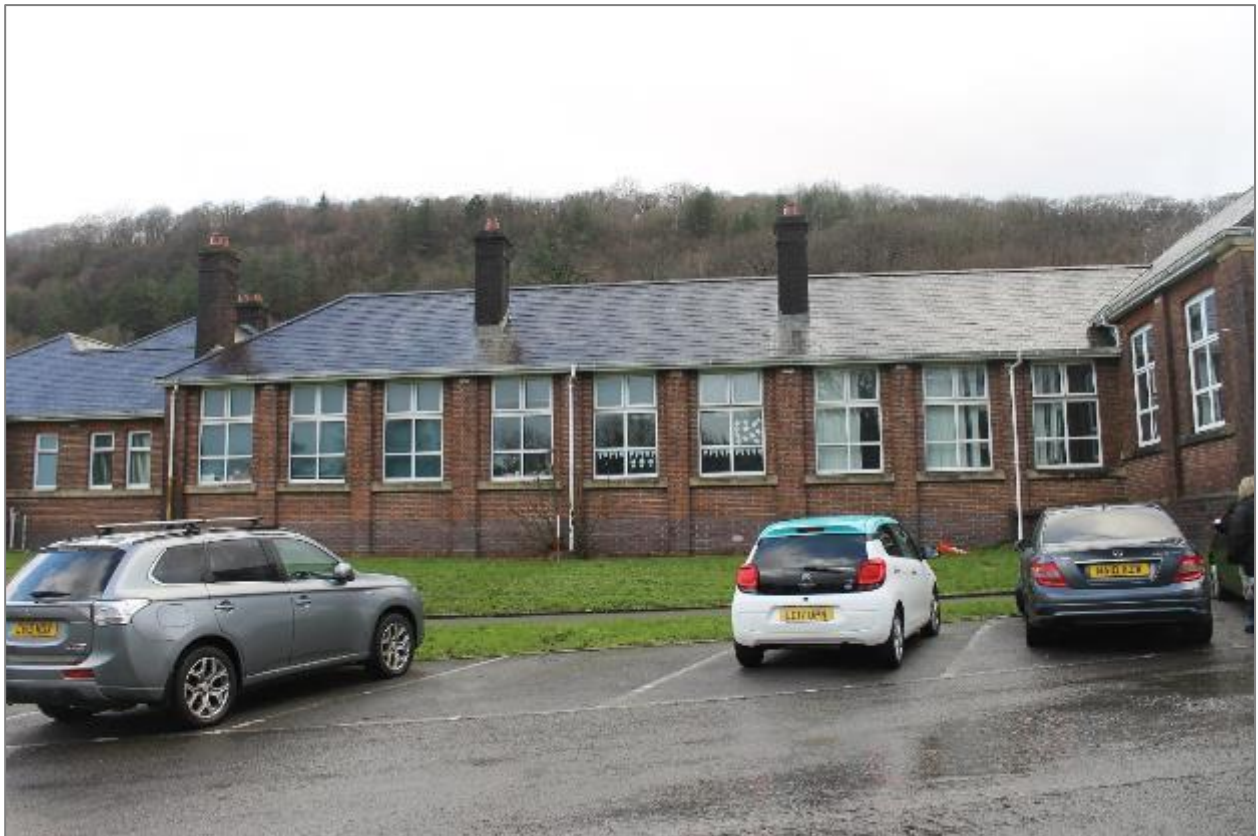
Photo 2: Southeast facing façade. Facing northwest. 1 x 1m scale.
