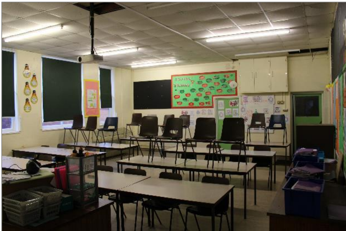
Photo 41: Corner classroom wall with entrance to storerooms.
