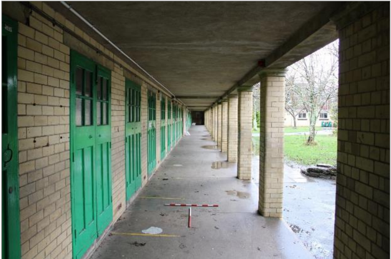
Photo 17: Walkway along the northwest range of the quadrangle. Facing northeast. 2 x 1m scales.
