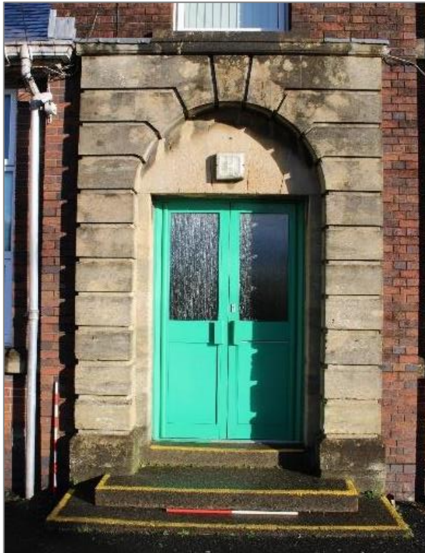
Photo 14: Doorway in southwest facing façade. 1 x 1m scale.
