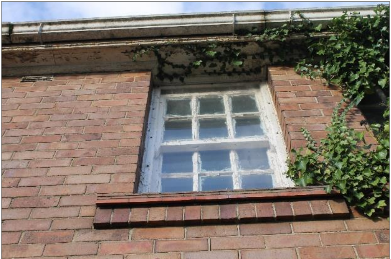
Photo 67: Southeast facing façade – first floor window.
