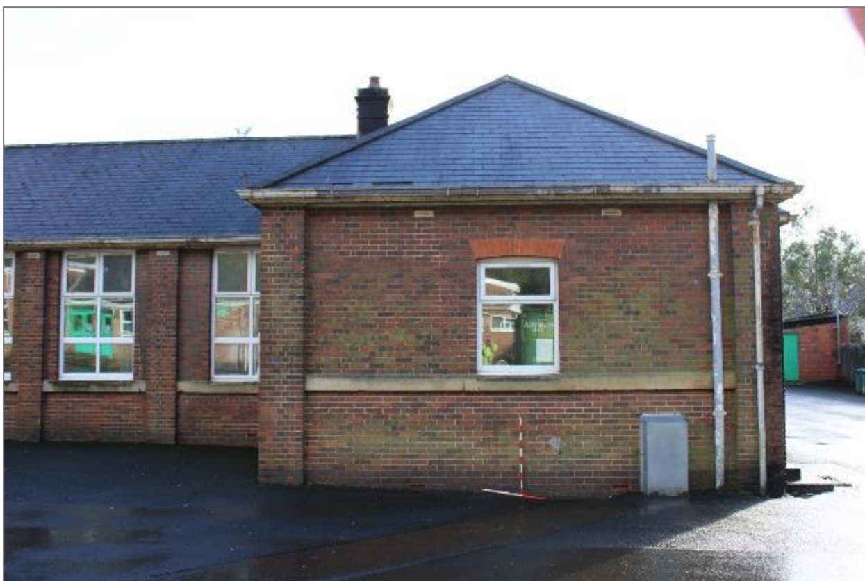
Photo 12: Northwest facing façade – western end. Facing southeast. 2 x 1m scale.
