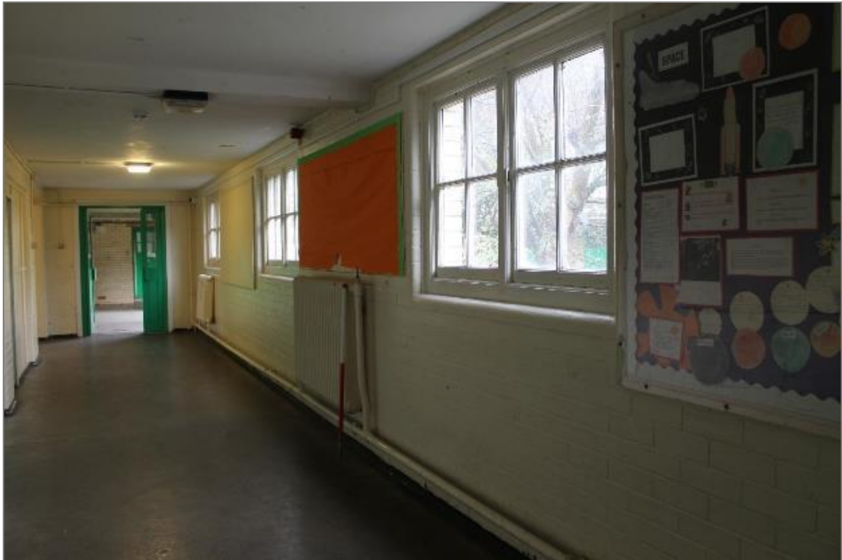
Photo 61: Corridor in the southwest range. Facing northwest. 1 x 1m scale.
