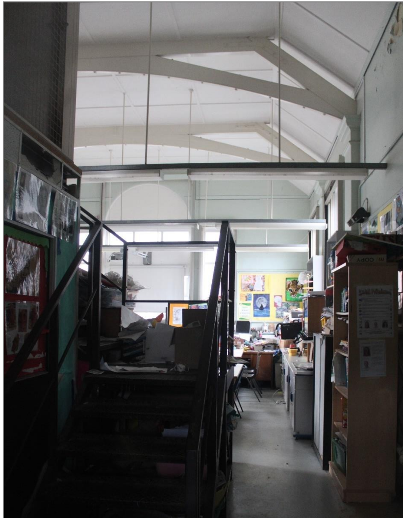
Photo 52: Northwest central hall, viewed from the entrance to the southeast.
