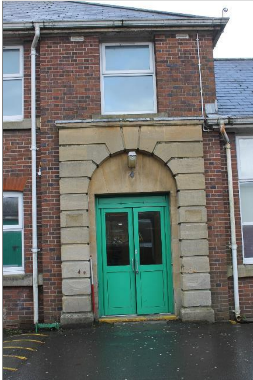
Photo 8: Doorway in northeast facing façade. Facing southwest. 1 x 1m scale.
