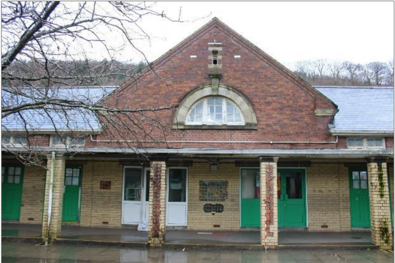
Photo 21: The central classroom on the northwest range of the quadrangle. 2 x 1m scale.
