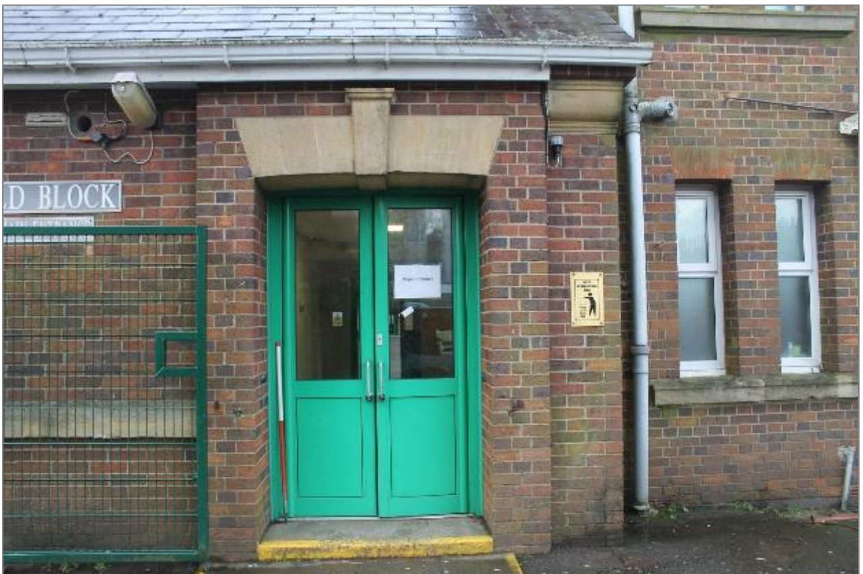
Photo 7: Doorway at southern end of northeast facing façade. Facing southwest. 1 x 1m scale.
