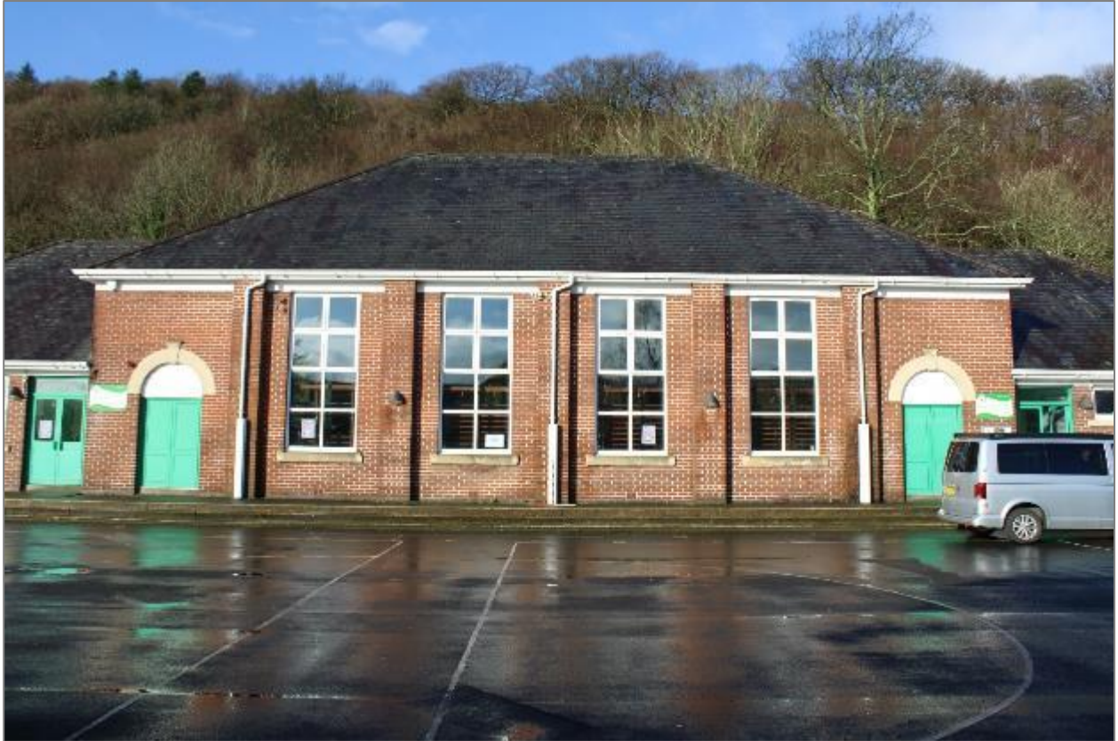
Photo 85: Gymnasium, southeast façade. Facing northwest.
