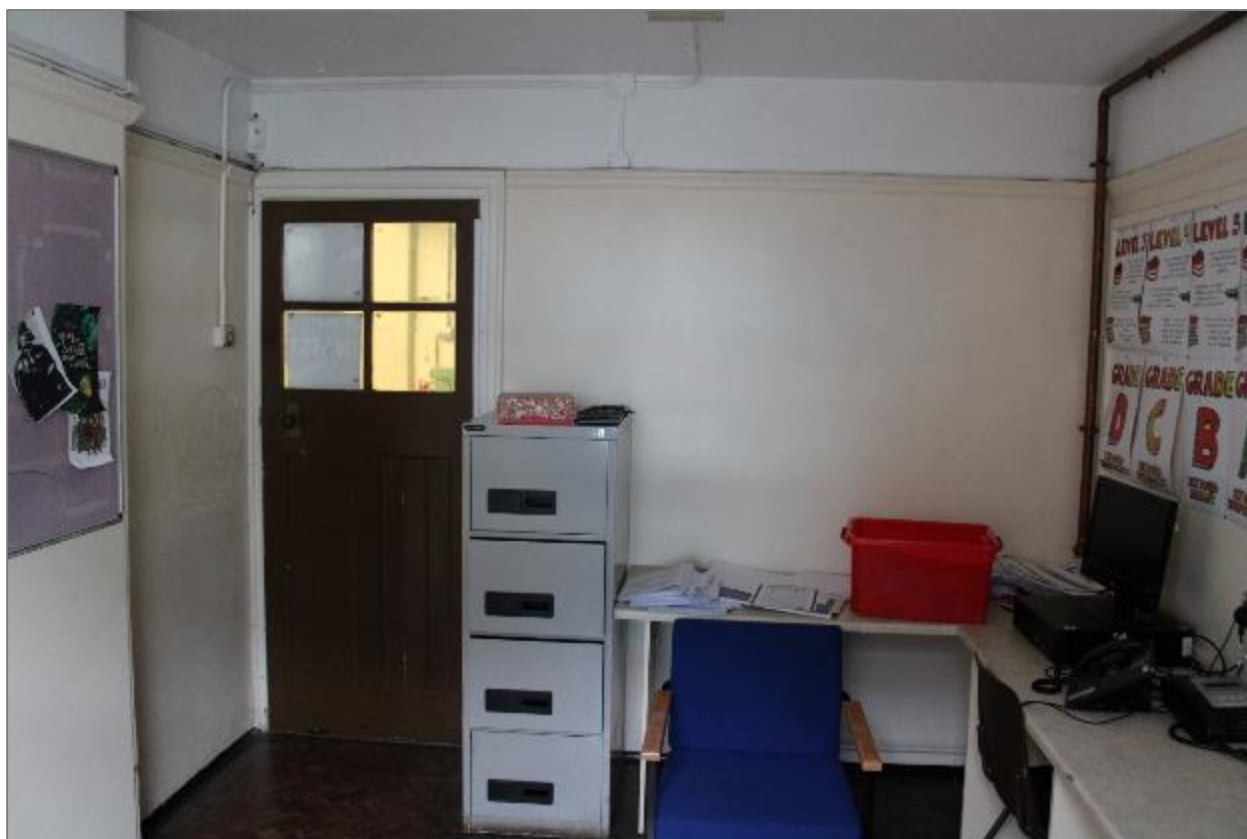
Photo 45: Office adjacent to corner classroom accessed via foyer.
