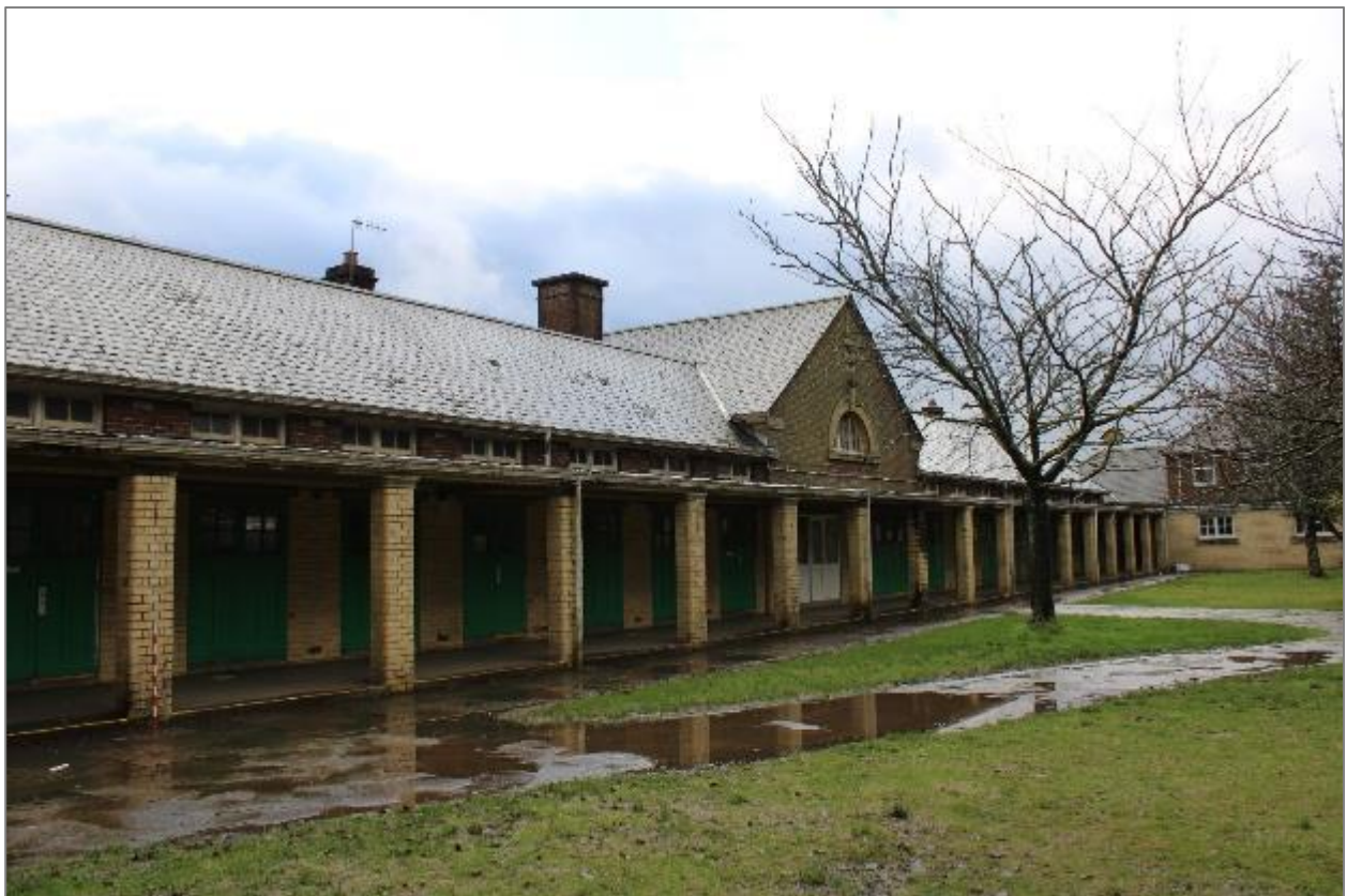
Photo 18: Walkway along the southeast side of the quadrangle. Facing south.
