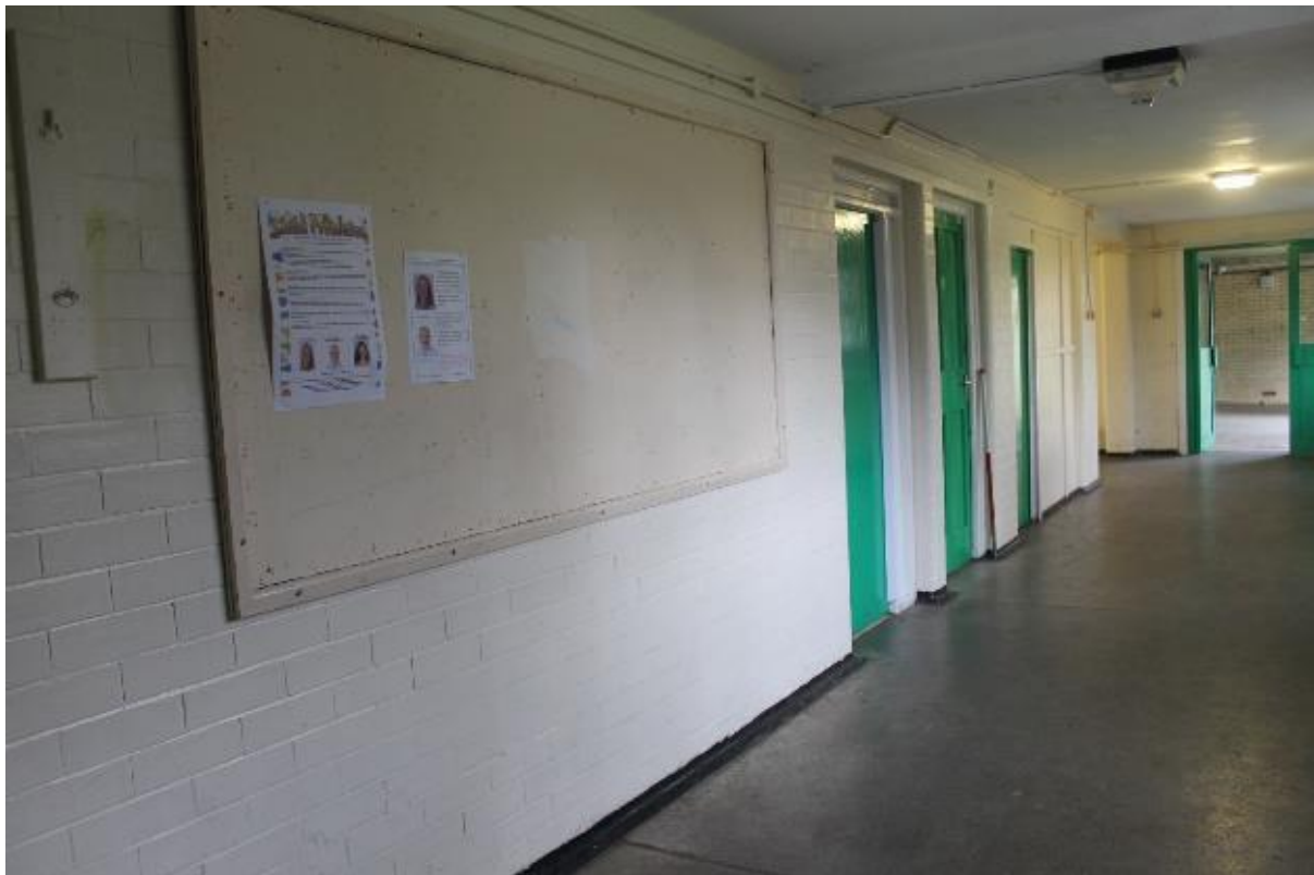
Photo 62: Corridor in the southwest range. Facing northwest. 1 x 1m scale.
