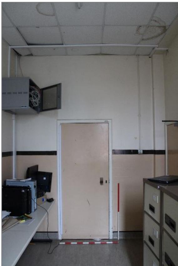
Photo 43: Storeroom located off corner classroom. 2 x 1m scales.
