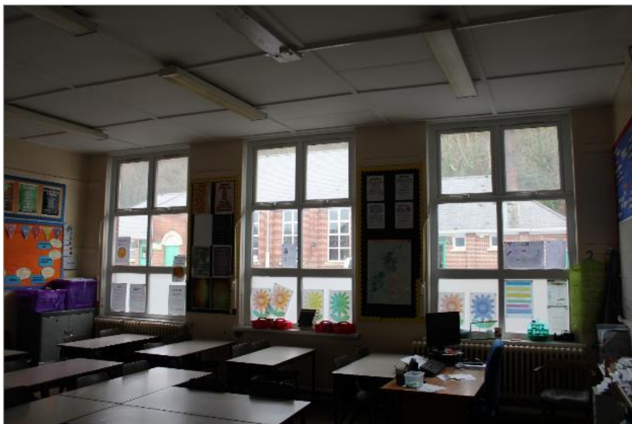
Photo 28: External wall of a standard classroom. Facing northwest.
