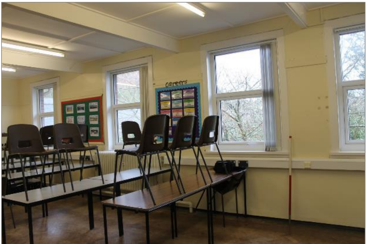
Photo 34: Wall looking out over the quadrangle in first floor classroom. 1 x 1m scale.
