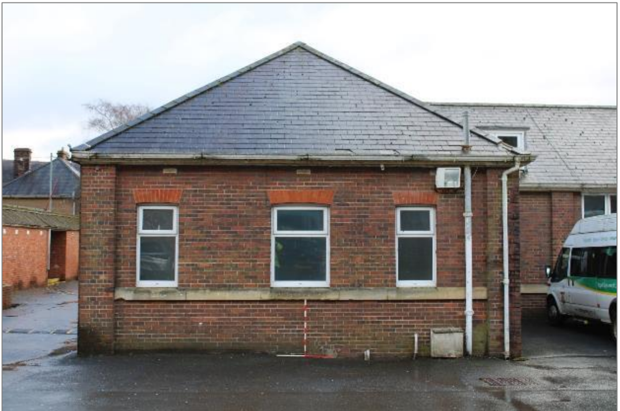
Photo 10: Northwest facing façade – northern end. Facing southeast. 2 x 1m scales.
