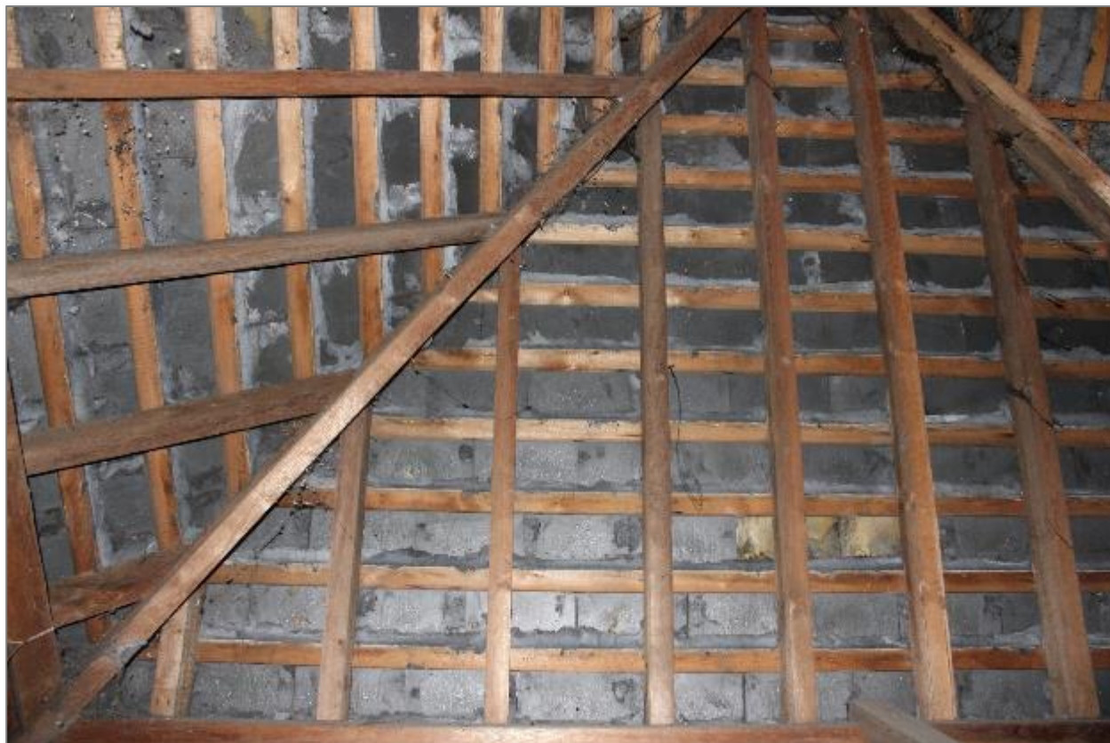
Photo 81: Internal roof structure, as viewed through the loft hatch.
