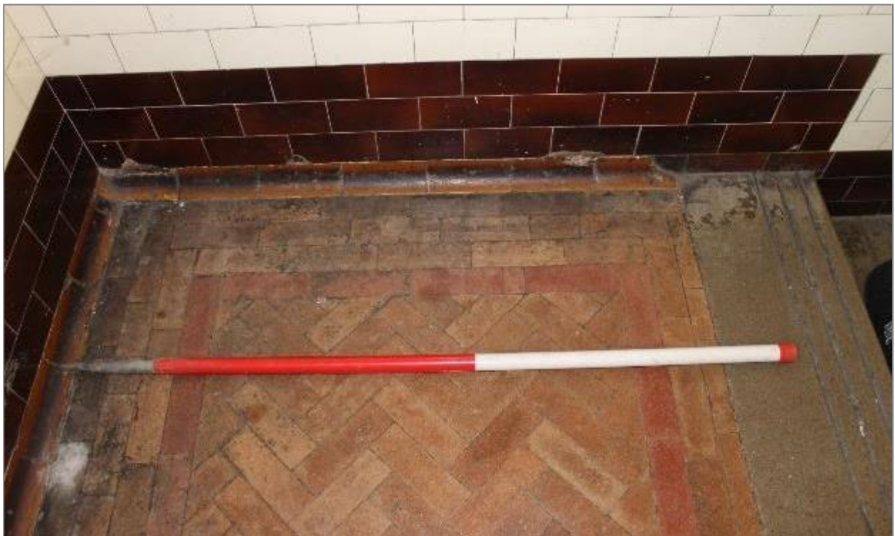
Photo 38: Floor detail of corridor leading to first floor classroom. 1 x 1m scale.
