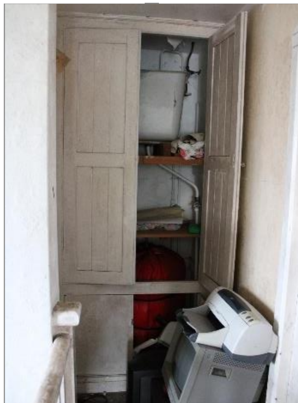
Photo 80: Airing cupboard on first floor landing. Facing northeast.
