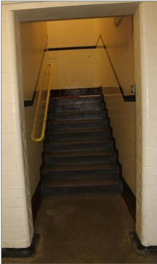
Photo 36: Lower stairway leading to first floor classroom. 1 x 1m scale.
