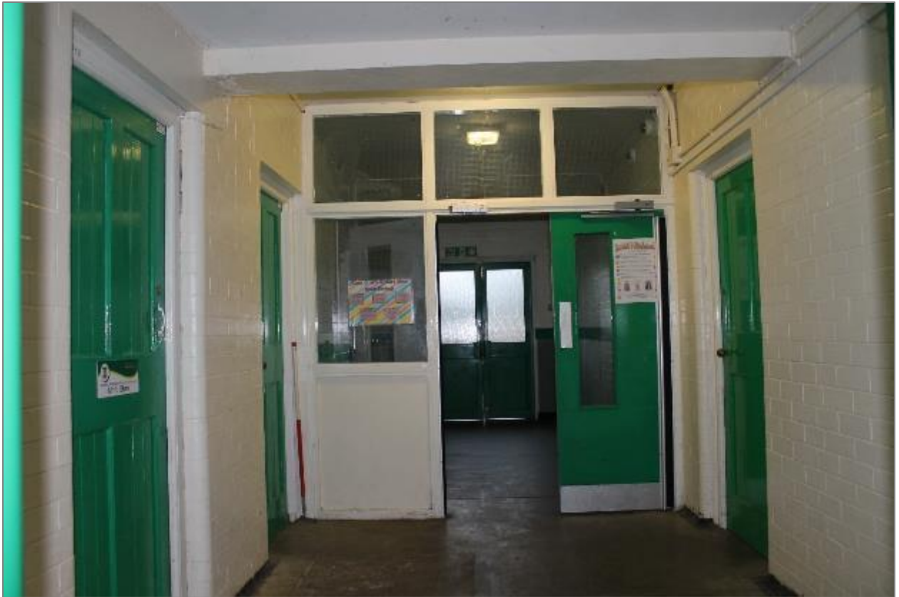
Photo 58: Entrance corridor in southern corner of the old block. Facing southwest. 1 x 1m scale.
