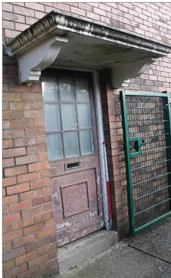
Photo 70: Front door detail on the southwest facing façade. 1 x 1m scale.
