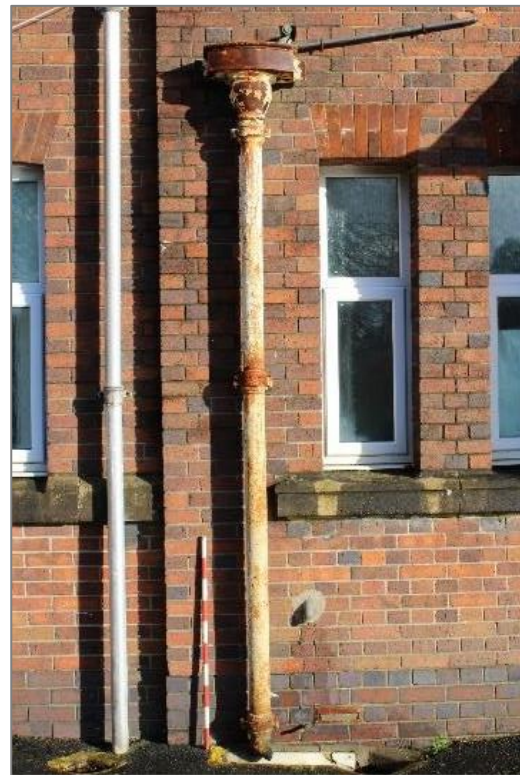
Photo 15: Downpipe on southwest facing façade. 1 x 1m scale.
