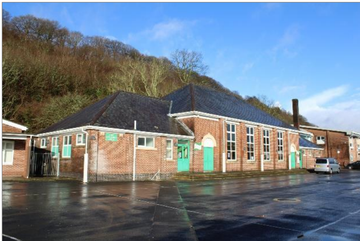
Photo 84: Gymnasium, southeast façade. Facing north.
