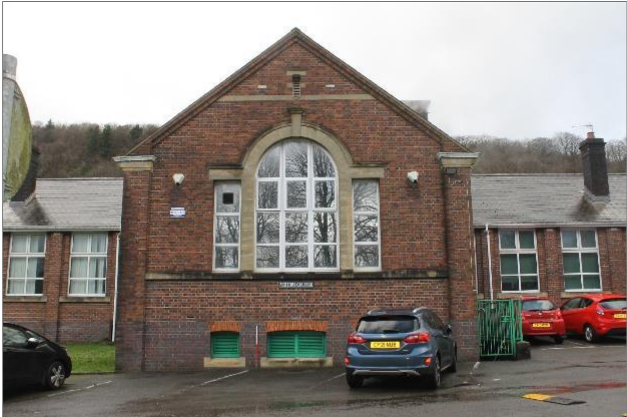
Photo 3: Southeast facing façade – extending hall. Facing northwest. 1 x 1m scale.
