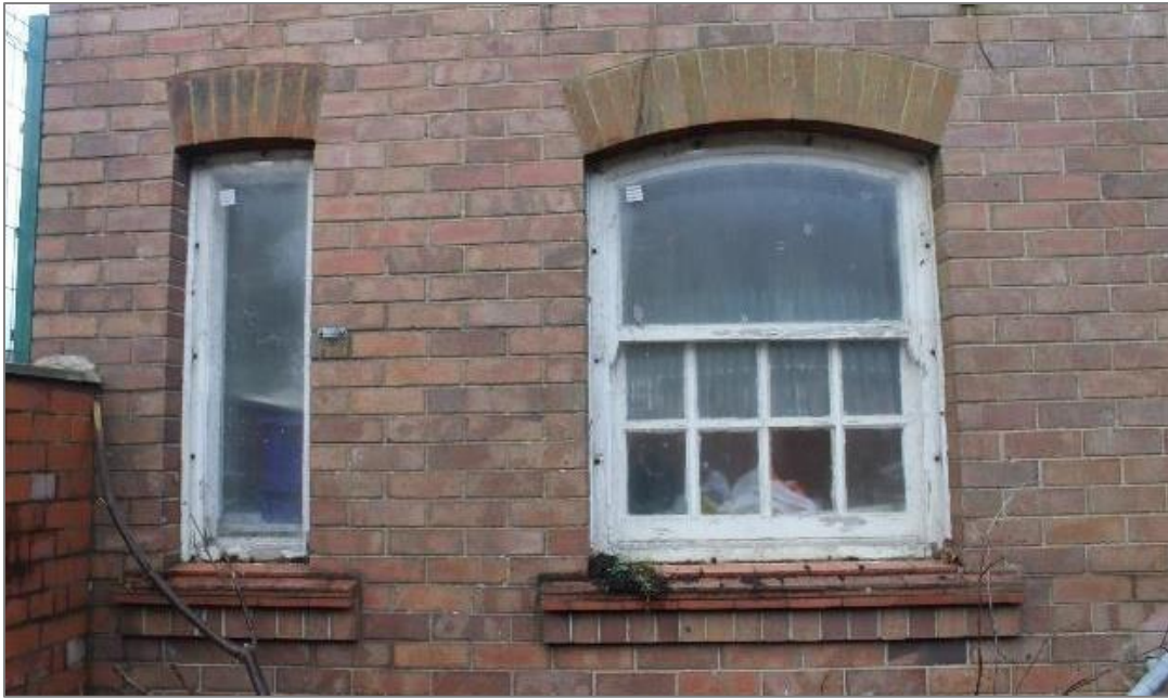
Photo 72: Northwest facing façade – ground floor windows.
