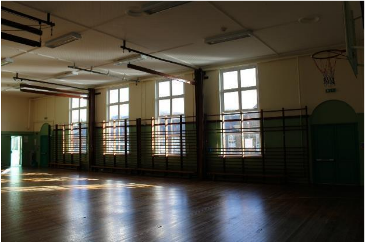
Photo 91: Interior of the gymnasium, facing west.
