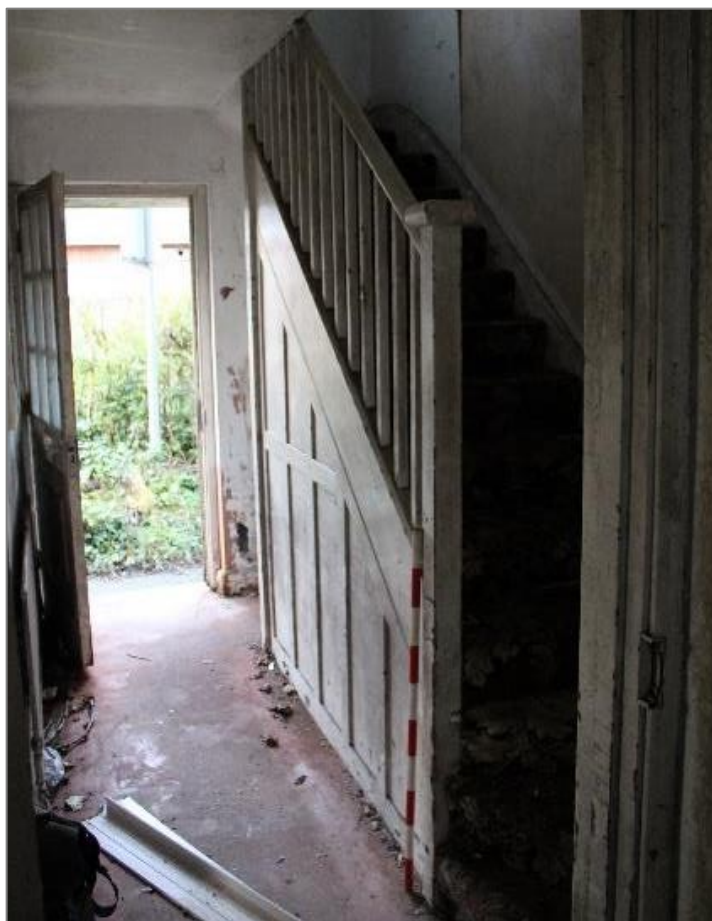
Photo 74: Entrance hall and stairs, facing southwest. 1 x 1m scale.
