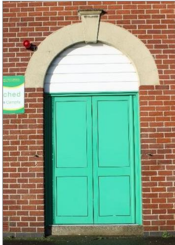
Photo 87: Gymnasium, door detail on the southeast façade.
