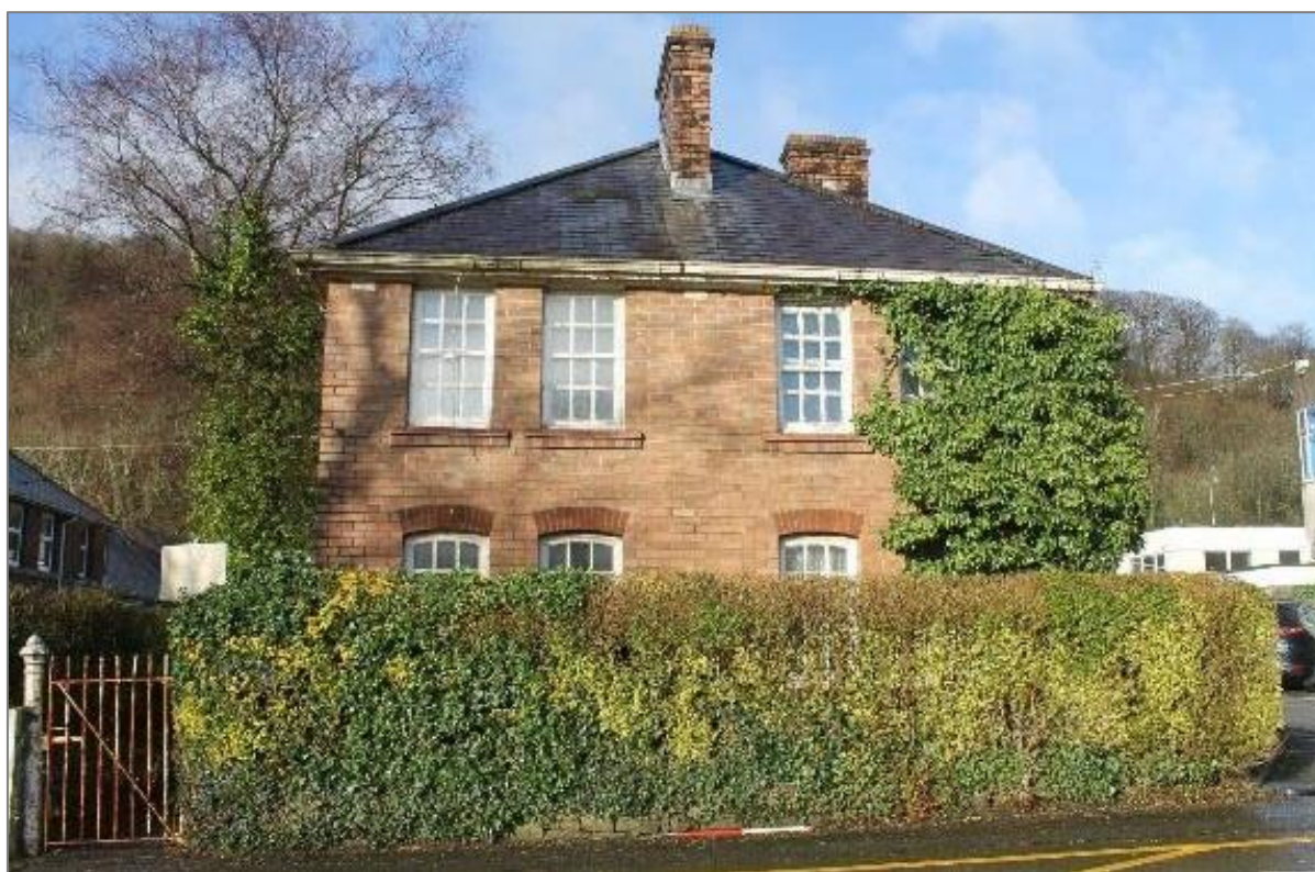
Photo 65: Southeast facing façade of former caretaker's house.
