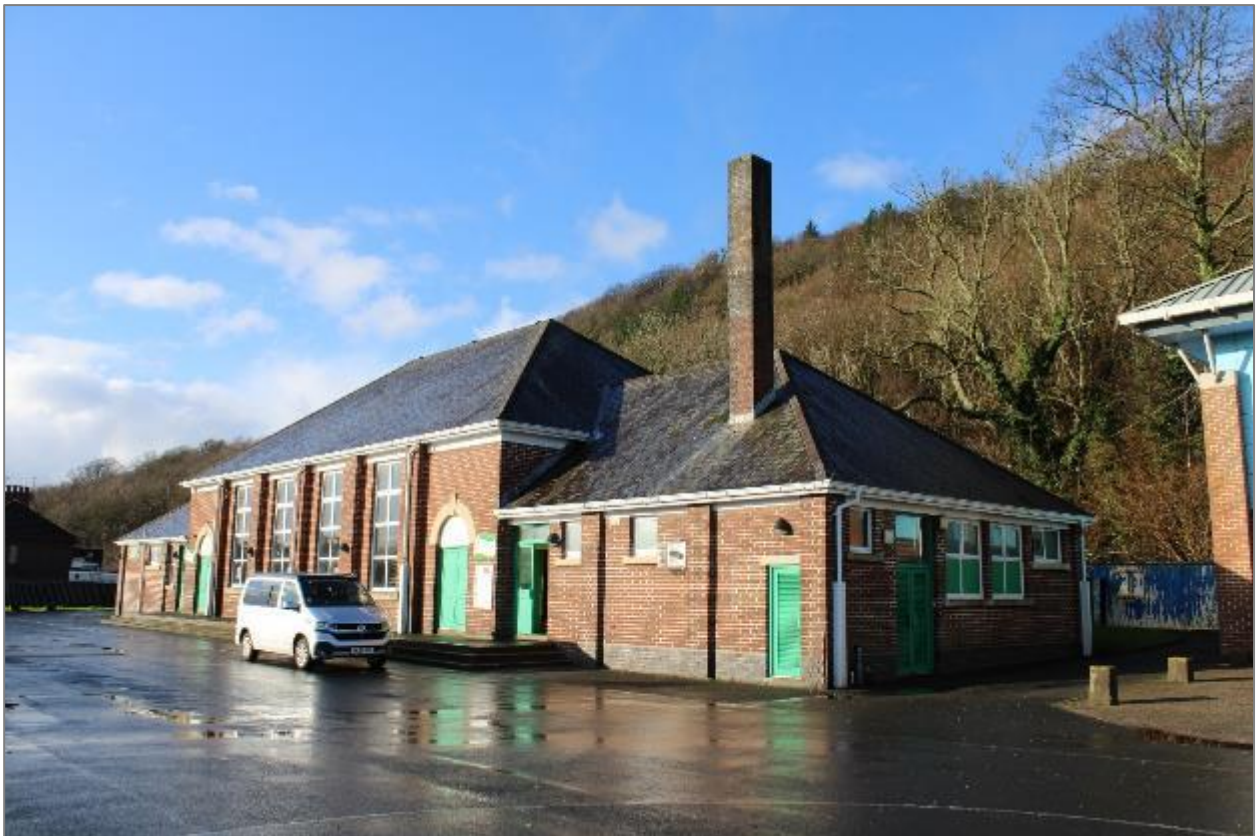
Photo 86: Gymnasium, southeast façade. Facing west.
