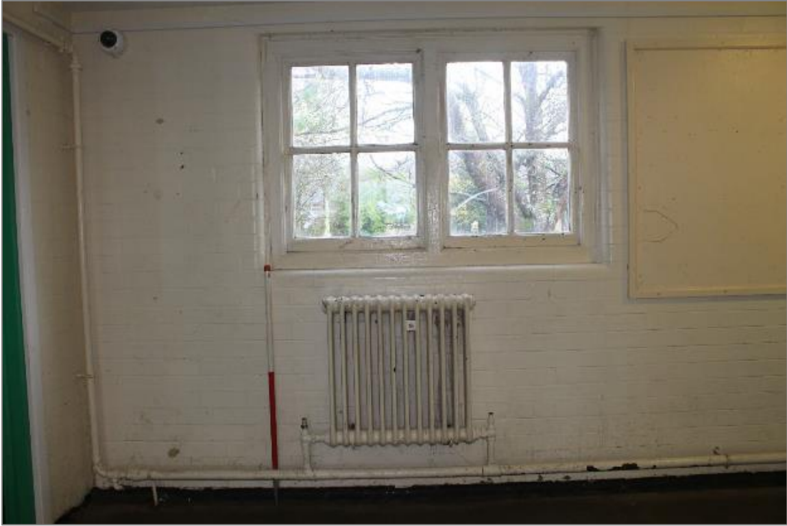
Photo 63: Corridor in the southwest range. Facing northeast. 1 x 1m scale.
