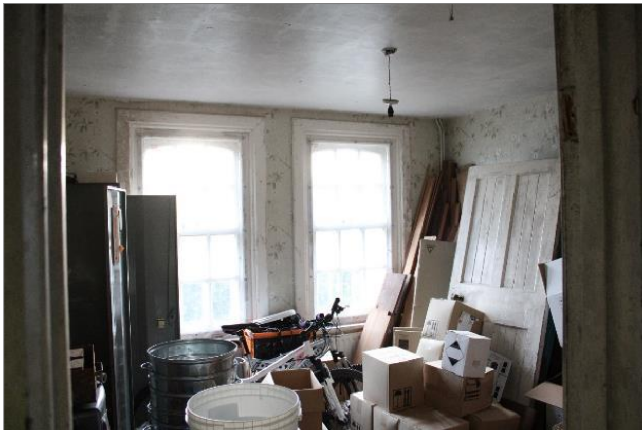
Photo 75: Front room 1. Facing west.
