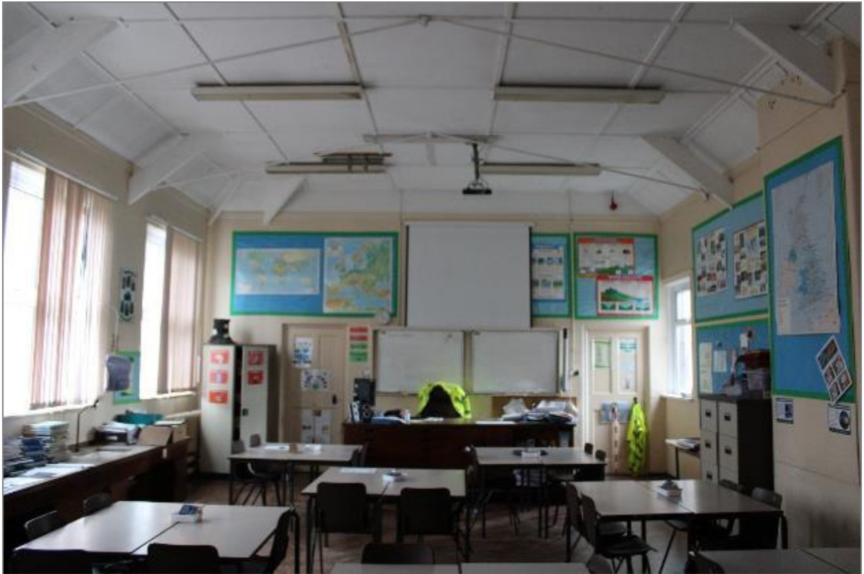
Photo 46: Corner classroom - doors to office visible in the northwest wall. 1 x 1m scale.
