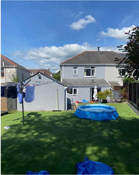
View of rear elevation and lawn area with timber panel boundaries to both neighbours
