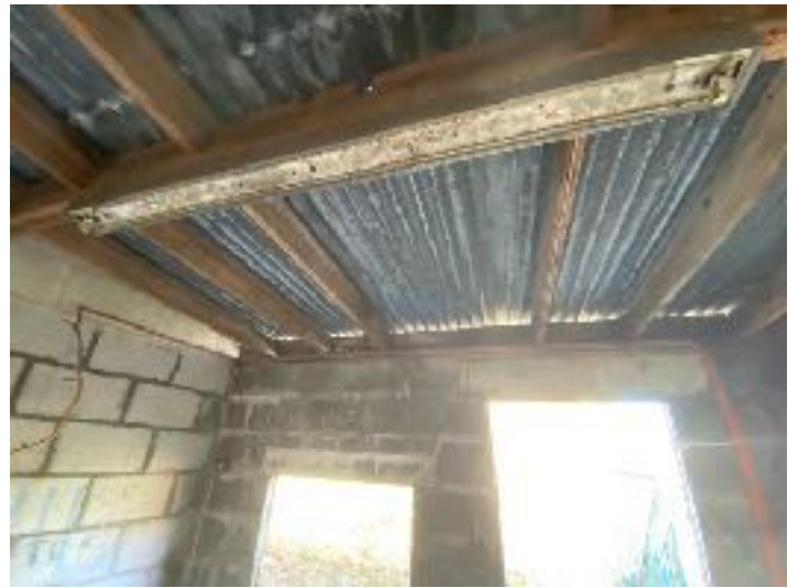
Internal view of the block work and corrugated sheet metal roof building
