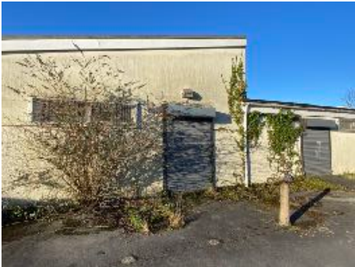
North east elevation of the former changing rooms and roller shutter doors
