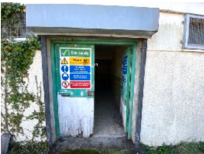
Access into the former changing rooms
