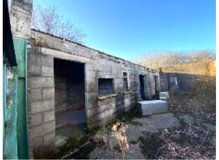
North west elevation of the block work building with no windows or doors.
