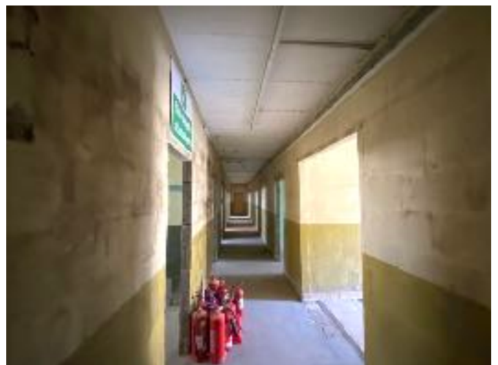
Internal corridor within the former changing rooms building with many individual rooms
