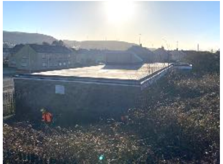
Bitumen felt flat roof in good condition over the whole building
