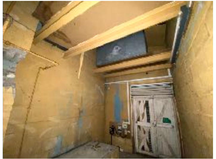
Raised plywood section of the roof for the location of the water tanks
