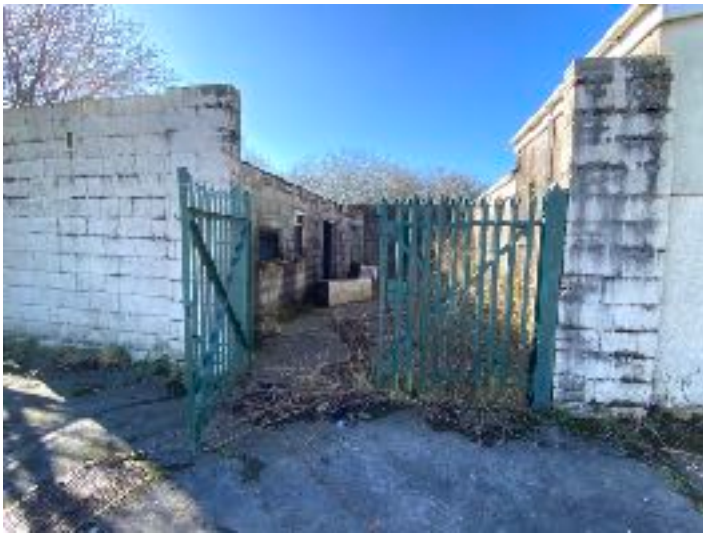
Access into the concrete court yard between the buildings
