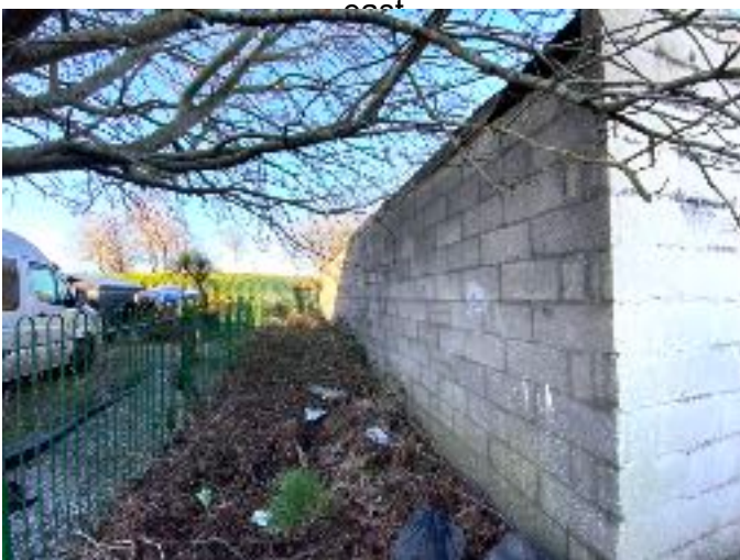
Bramble scrub between south east block work building and the residential property boundary to the south east
