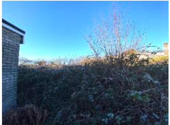
Head height bramble scrub to the rear south west side of the building
