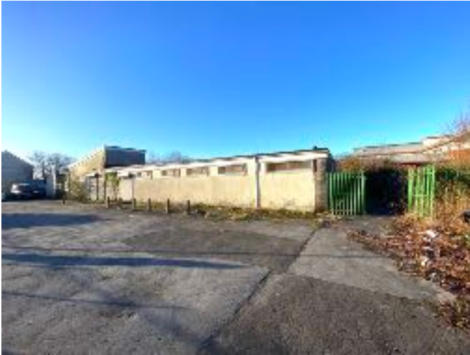
North east elevation of the building and tarmac hardstanding viewing south west
