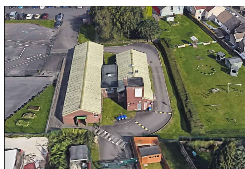
Photo 12 (3D IMAGE OF SITE)
