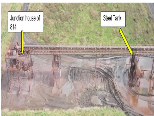
Fig 21 : Junction house 814 , Steel tank
