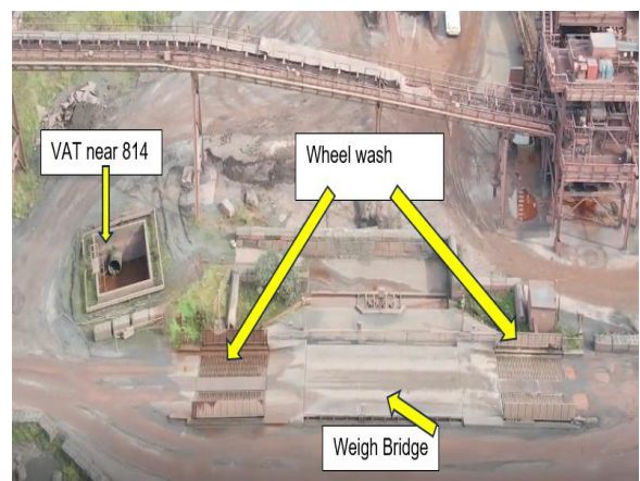
Fig 22: Vat, Wheel wash, Weigh Bridge
