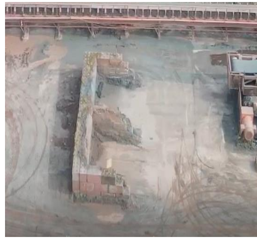
Fig 24: Lego block wall
