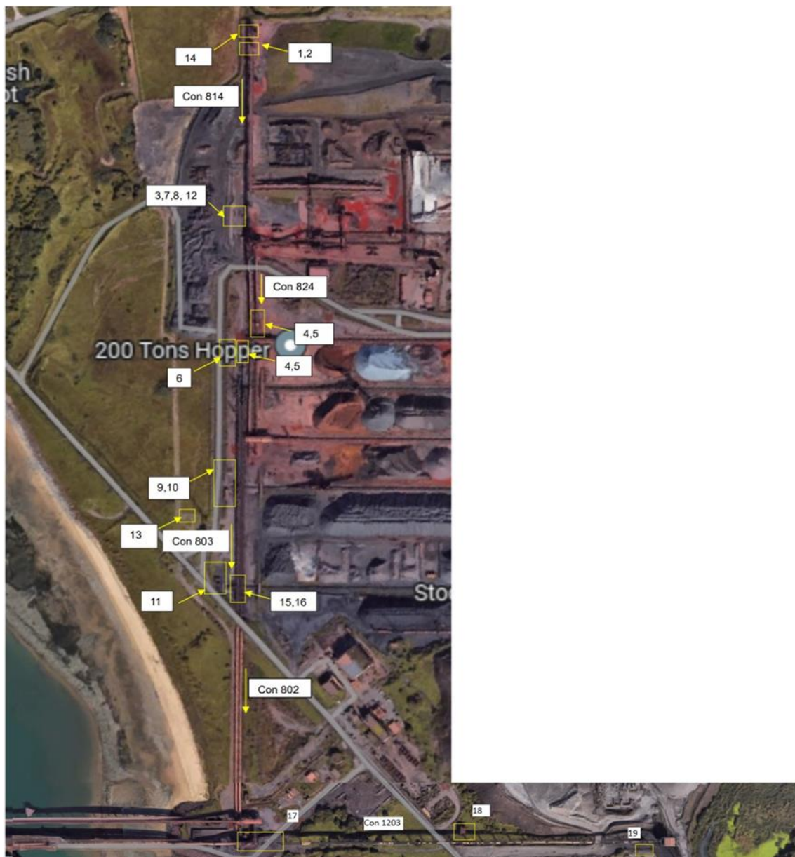
Fig 4 Aerial Photo showing the area of Phase 1(North Conveyor North -South and East-West)
