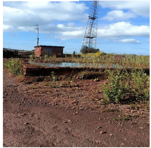
Fig 14 : Building at end of 806
