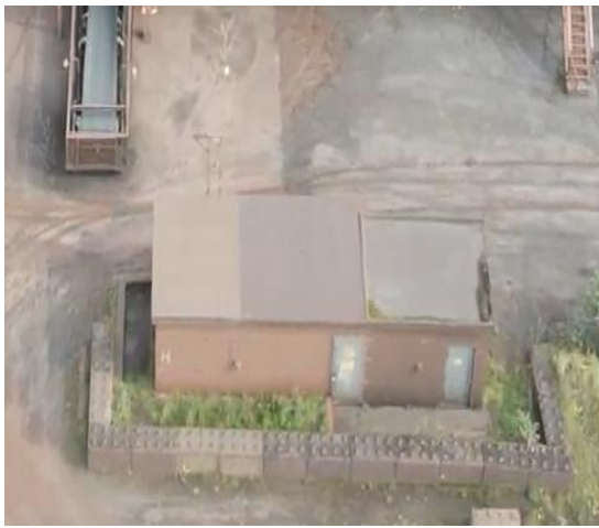
Fig 23 : Building at end of 806
