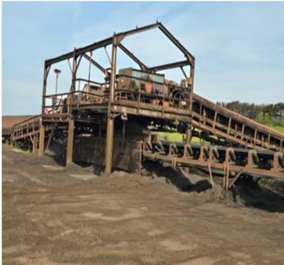
Fig.14 Transfer house at Junction 882/883
