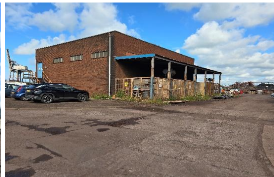
Fig 11. Harbor Jetty Substation
