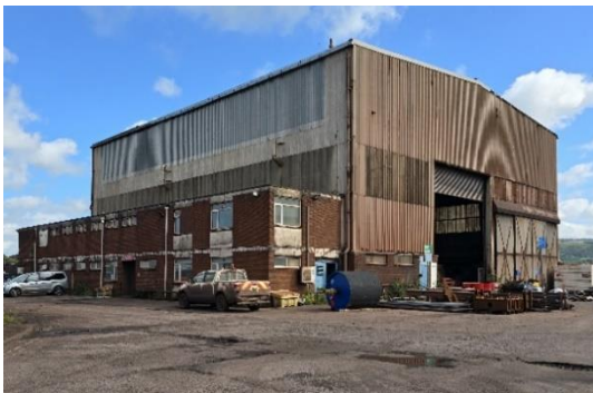
Fig 10 . Mobile Plant Workshop
