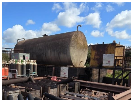
Fig 17. Mobile Plant workshop
