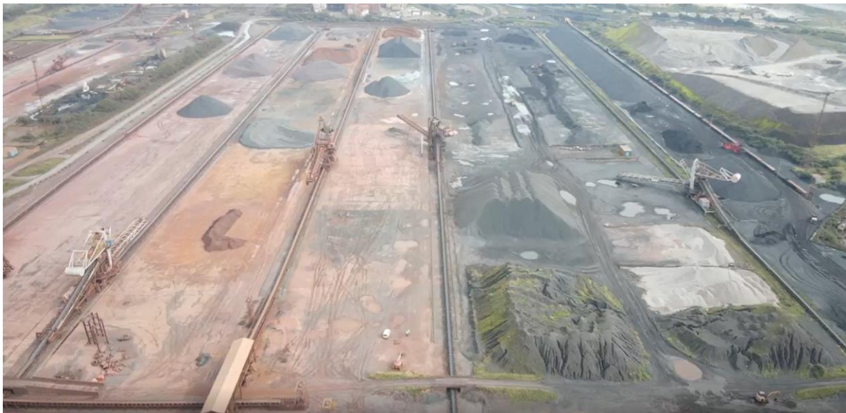
Fig -1a: Overview of Phase 2A (Burdening Area)
