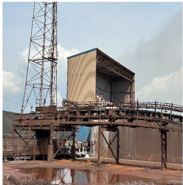
Fig.17 Additive Bunker an Conv 869
