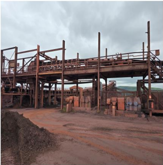
Fig.6 Structural steel for Conv. 823
