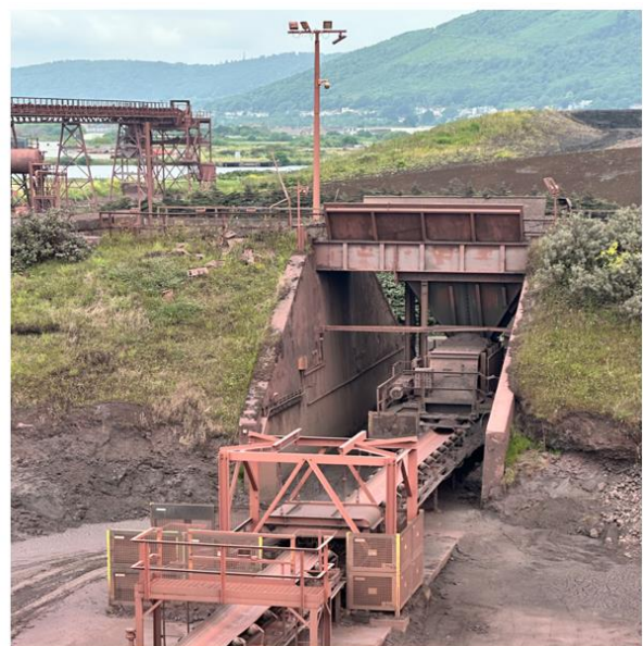
Fig.15 Screen & Unloading steel hopper/ramp
