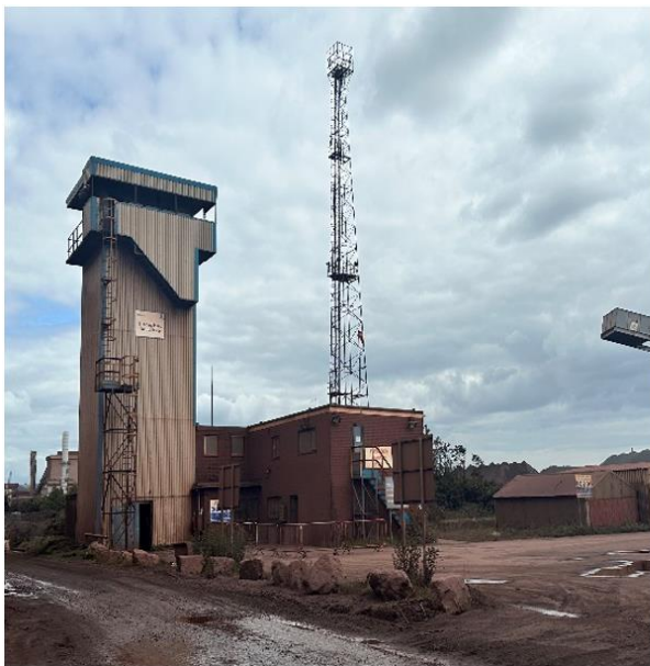
Fig.16 Blending Plant office
