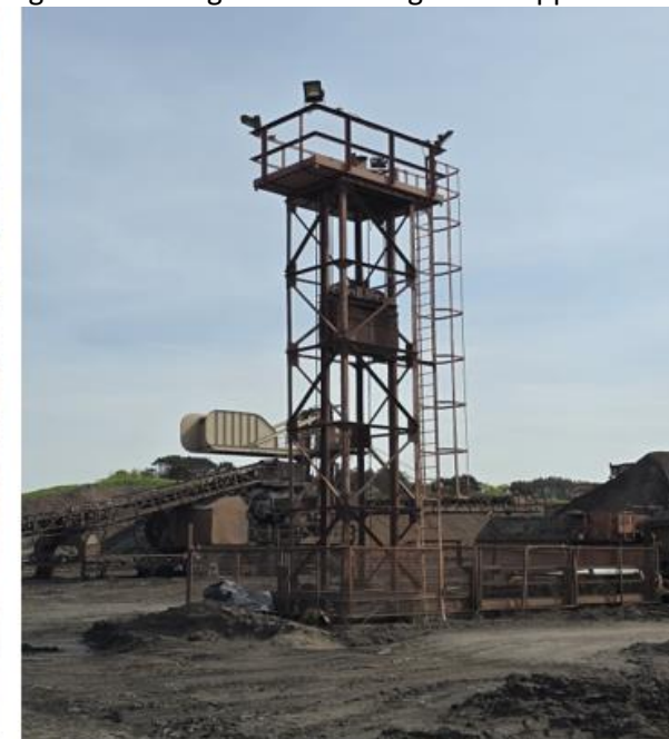
Fig.21 Drop Weigh Tower
