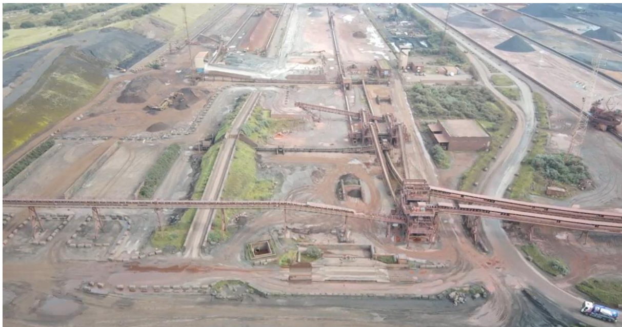
Fig -2a: Overview of Phase 2B (Blending area)
