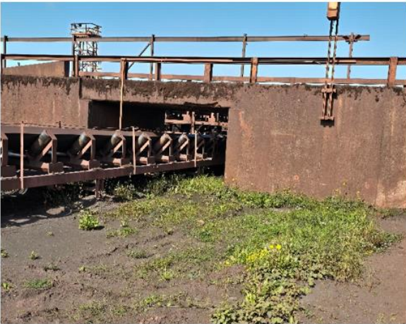
Fig. 12 Ramp on Conv.806
