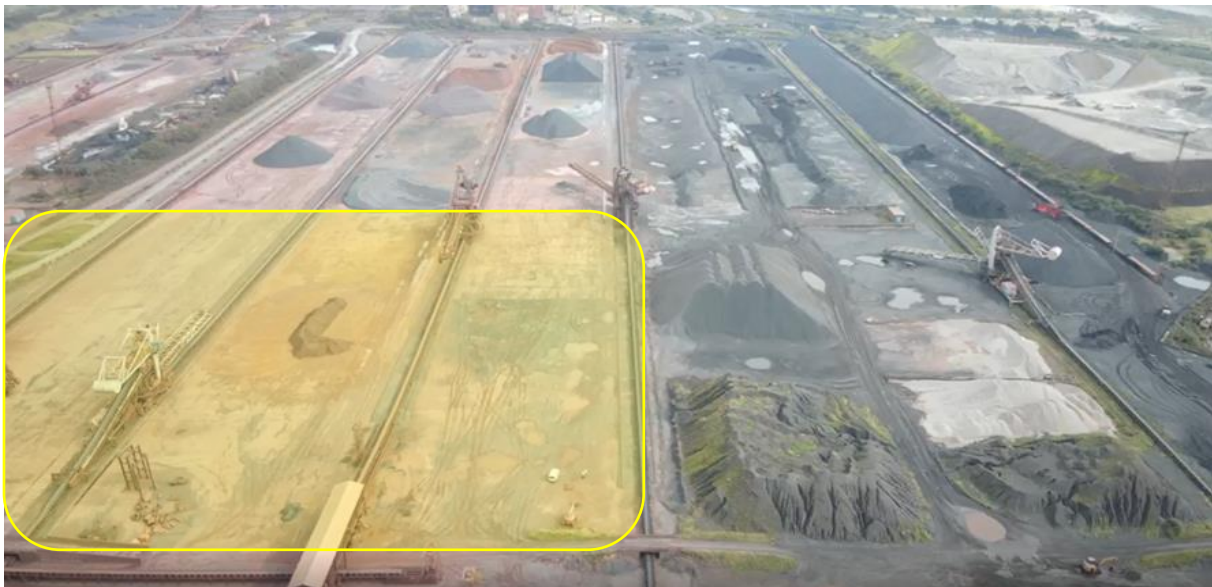
Fig 3: Lay down area (Marked in Yellow Box)
