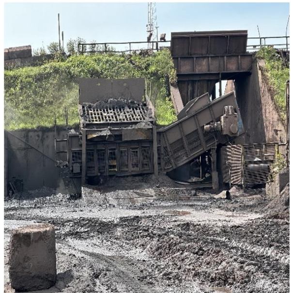
Fig.19 Screening and Unloading steel hopper
