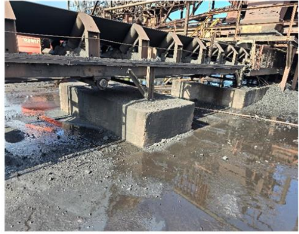
Fig. Combined footing at tail end of conv.804
