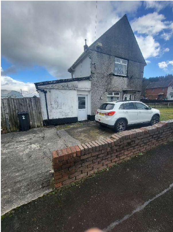
Front/side elevation view showing existing ground floor side extension and concrete parking area
