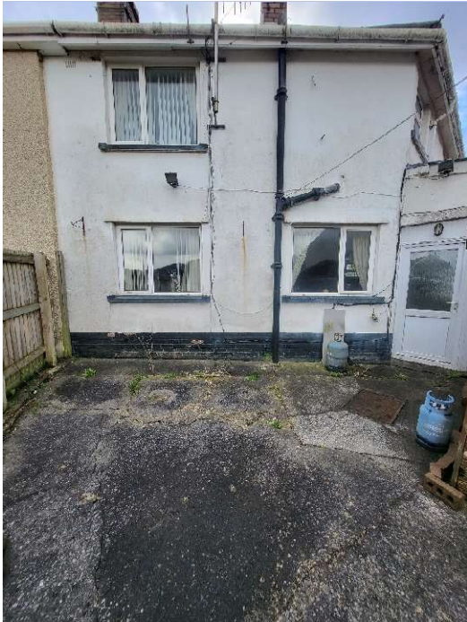
Rear elevation view of concrete yard area and timber fence boundary to neighbours
