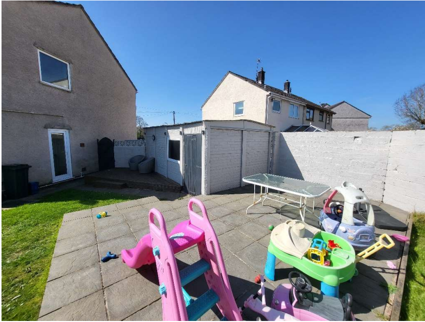
Side area of plot with existing garage and patio area. Blockwork boundary walls to the rear and side will remain untouched.
