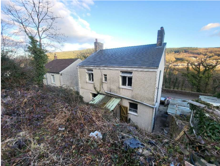
Rear elevation view of existing rear lean to outbuilding where new extension will be sited and area of new retaining wall. Side area with existing outbuildings can also be seen.
