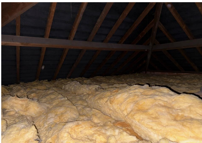
Figure 8: First floor roof void and bedrooms within the historic roof space
