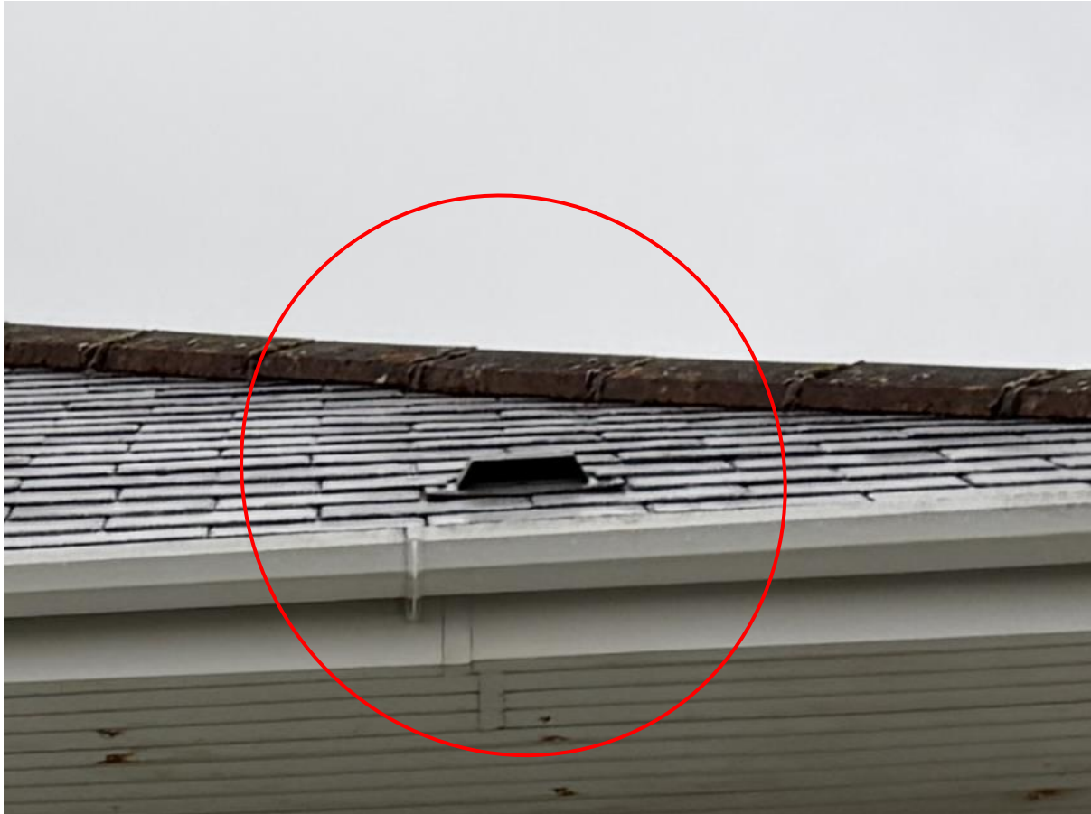
Figure 4: Vents with internal grill on the eastern and western aspect of the Roof Covering
