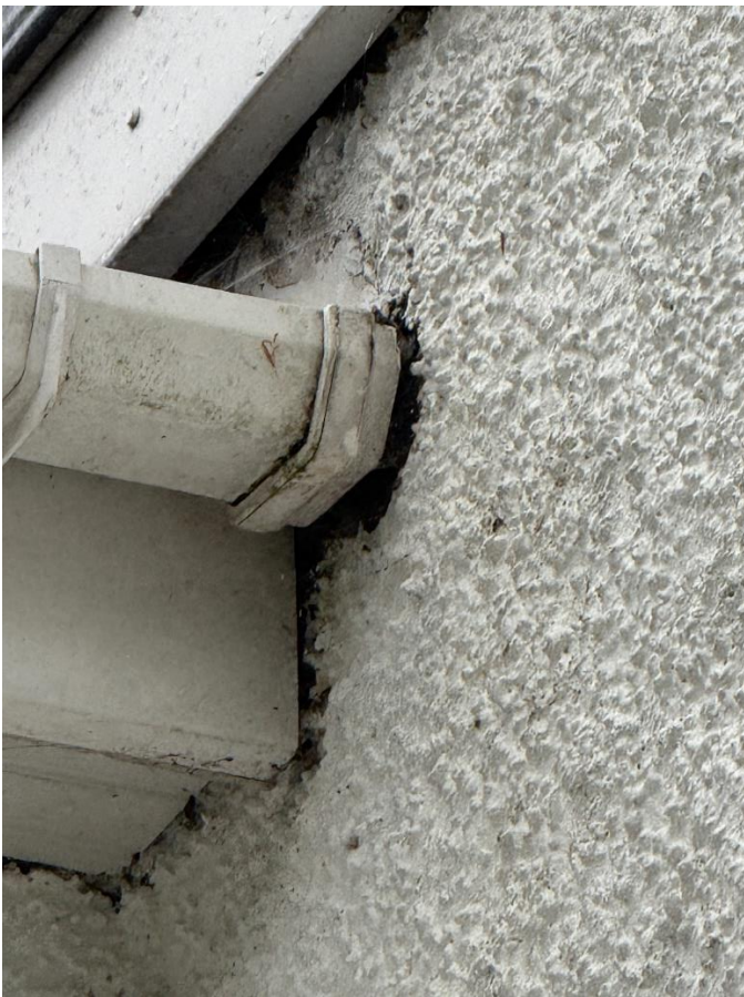
Figure 7: Checked PRF Gaps in soffits and fascia
