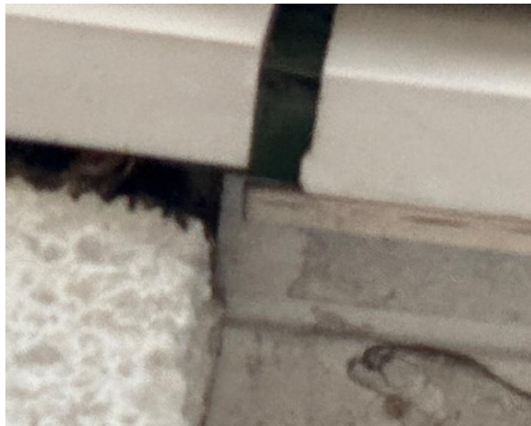
Figure 7: Checked PRF Gaps in soffits and fascia
