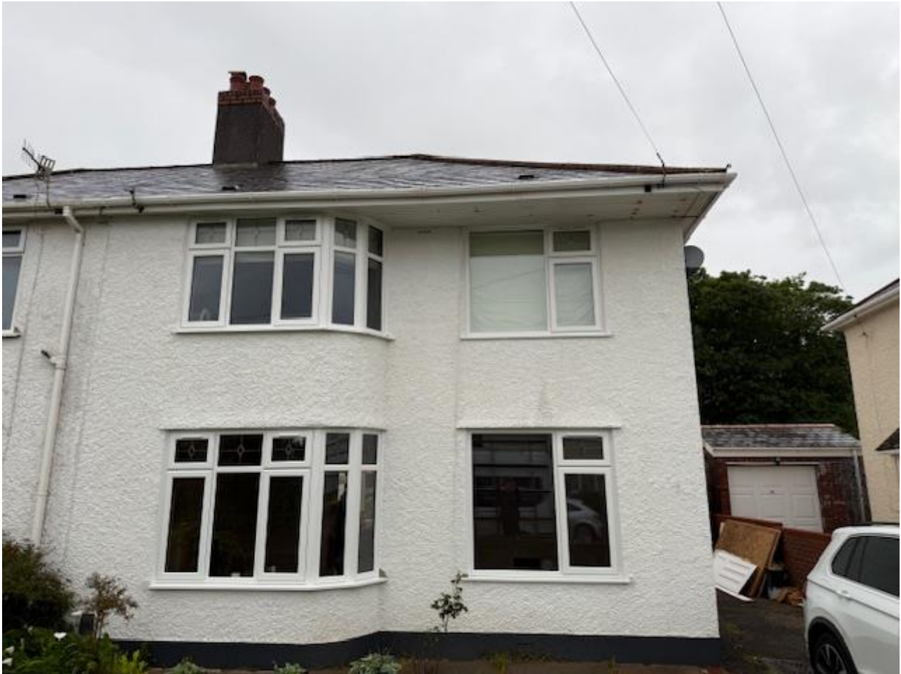
Figure 5: Roof Surfaces and Walls - front aspect (West aspect)
