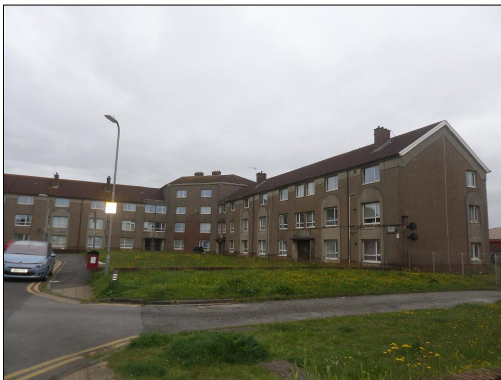
Photo 6: Coronation House complex (view looking north).
