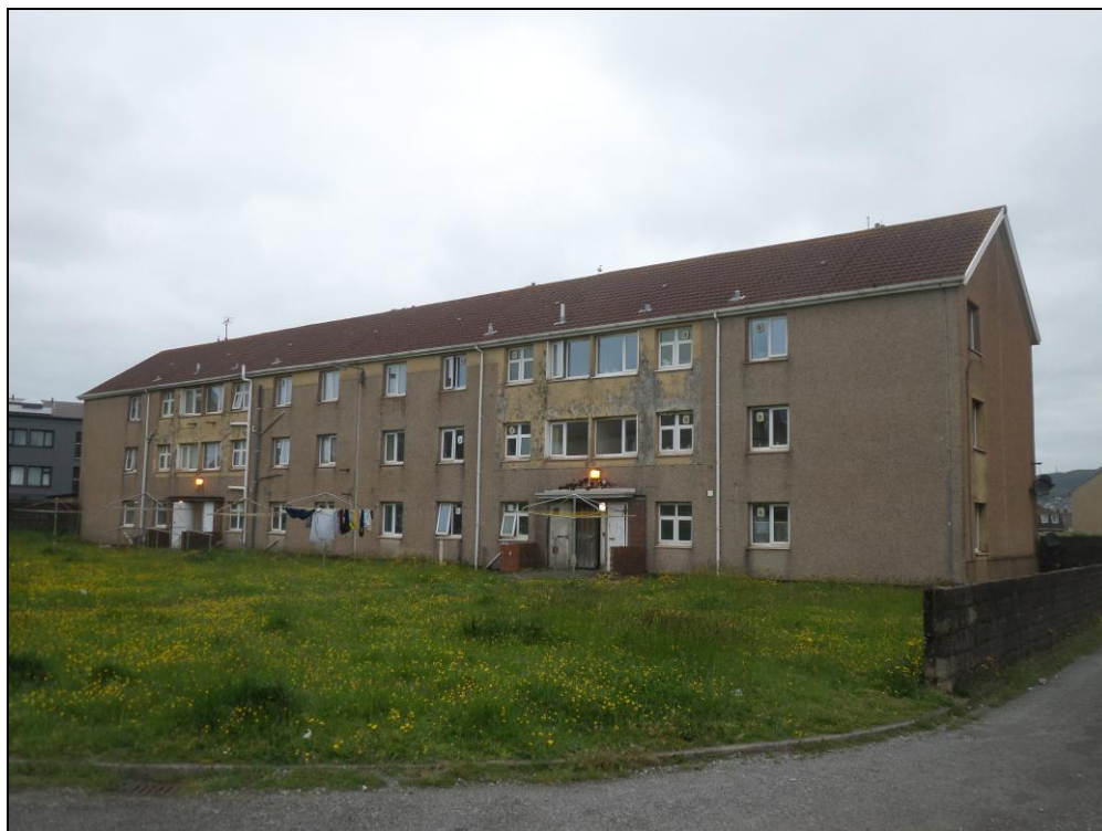
Photo 9: Cardigan House's southern elevation (view looking north).
