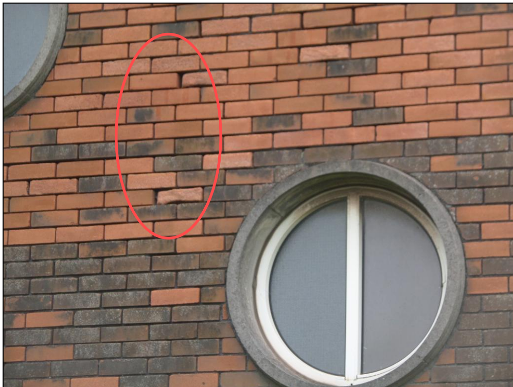
Photo 5: Missing pointing between red brick on stairwell (view looking south east).
