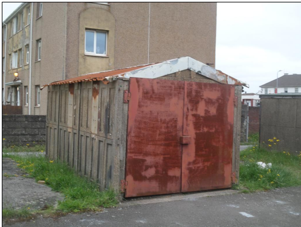
Photo 12: Detached garage located at rear of Cardigan House (view looking west).
