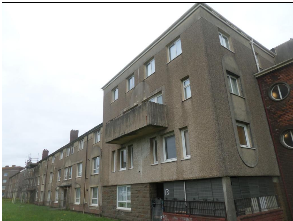
Photo 1: Southern extent of Carmarthen House (view looking north east).
