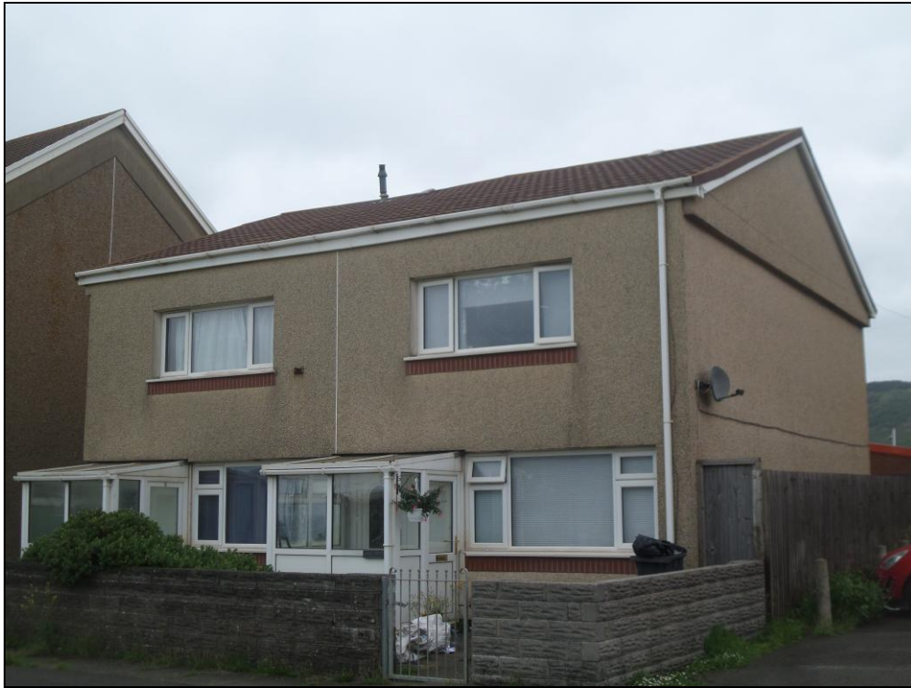
Photo 11: Southern elevation and eastern gable end of semi-detached properties (view looking north west).
