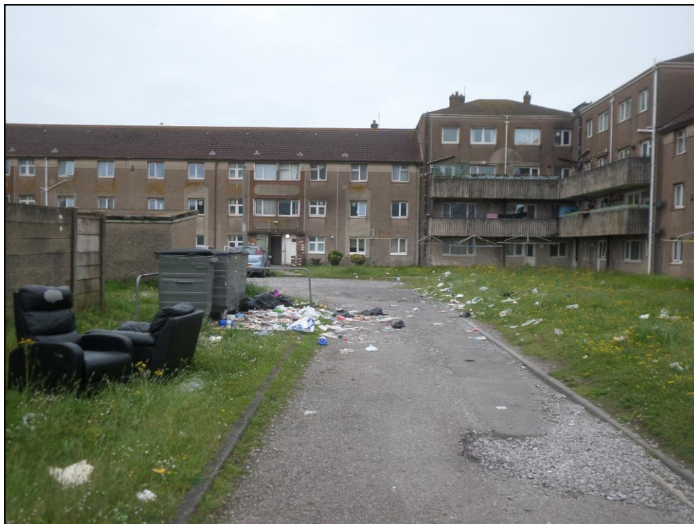
Photo 2: Rear of armarthen House (view looking south).
