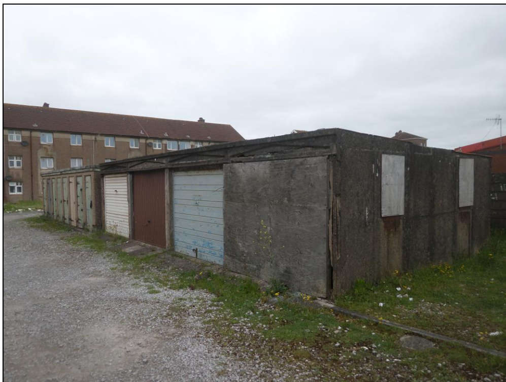
Photo 13: Row of garages and storage units at rear of Carmarthen House (View looking north west).
