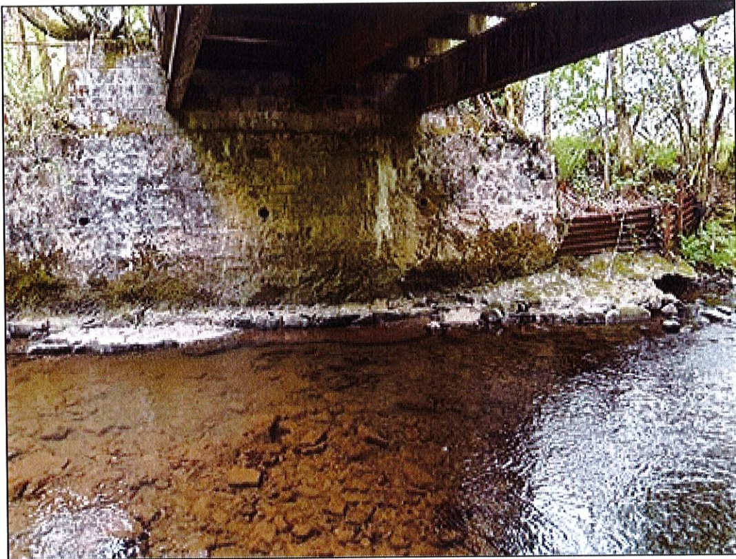
Photo Two The north abutment appears to have been built for a wider bridge. The abutment is on a sandstone ledge and there does not appear to be any undermining of the foundations.
