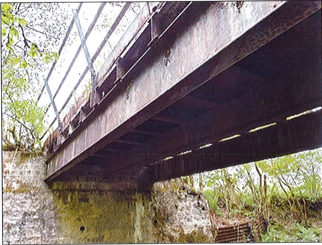
Photo One General view of the bridge looking north. The bridge construction can be seen with a concrete deck on steel plate shuttering supported on cross beams at 800mm centres which are in turn carried by main beams spanning from abutment to abutment.
