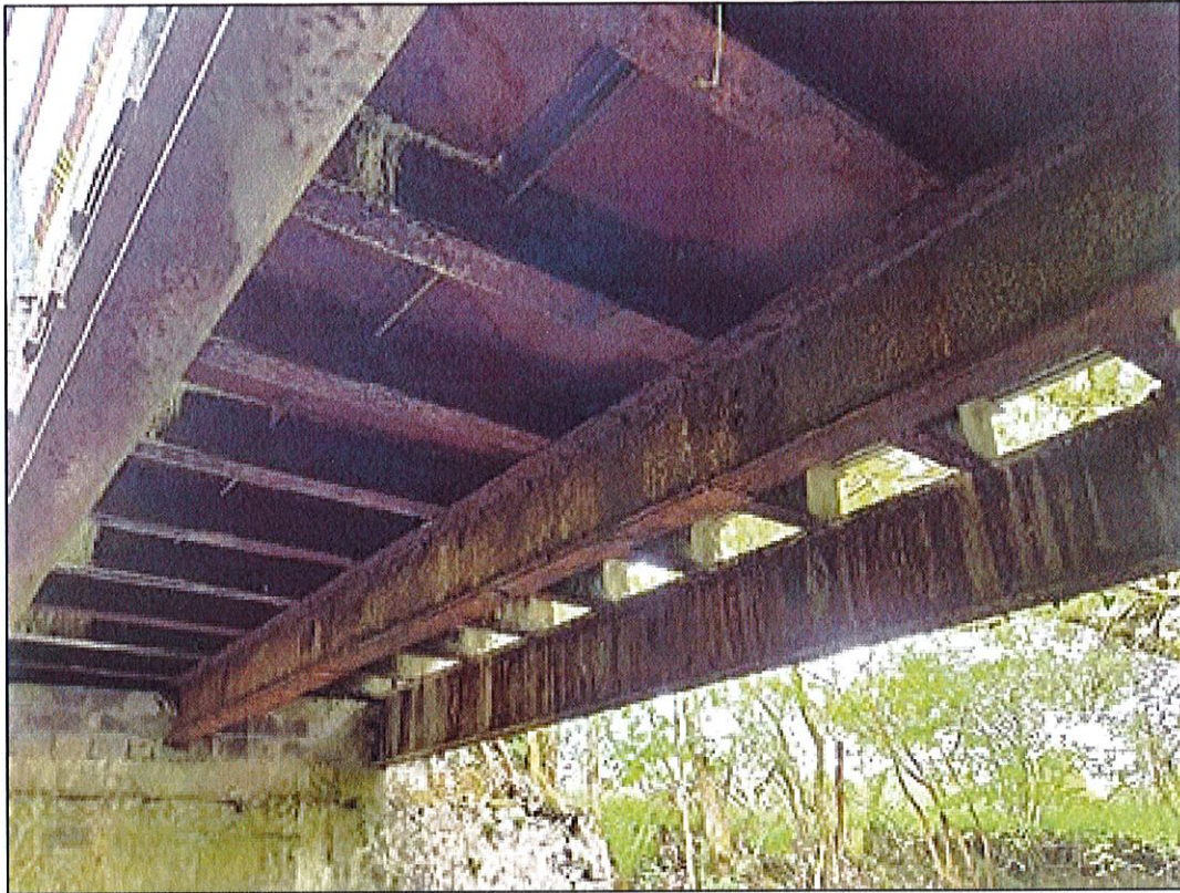
Photo Three The underside of the bridge showing the three main support beams.
