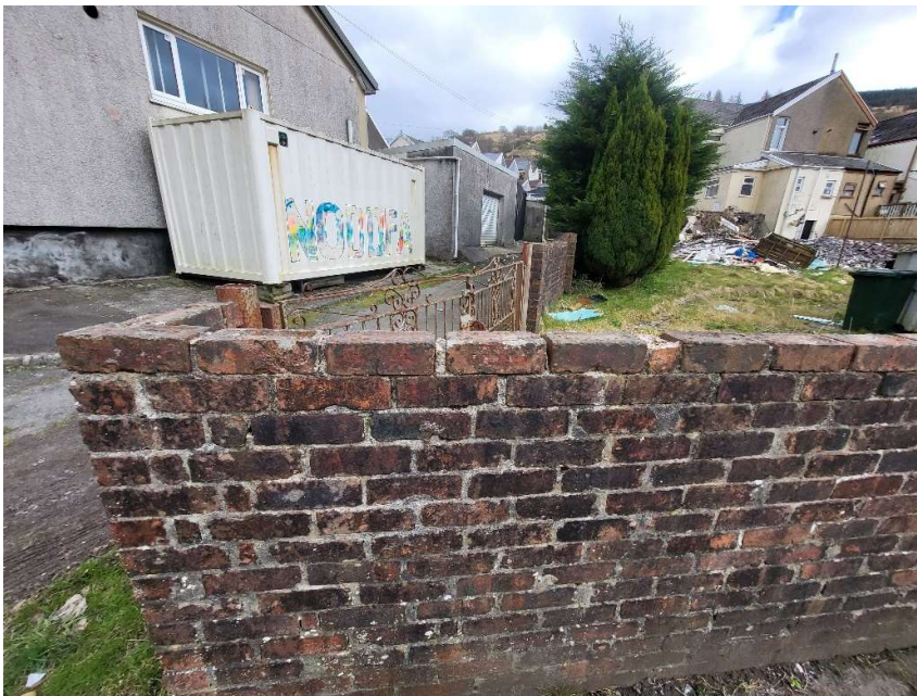
Rear and side boundaries onto lane. Brickwork walls will remain in place. Existing gates to driveway also in view
