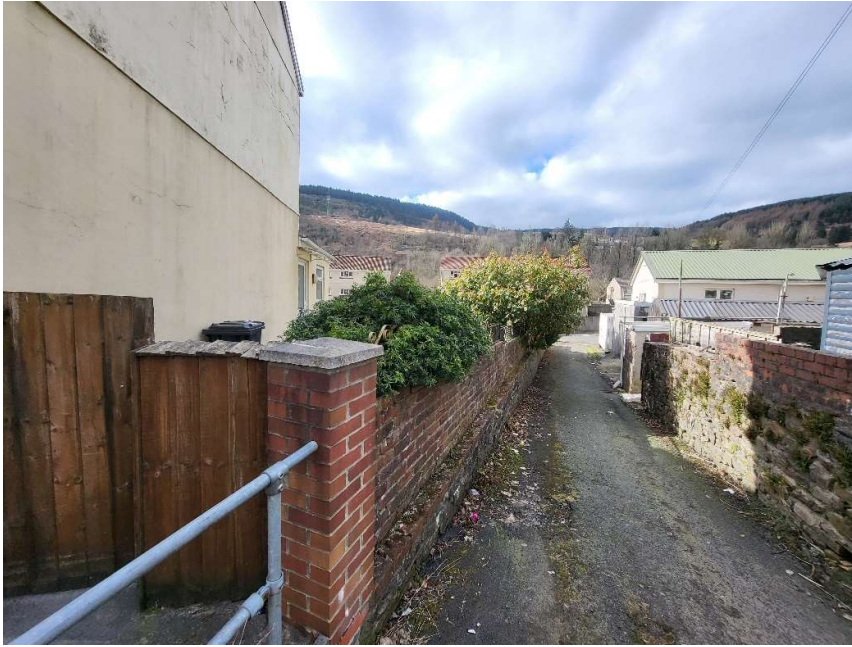
Side boundary to lane. This is where the extension will sit on an existing patio area
