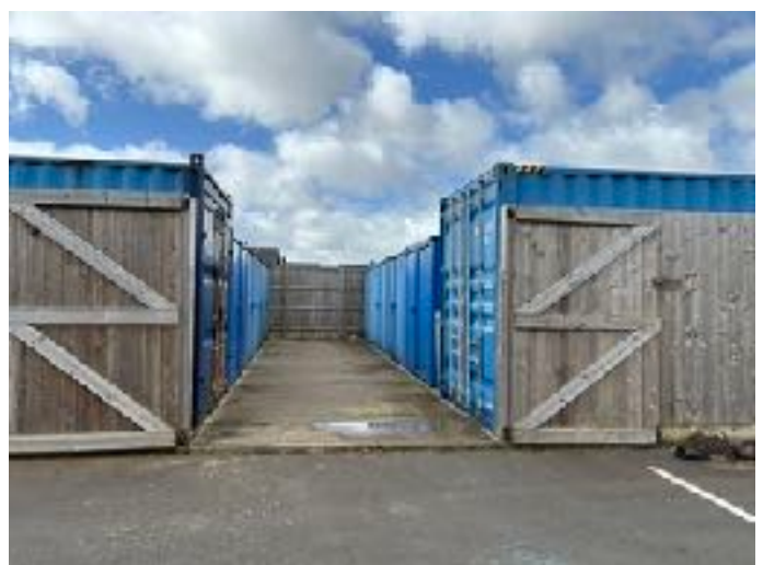
Storage containers to the west of nursery building
